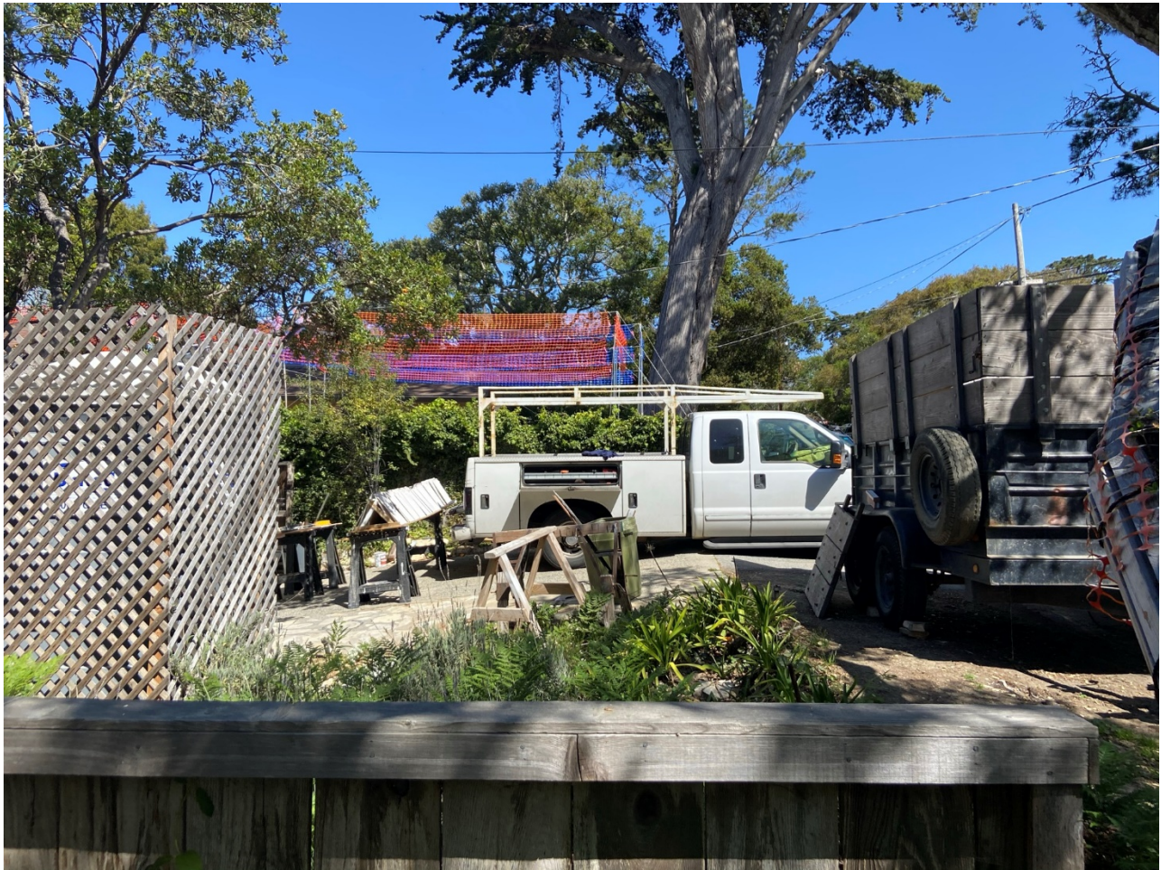
Figure 1. Garage story poles. Project proposal shown in orange with Applicant's proposed alternative shown in blue.
