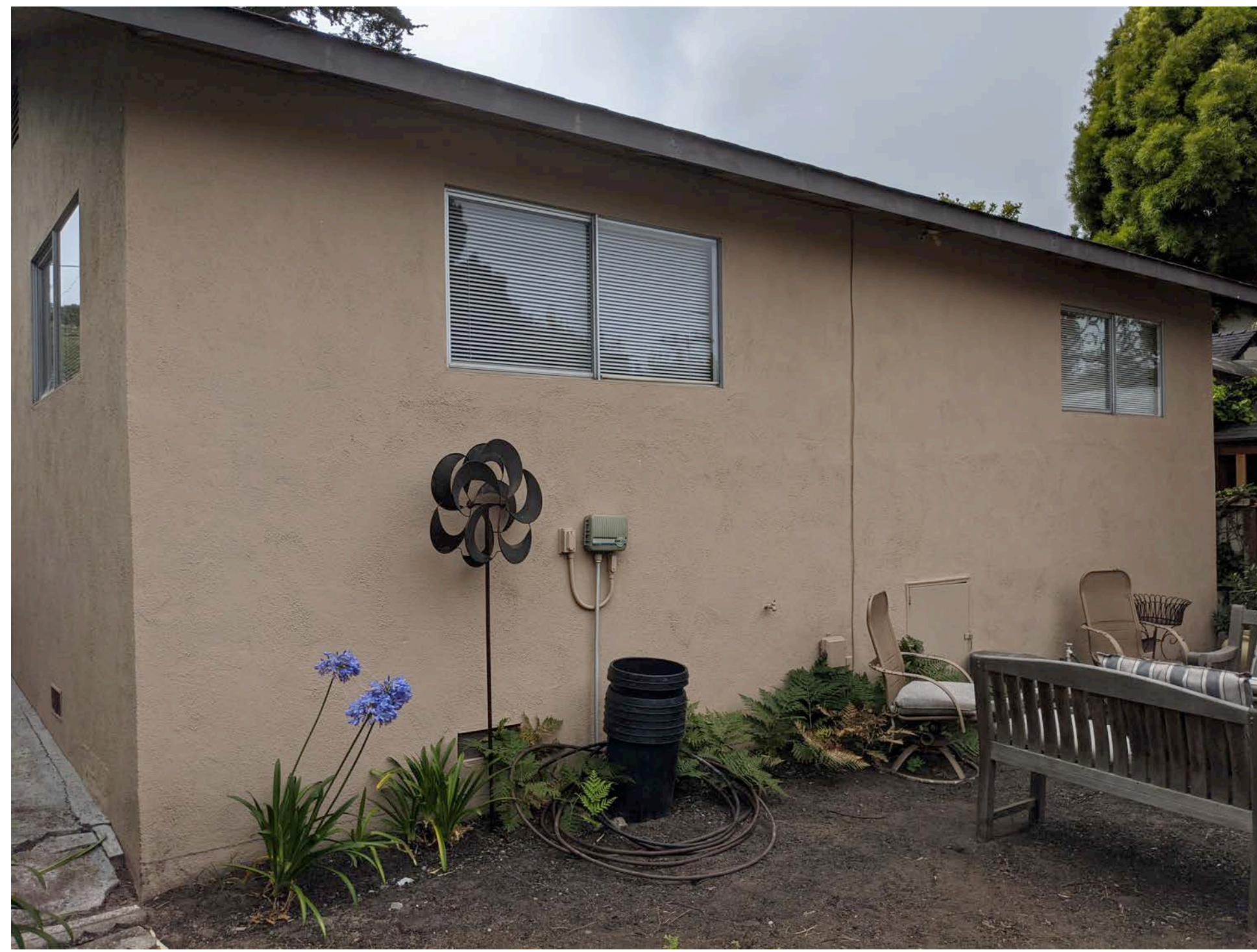
Existing Residence From Rear Yard
