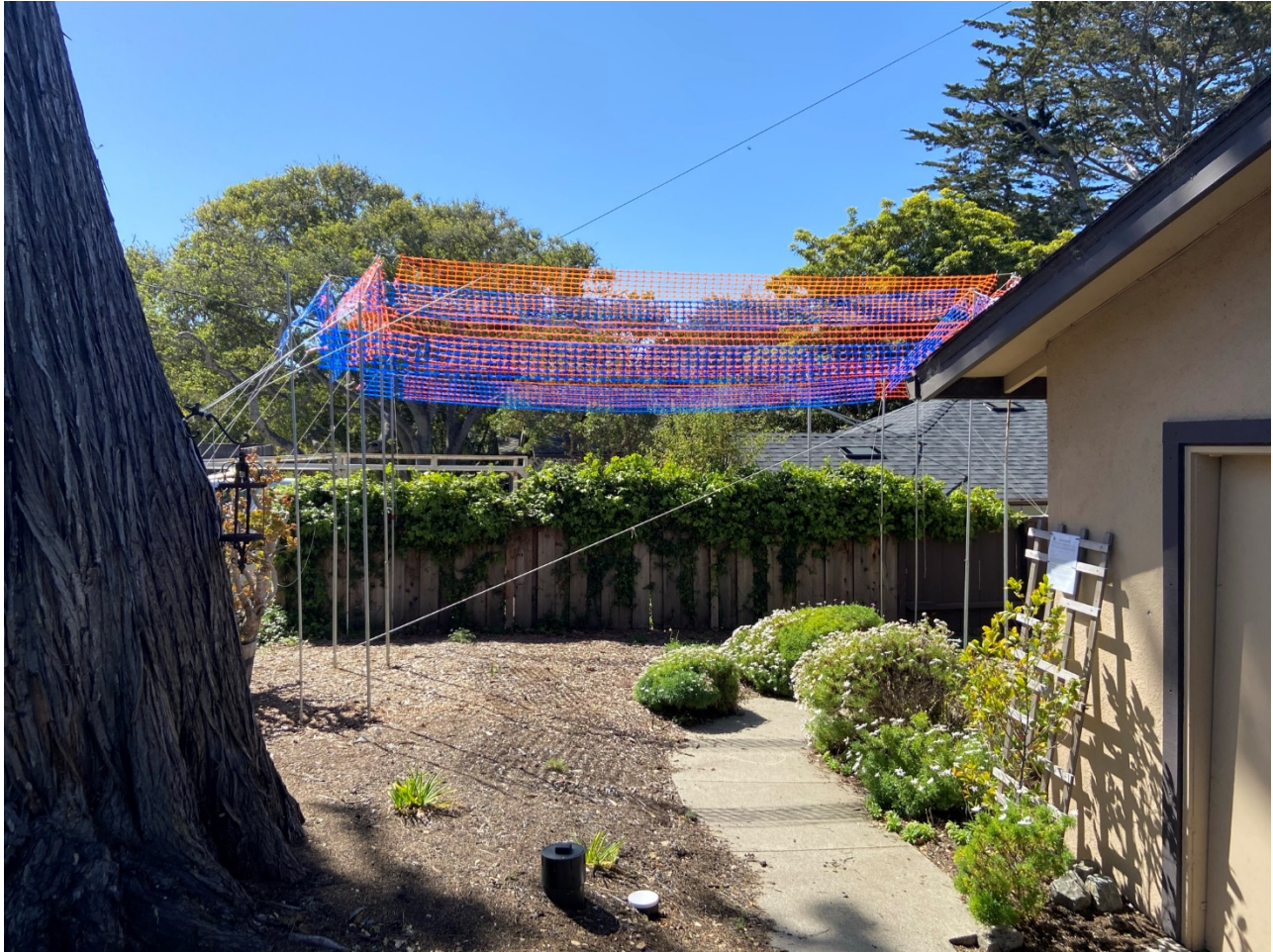
Figure 3. Garage story poles. Project proposal shown in orange with Applicant's proposed alternative shown in blue.
