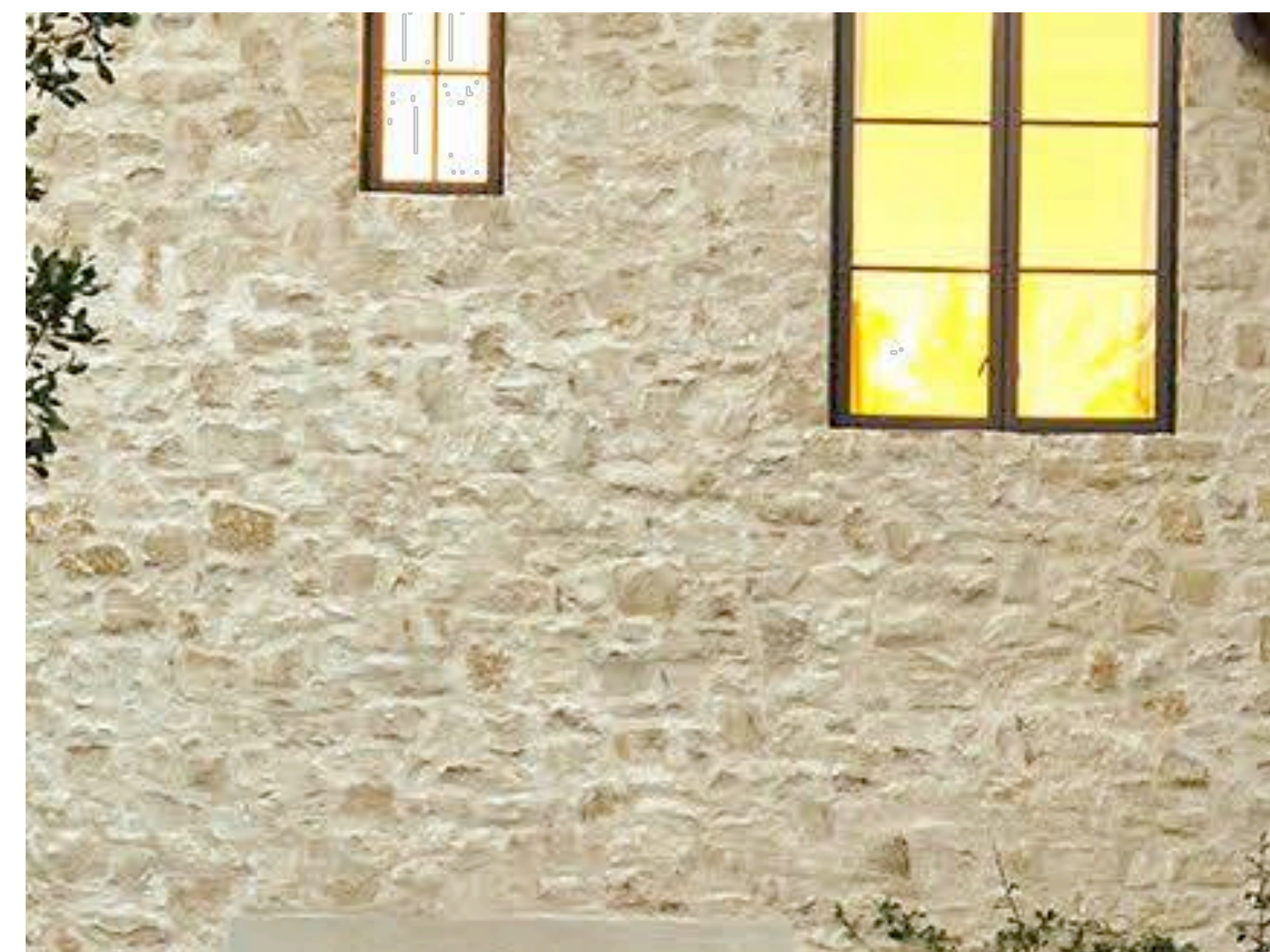
Exterior Walls & Site Walls Over-Grouted Natural Limestone Veneer Fond-du-Lac Rustic or Equal
