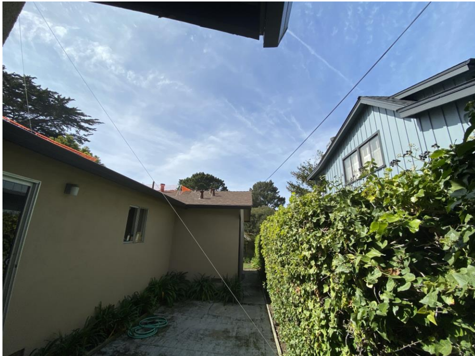
Figure 3. Roof Deck at Far Ridge with Adjacent Neighbor's Residence (north).
