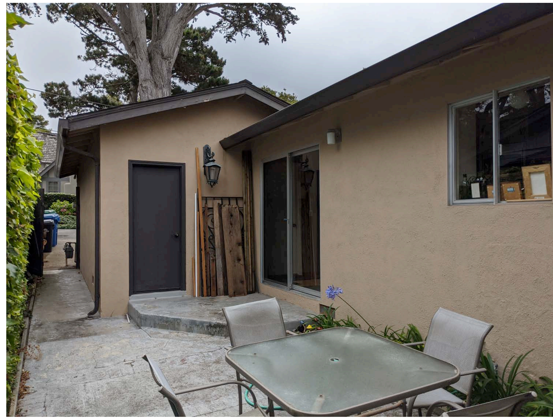
Existing Residence From North Side Yard
