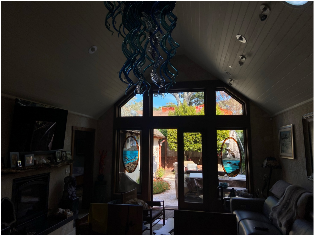
Figure 4. Northwest corner of roof deck (area immediately left of trees) visible from neighbor's living room/kitchen.
