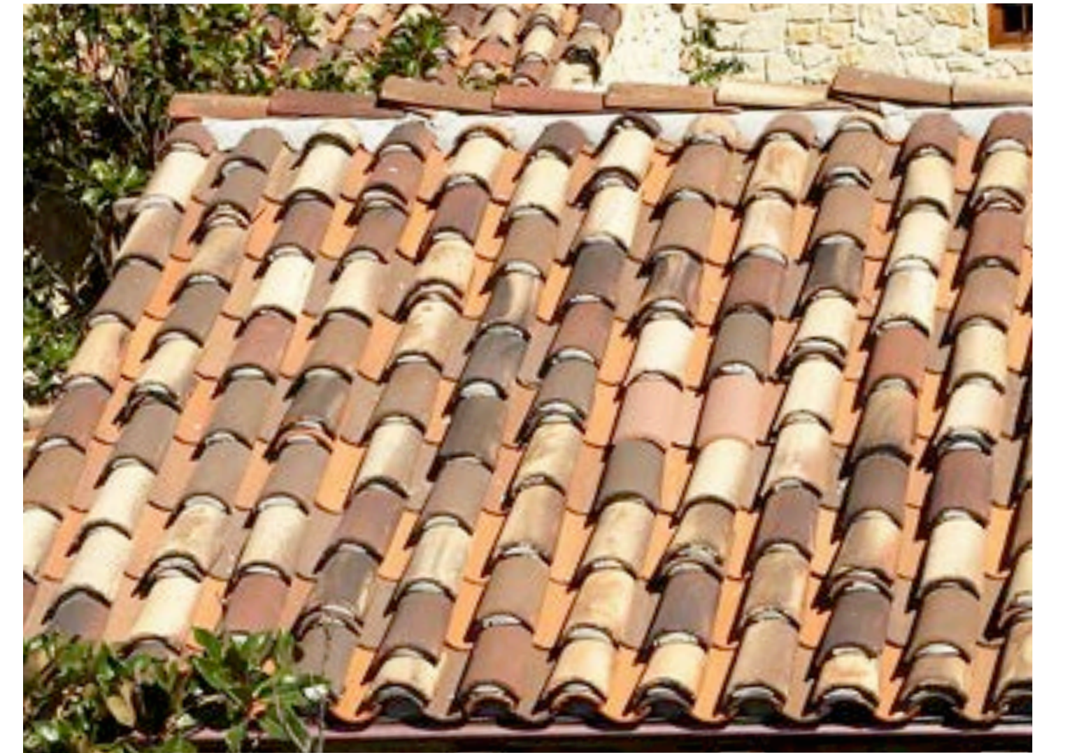
Roofing Two-Piece Mission Clay Tile Redland Clay Tile
