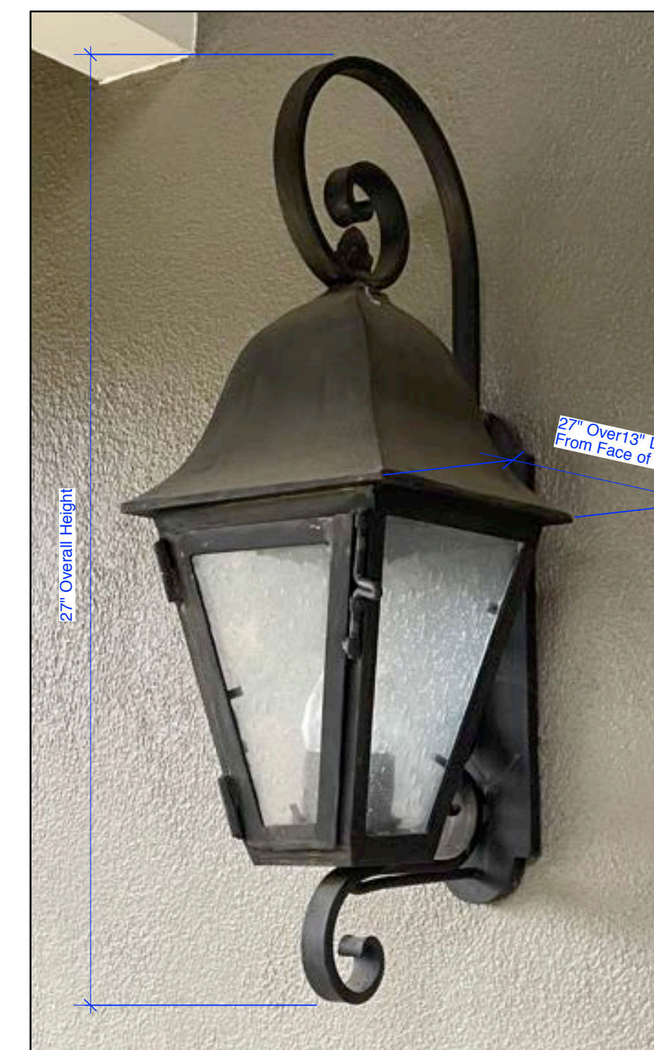
Existing Wall Mounted Exterior Lantern 13" x 27" (Overall Height) Existing Black Painted Finish
