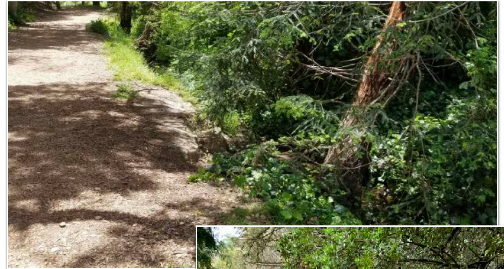
Area of Stream Stability Projects #4 & #5
