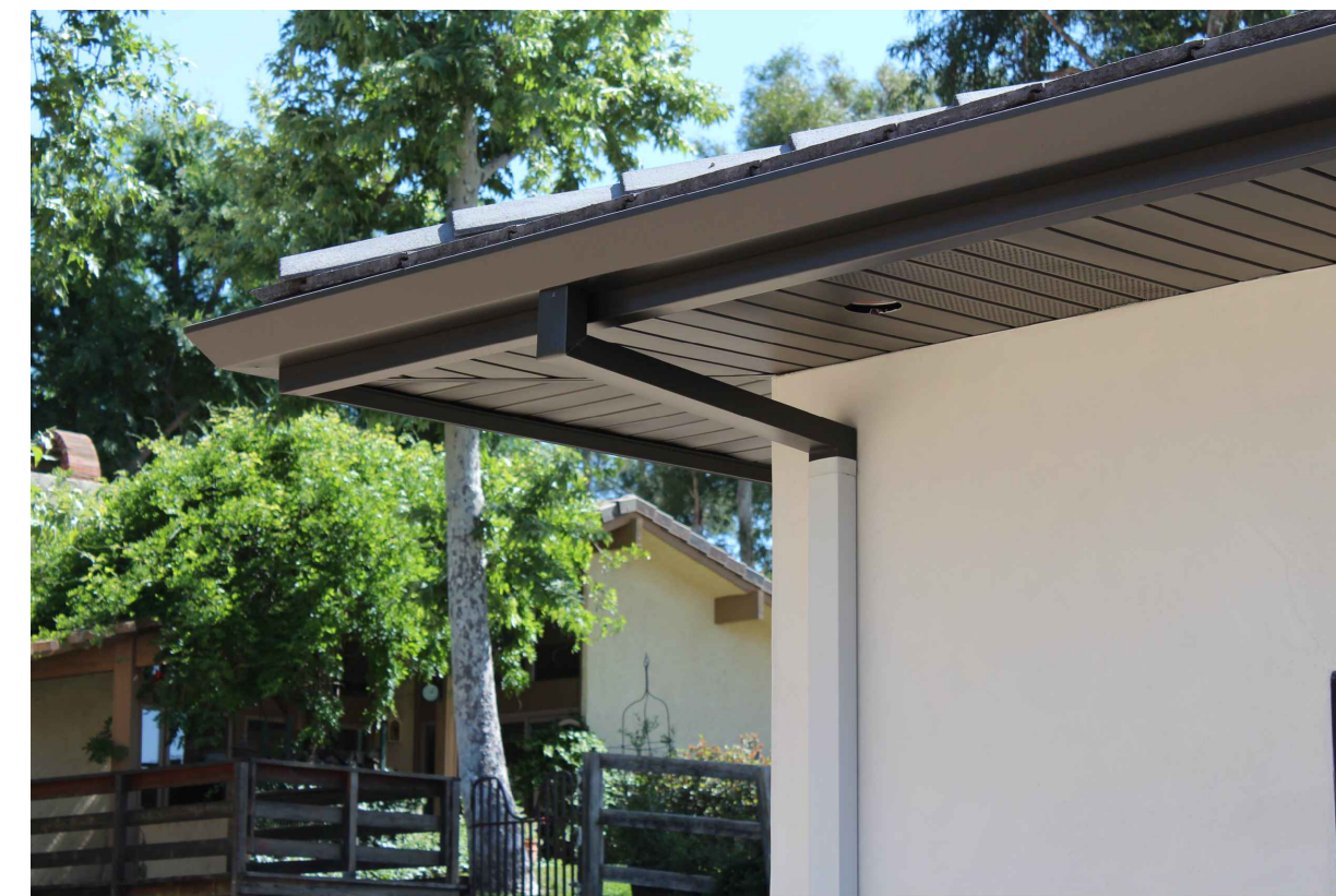
BLACK METAL FASCIA GUTTERS W/ PAINTED DOWNSPOUTS
