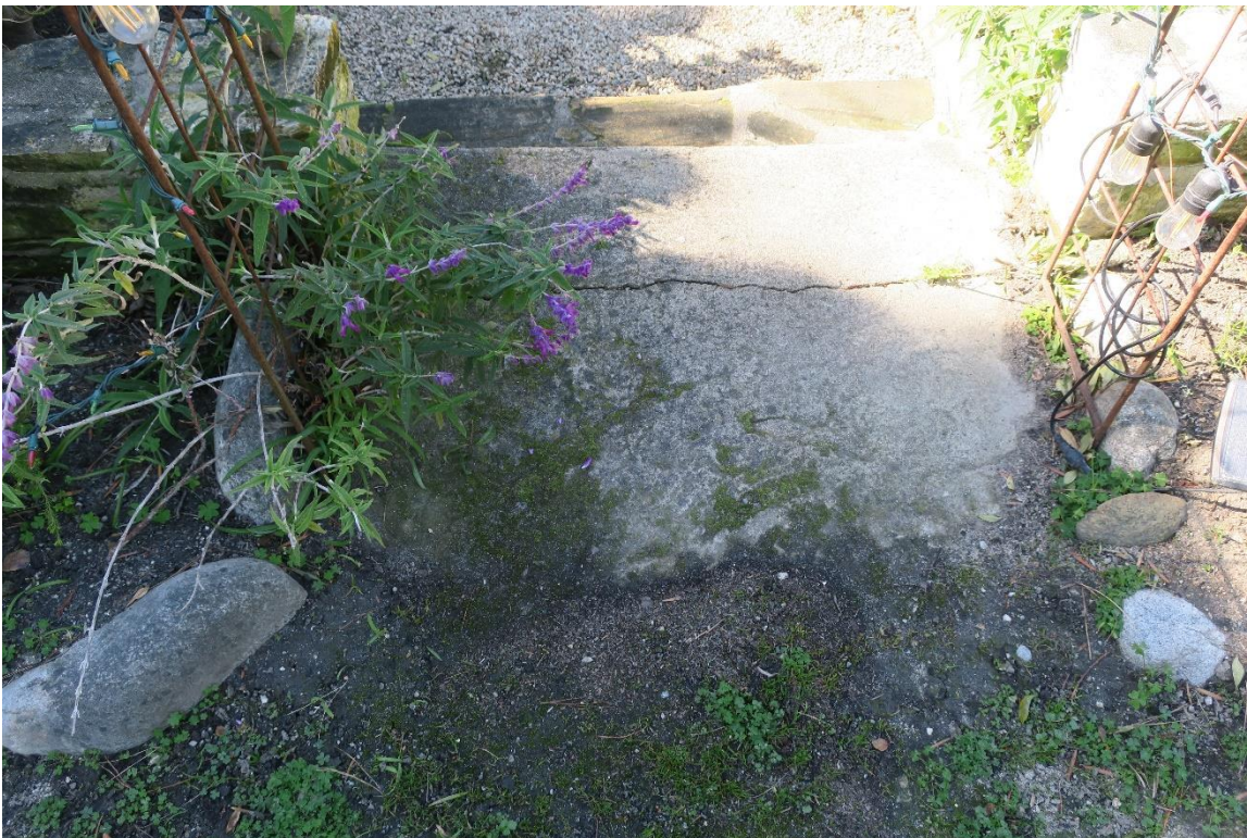
Step landing fronting Santa Rita Street.
