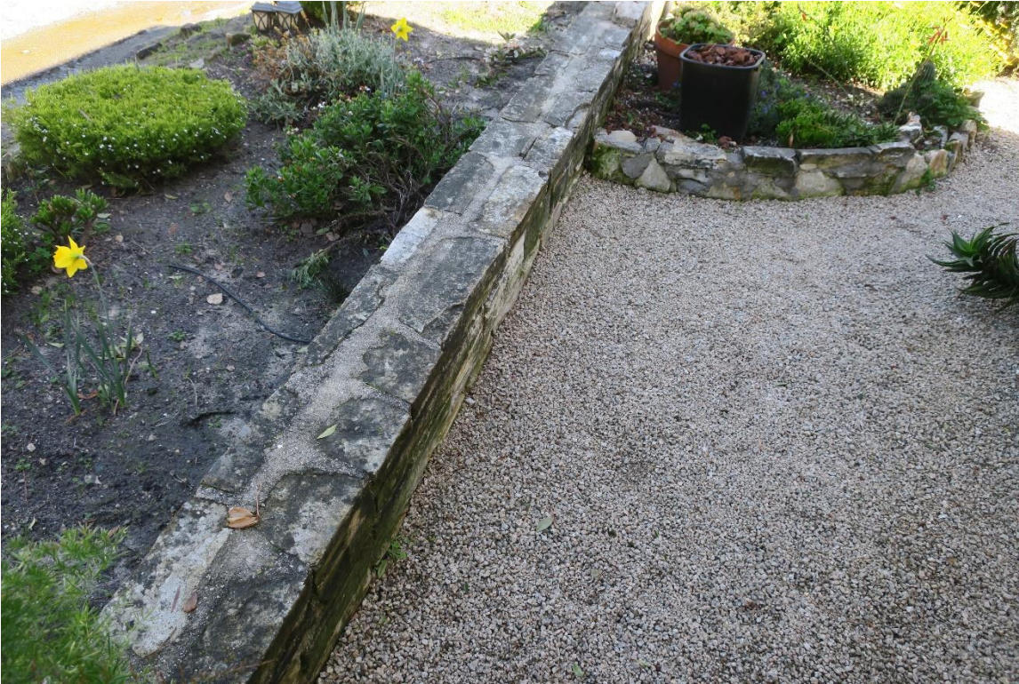
Retaining/garden wall just outside the north property line.
