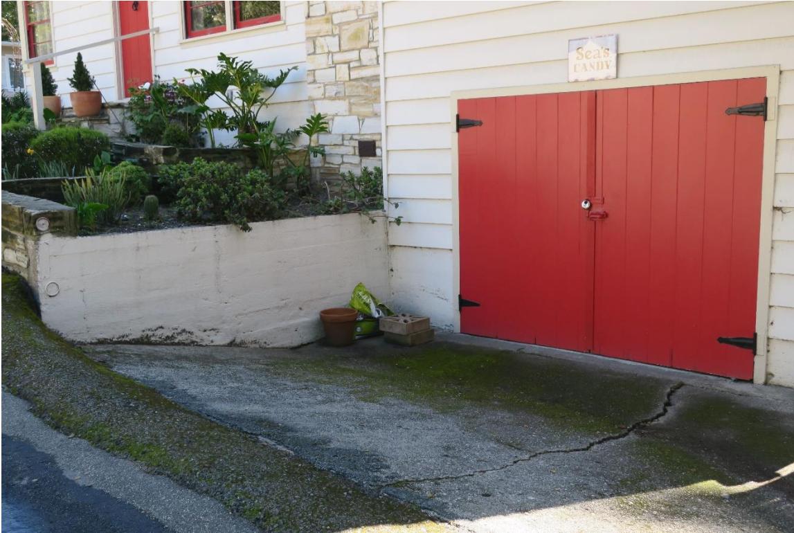
Planter-style retaining wall east of and adjacent to the driveway fronting 1 st Avenue. View southeast.
