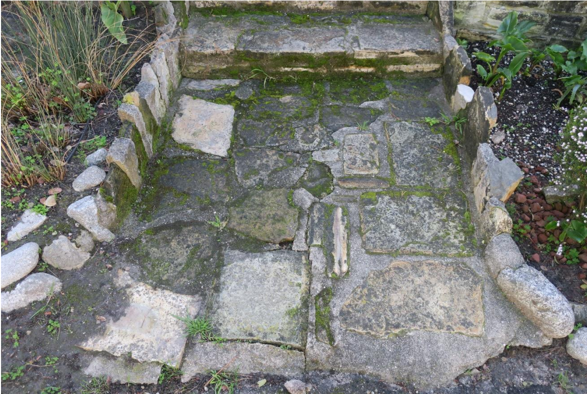
Step landing fronting 1 st Avenue.
