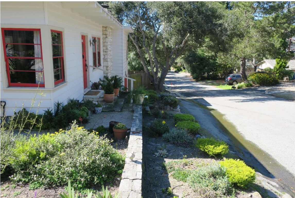
Retaining/garden wall just outside the north property line. View west.
