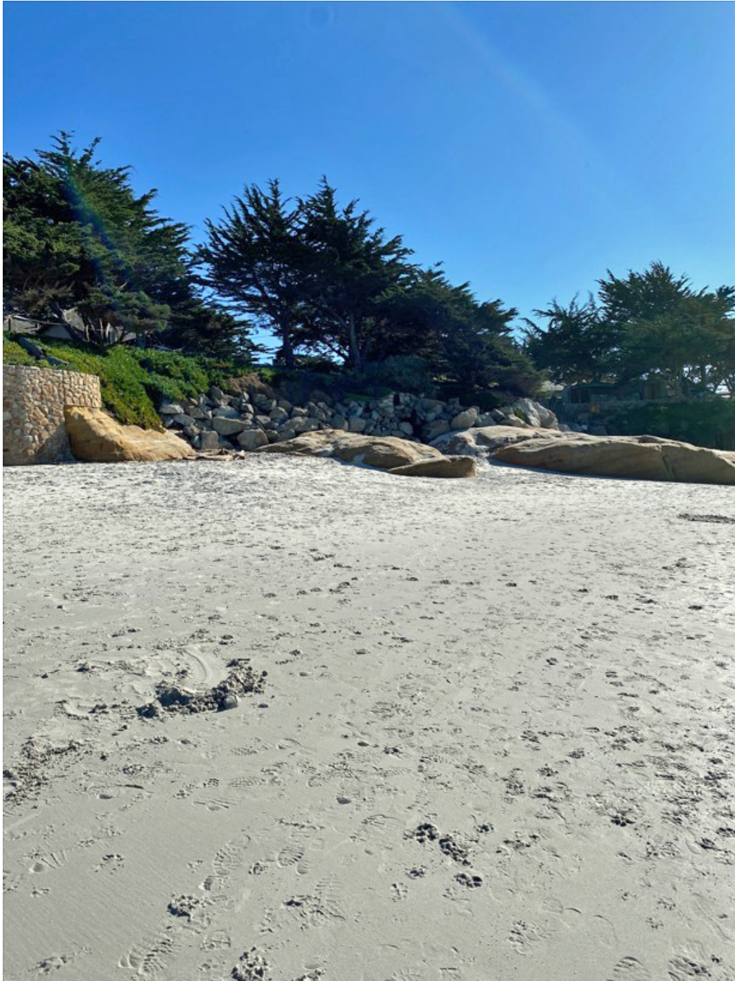
Photograph 16: Showing Revetment R1 on January 30, 2023
