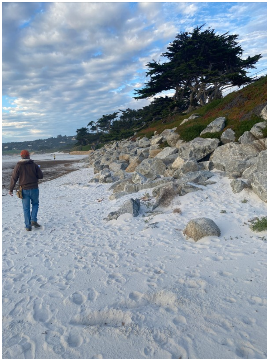
Photograph 50: Most of Revetment R3 is in Good Condition on December 22, 2022
