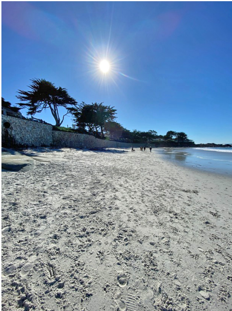
Photograph 8: Showing Seawall S2 on January 30, 2023
