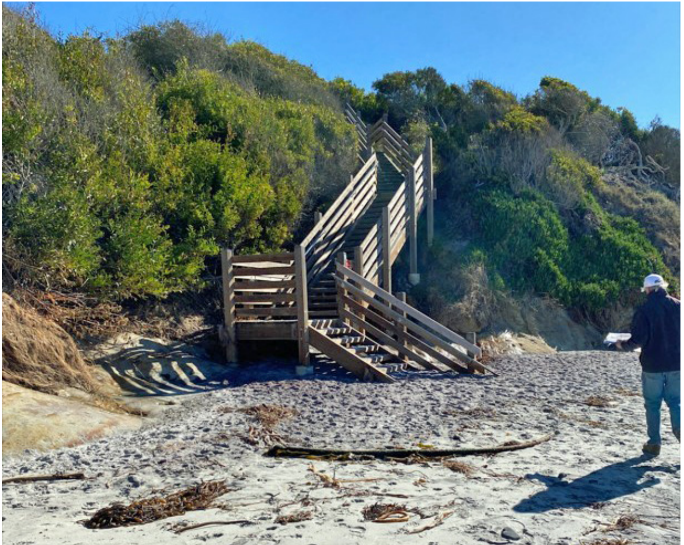
Photograph 96: Stairway ST11 on January 30, 2023
