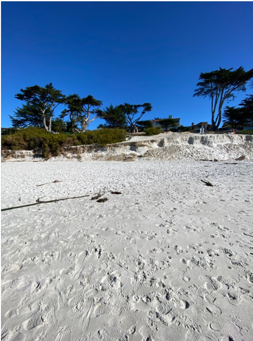
Photograph 85: Location of North Area of Revetment R5 on January 30, 2023
