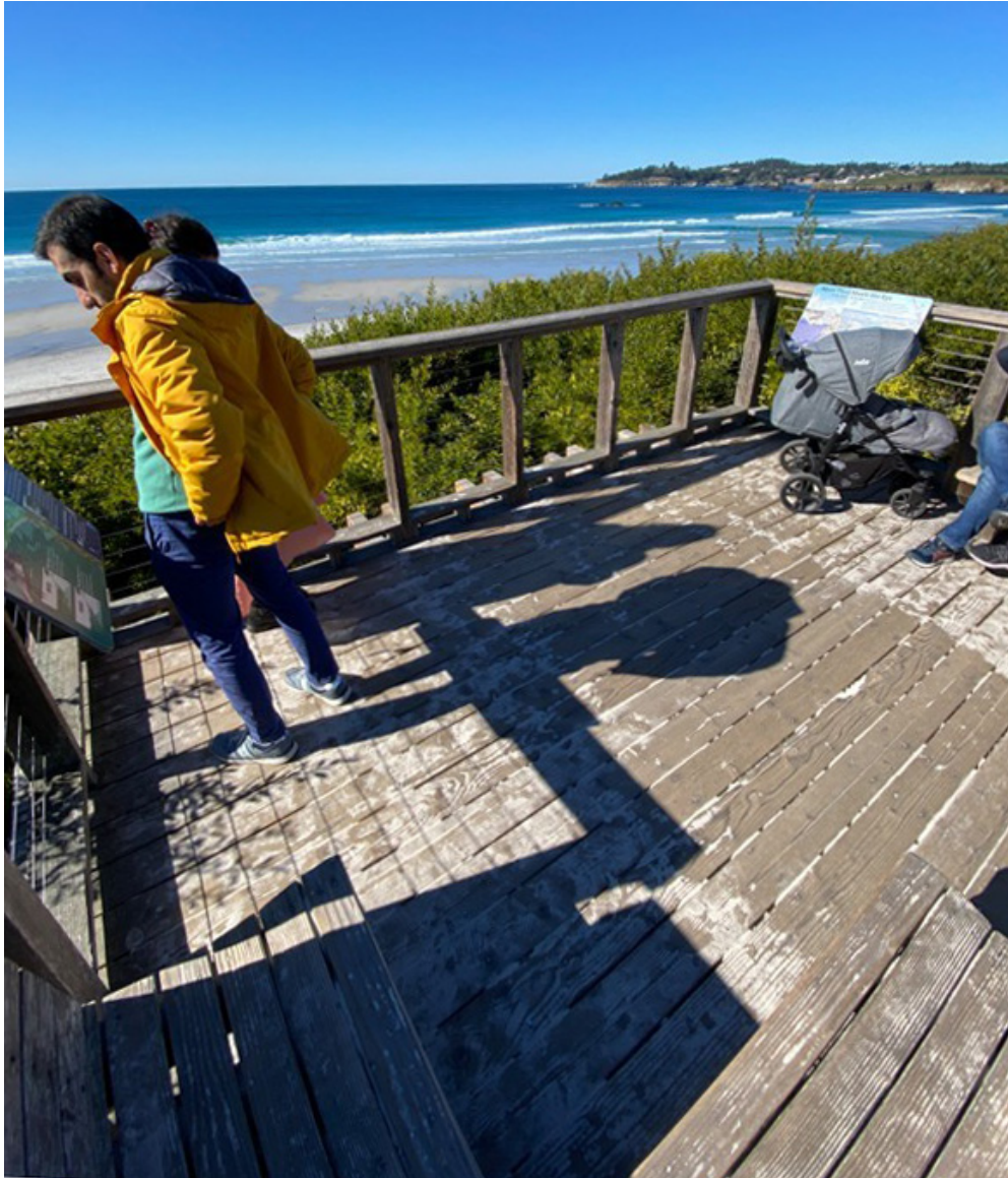
Photograph 90: Stairway ST10 Overlook Platform on January 30, 2023
