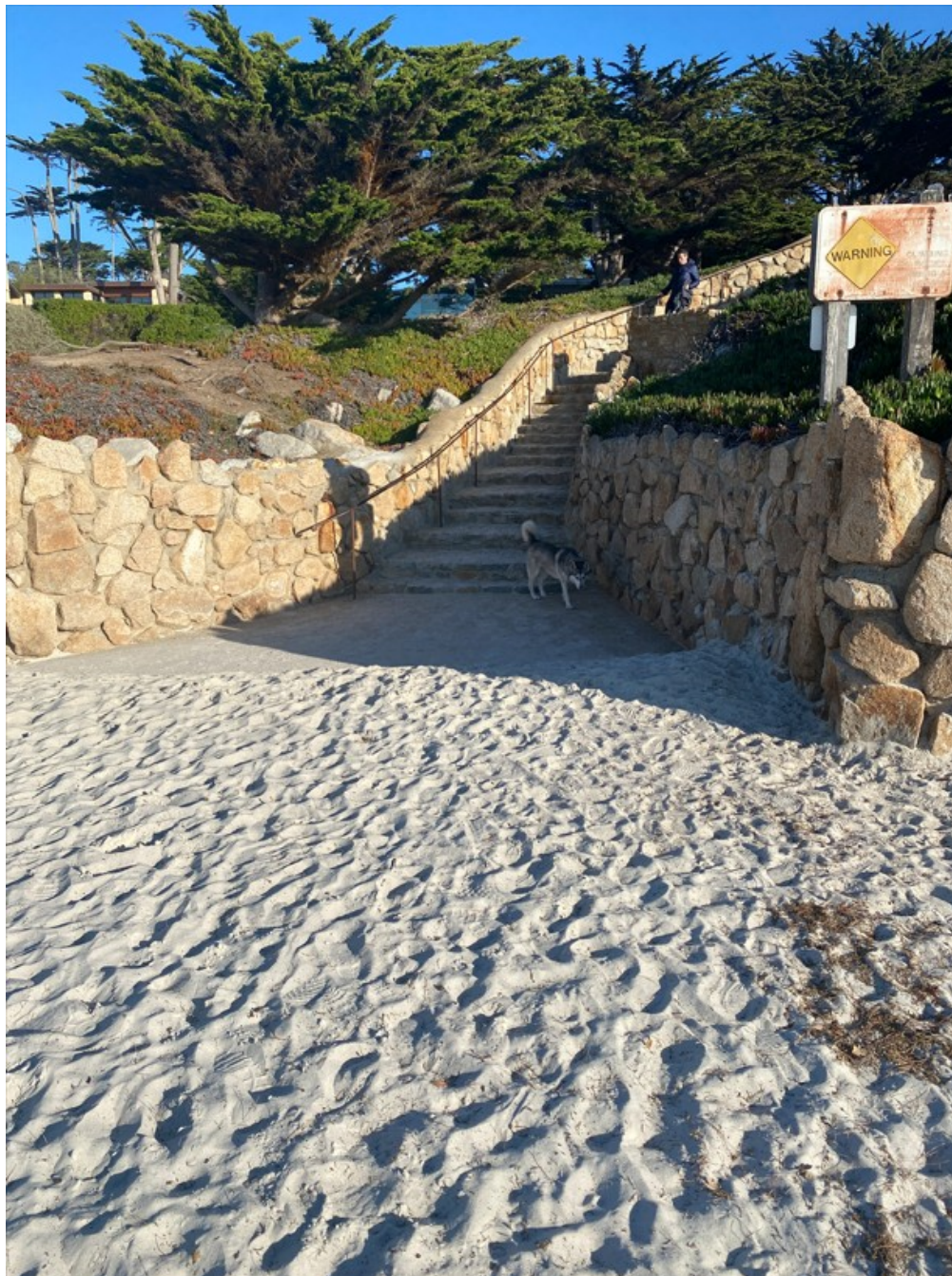
Photograph 27: Public Access Stairway ST3 on December 22, 2022
