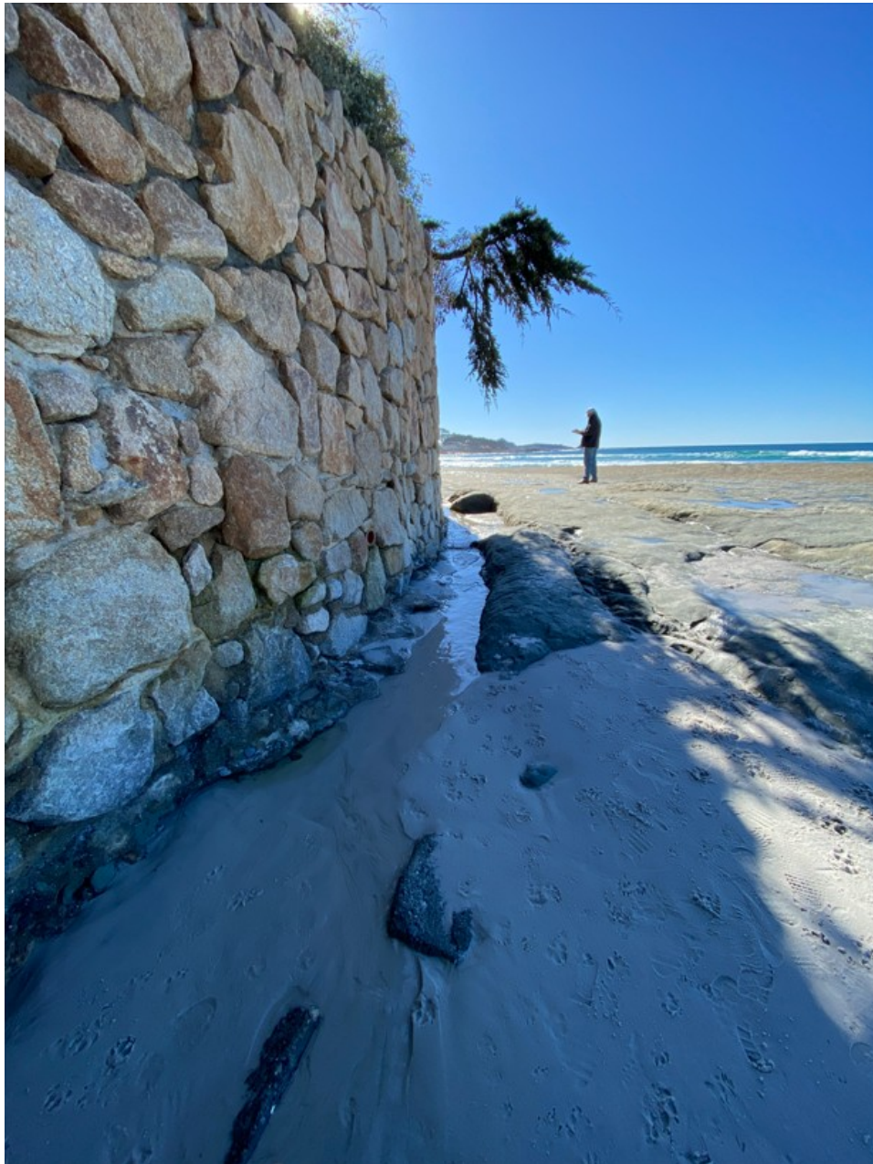
Photograph 70: Seawall S7 Foundation on January 30, 2023
