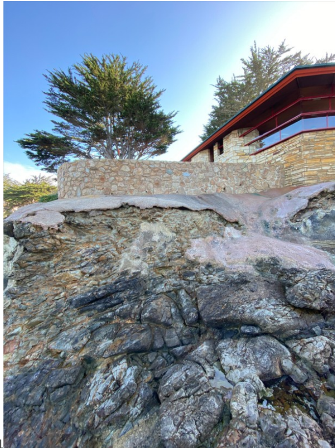
Photograph 1: Privately Owned Seawall S1 on December 22, 2022
