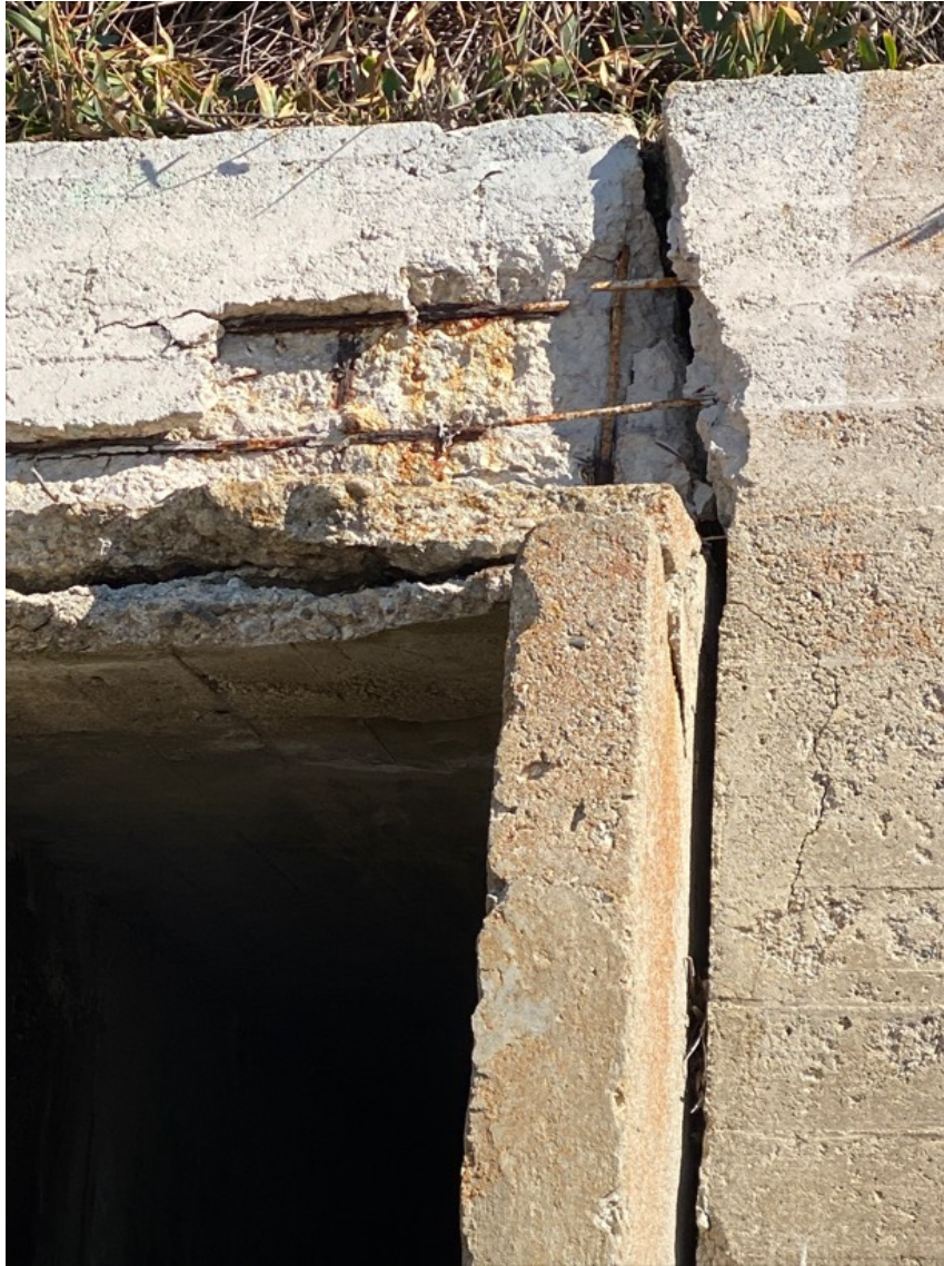
Photograph 95: Seawall S10 on January 30, 2023
