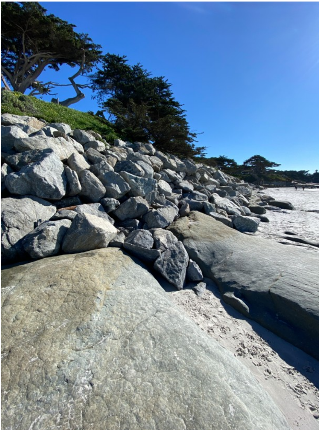
Photograph 53: Profile View of Revetment R3 on January 30, 2023
