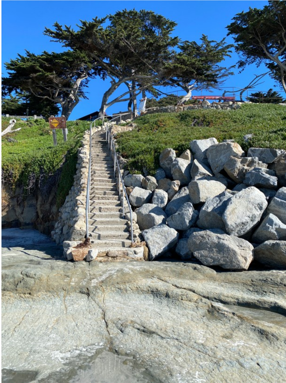
Photograph 57: Showing Stairway ST5 on January 30, 2023
