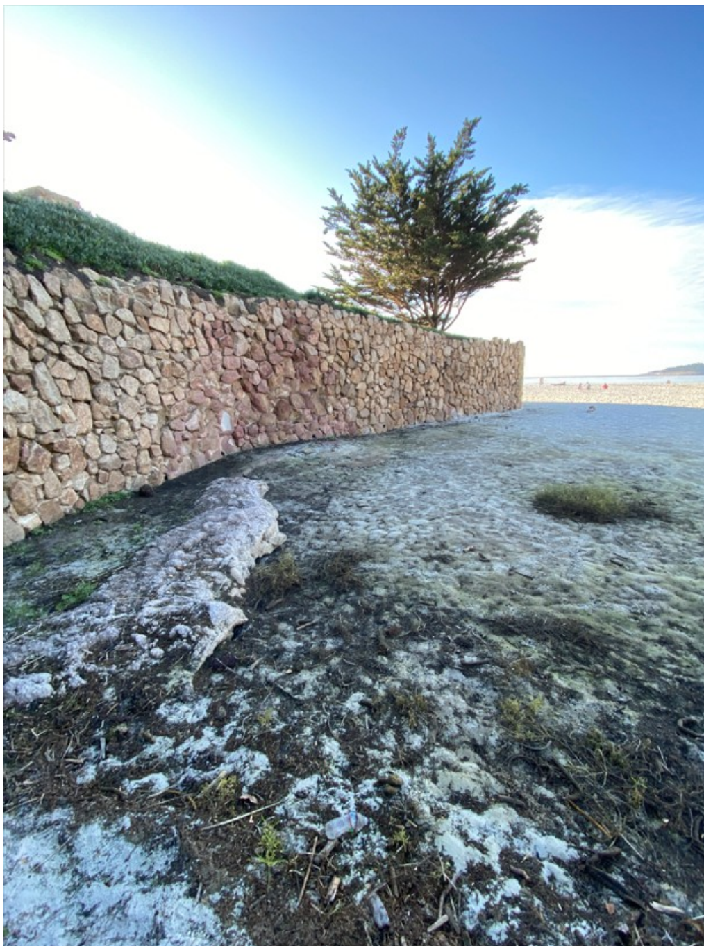
Photograph 22: Southern End of Seawall S3 on December 22, 2022
