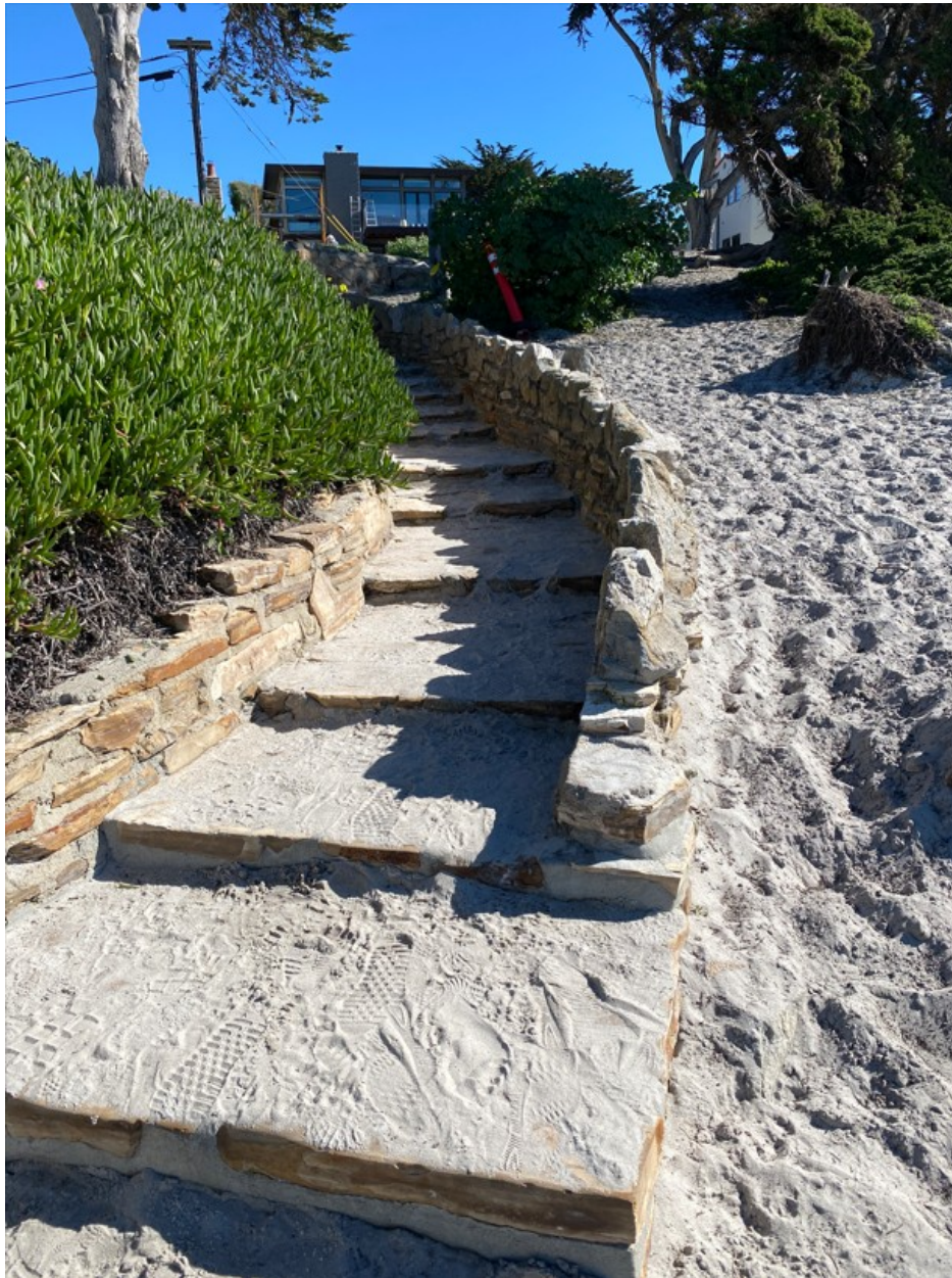
Photograph 86: Stairway ST9 on January 30, 2023
