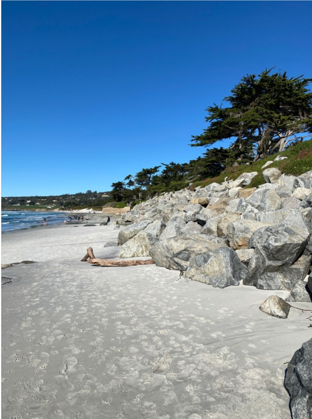
Photograph 52: Showing Revetment R3 Looking North on January 30, 2023
