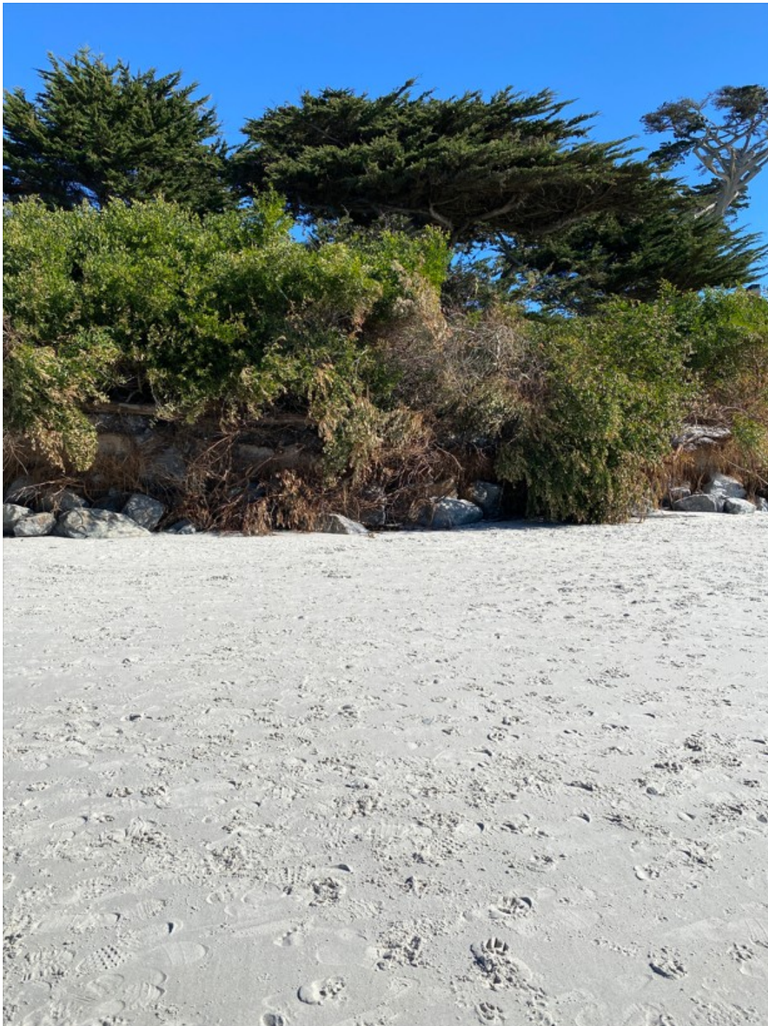
Photograph 83: Showing Additional Revetment R5 Rip-rap on January 30, 2023
