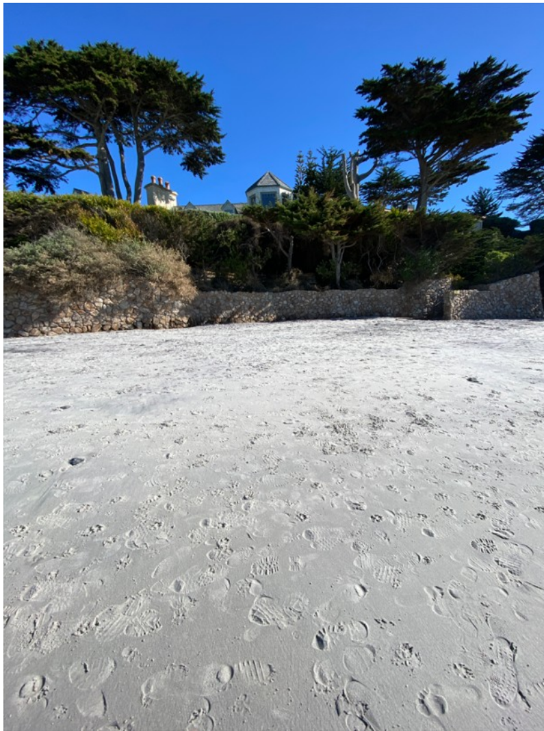
Photograph 97: South Portion of Privately Owned Seawall S11 on January 30, 2023
