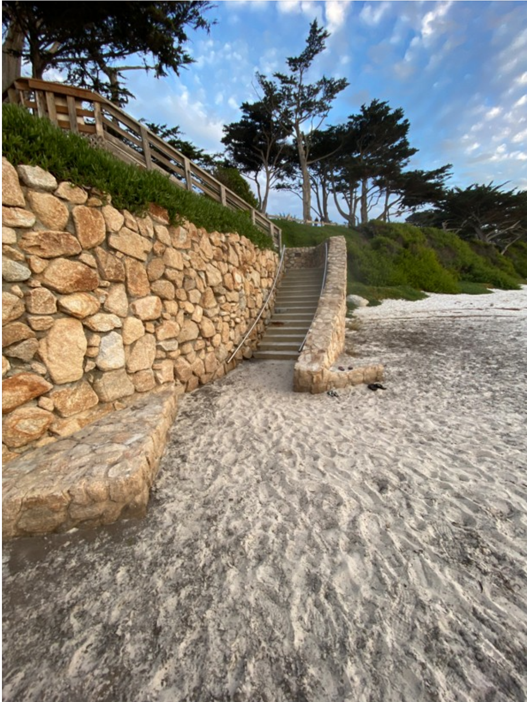
Photograph 64: Showing Stairway ST6 on December 22, 2022
