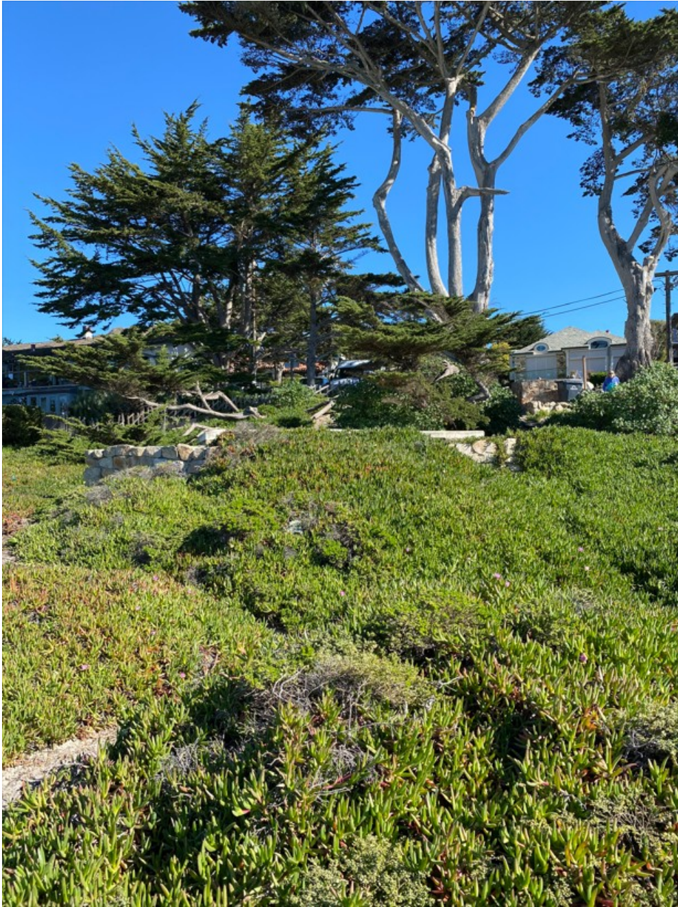
Photograph 88: Seawall S8 on January 30, 2023
