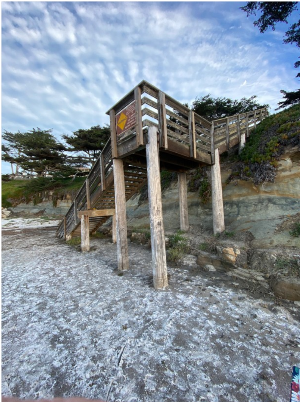
Photograph 38: Showing Public Access Stairway ST4 on December 22, 2022
