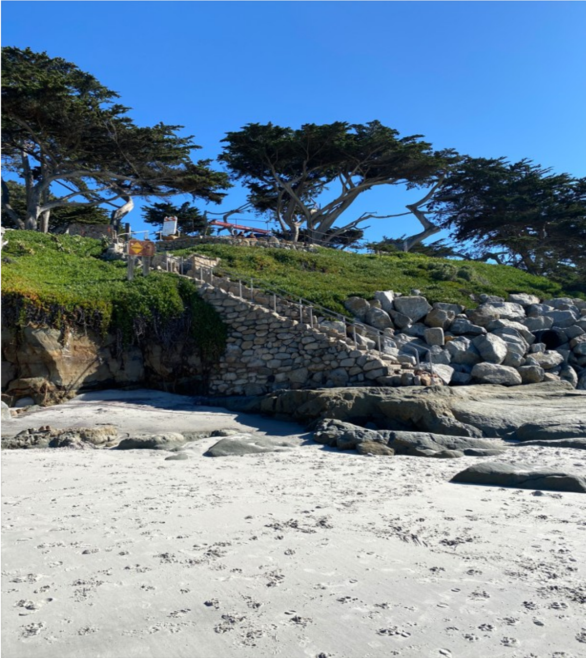
Photograph 56: Showing Stairway ST5 on January 30, 2023
