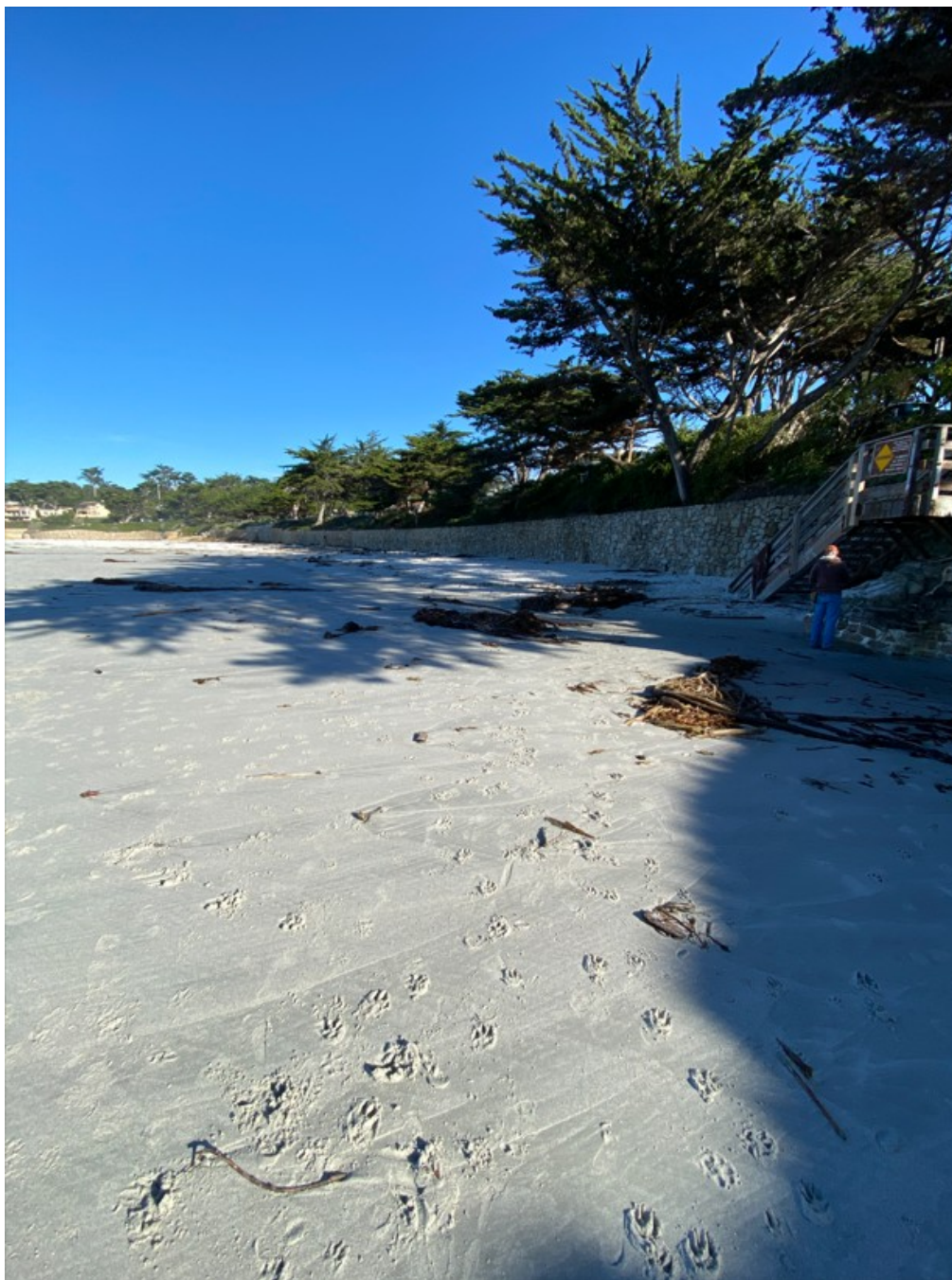
Photograph 3: Seawall S2 on December 22, 2022
