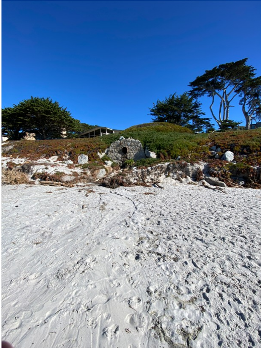
Photograph 89: Revetment R5 and Seawall S9, Showing Small Amount of Riprap Boulders on January 30, 2023
