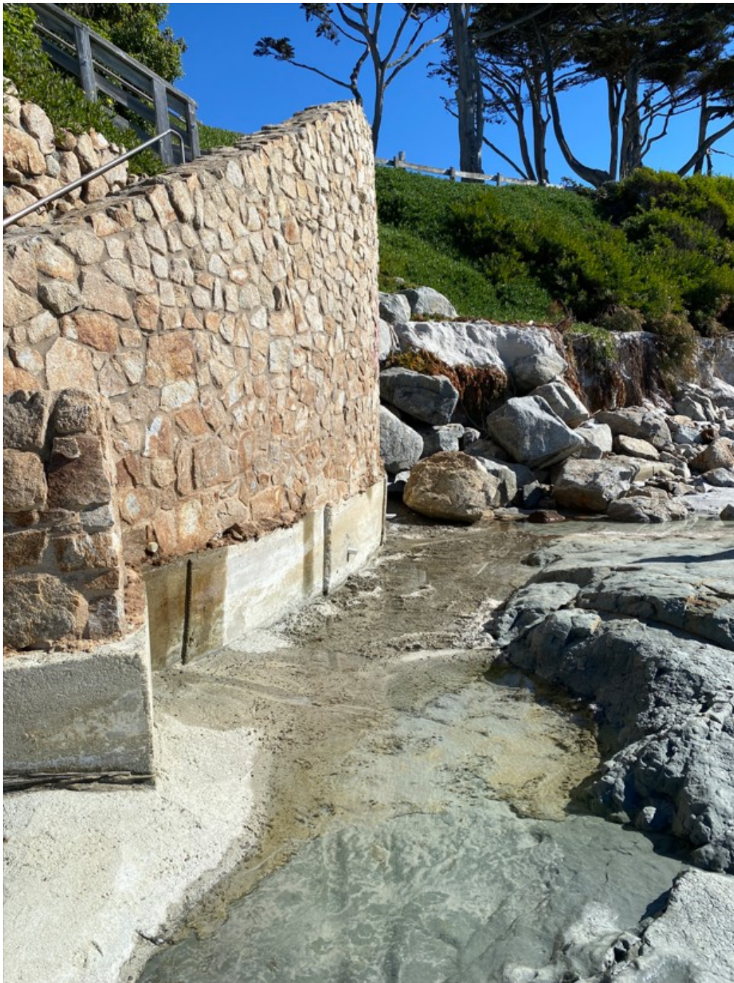
Photograph 68: South Foundation of Seawall S7 on January 30, 2023
