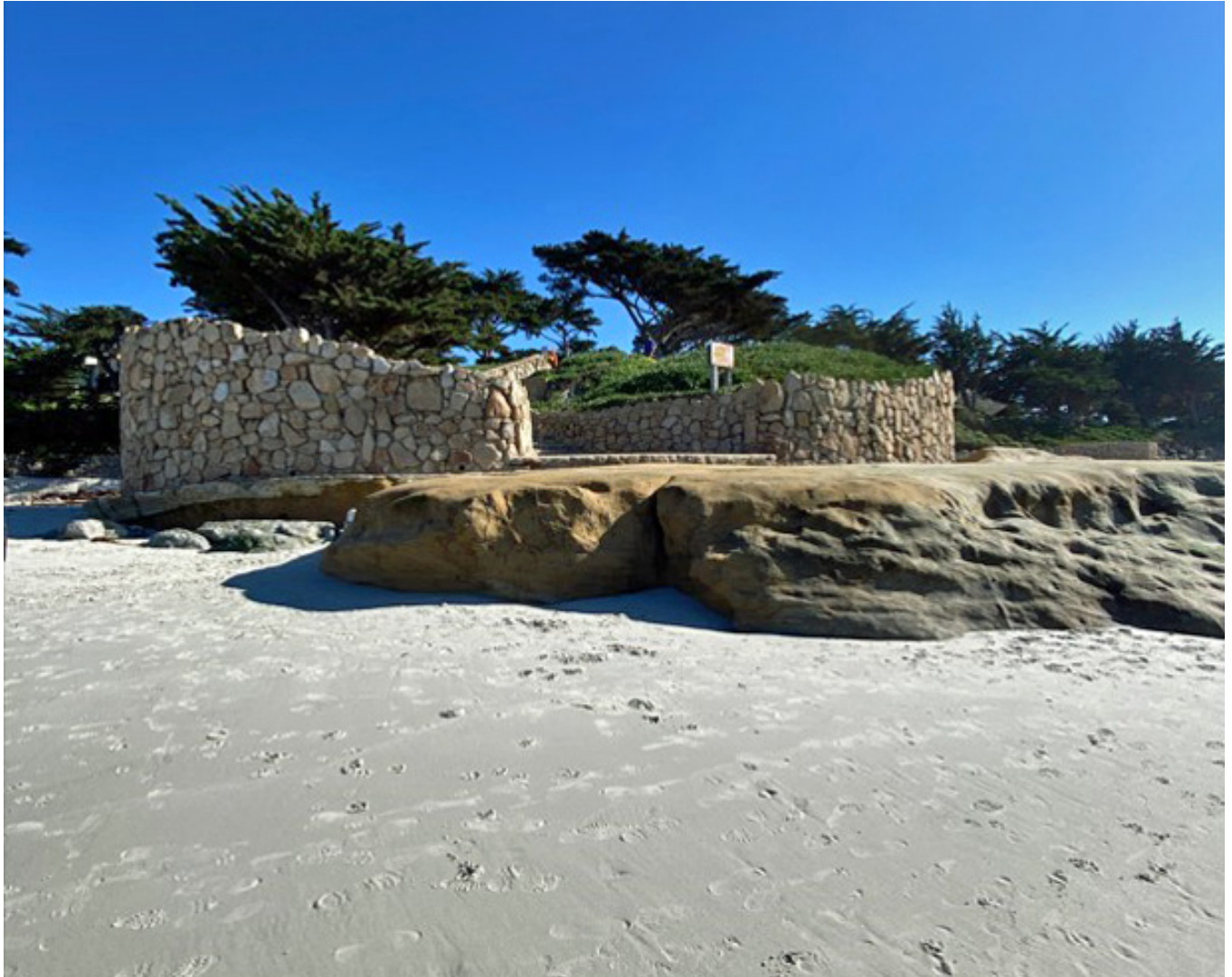
Photograph 28: Showing Public Access Stairway ST3 with Seawall S3 on Both Sides On January 30, 2023
