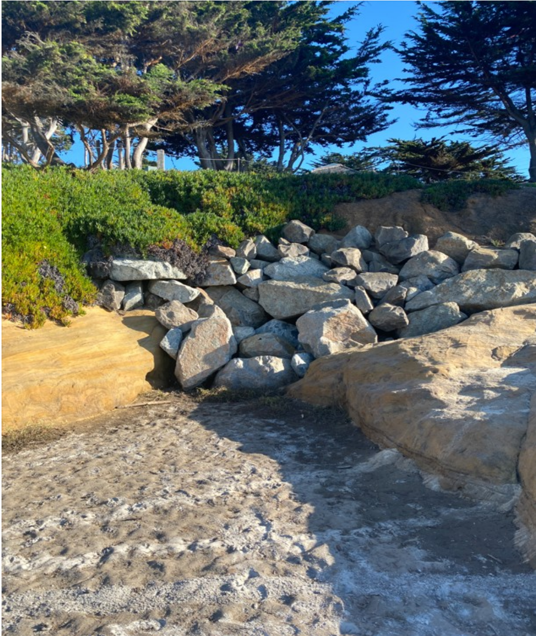
Photograph 19: Revetment R1 on December 22, 2022
