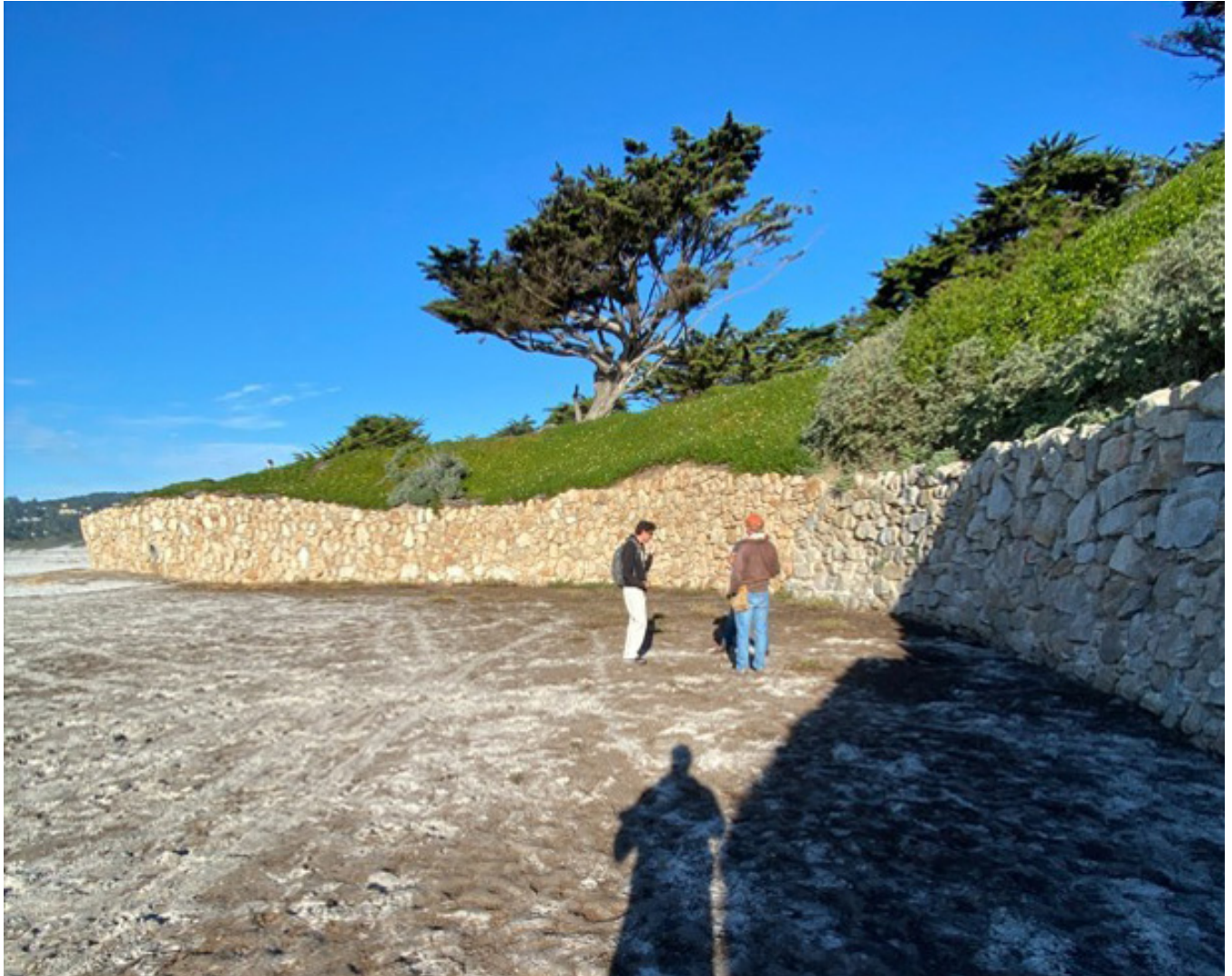
Photograph 25: Looking North at Seawall S3 on December 22, 2022
