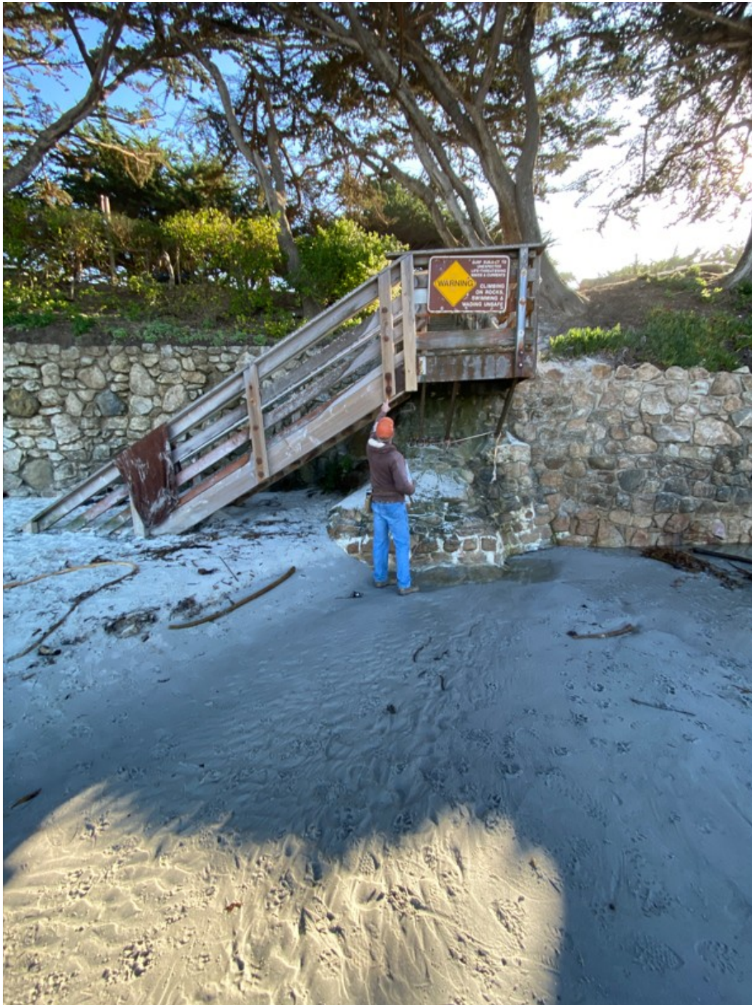
Photograph 4: Stairway ST1 on December 22, 2022
