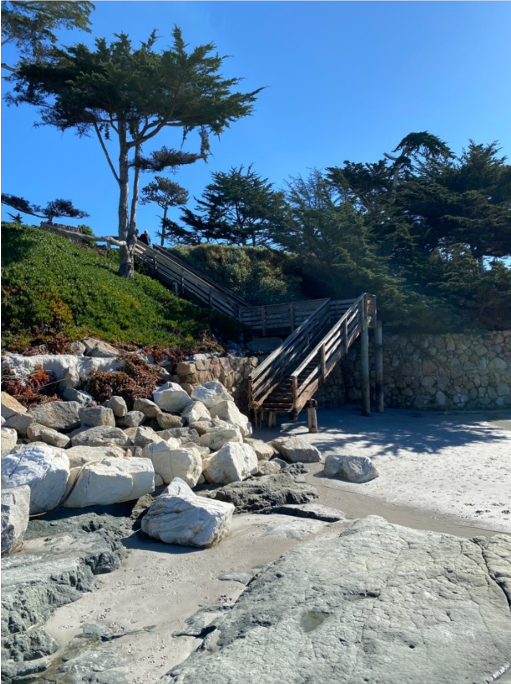
Photograph 73: Stairway ST7 on January 30, 2023
