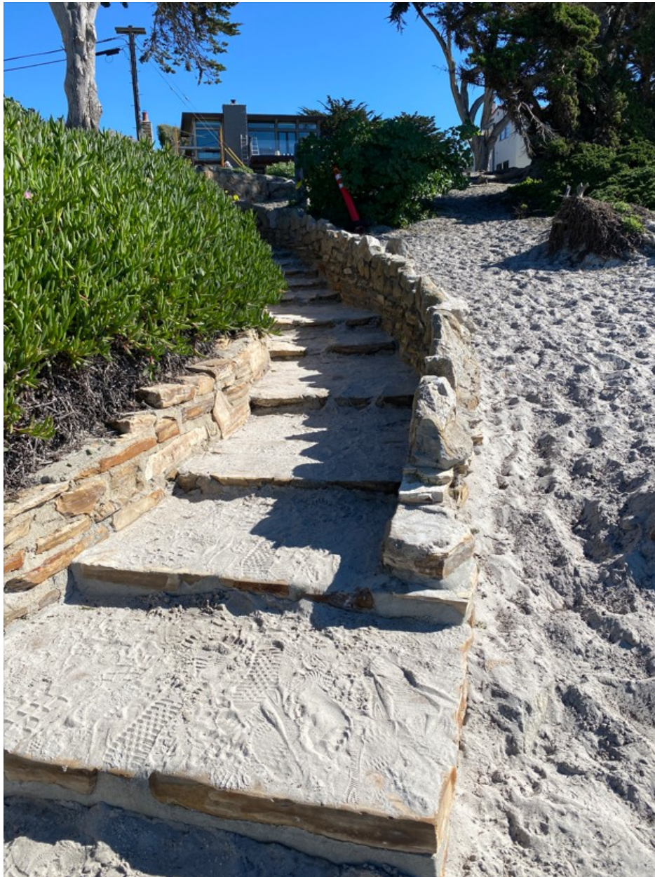
Photograph 86: Stairway ST9 on January 30, 2023
