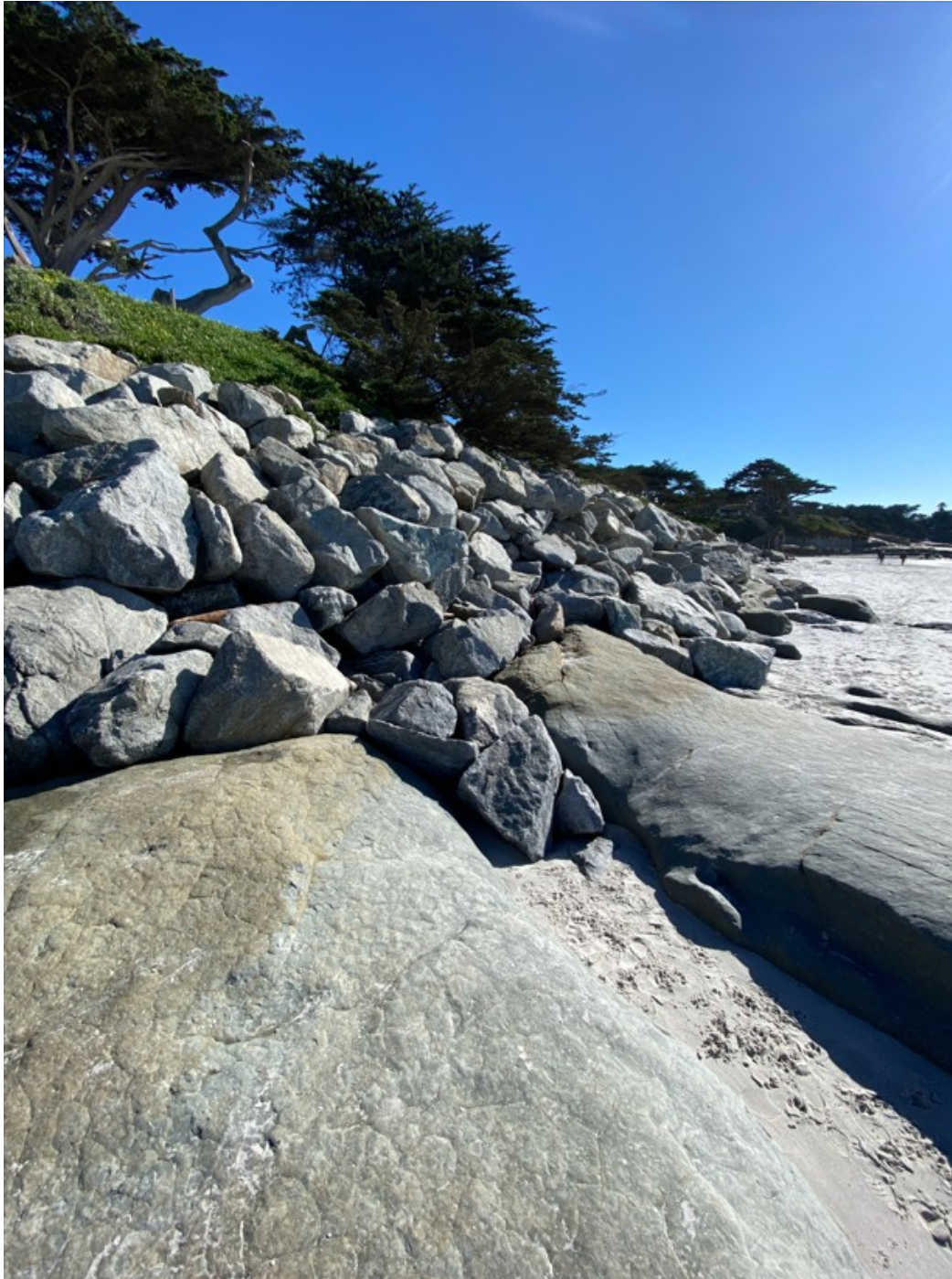
Photograph 53: Profile View of Revetment R3 on January 30, 2023
