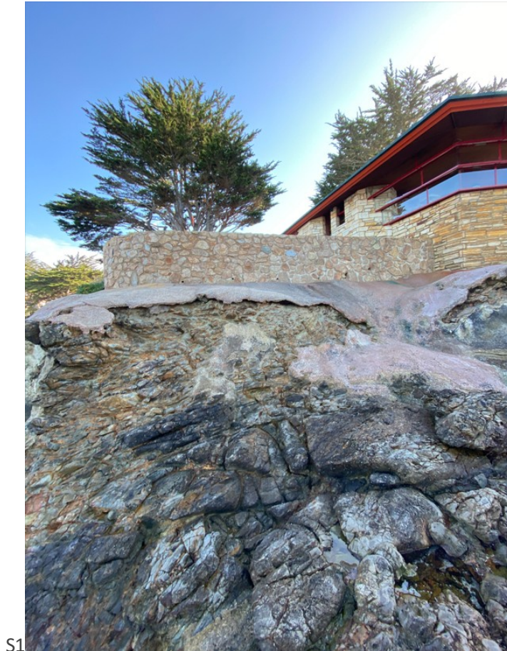
Photograph 1: Privately Owned Seawall S1 on December 22, 2022
