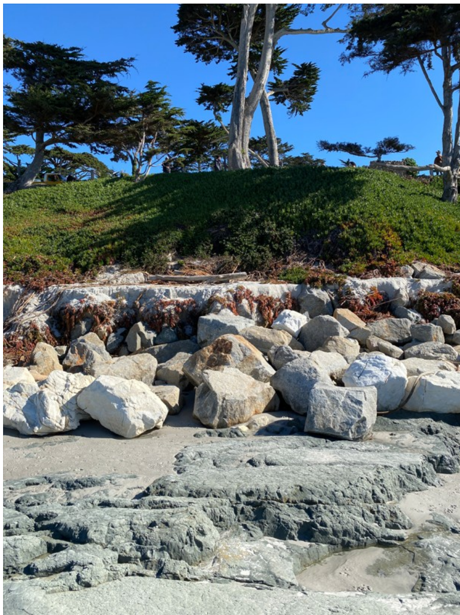
Photograph 75: South Portion of Revetment R5 on January 30, 2023 Showing Bedrock Platform Below Beach Sand and Old Erosional Scarp in Ice Plant Above Revetment
