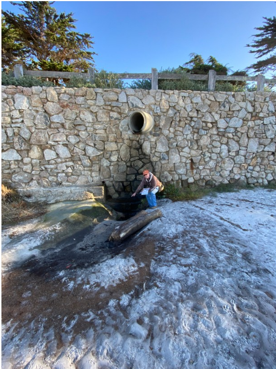
Photograph 10: Storm Drain near NorthNorthern End of Seawall S2 on December 22, 2022
