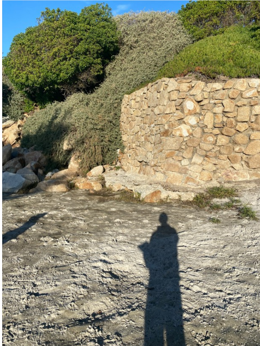
Photograph 32: North End of Seawall S3 on December 22, 2022
