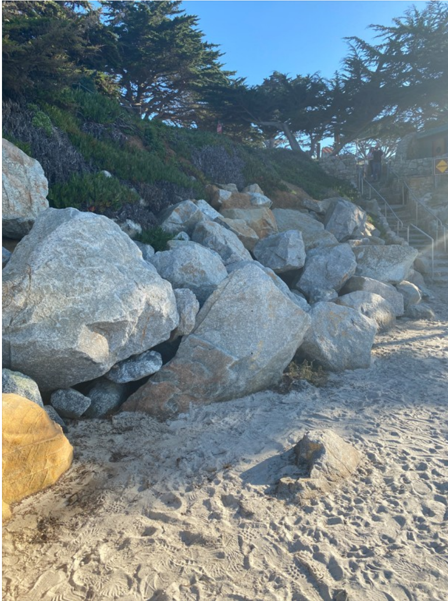
Photograph 17: Revetment R1 on December 22, 2022
