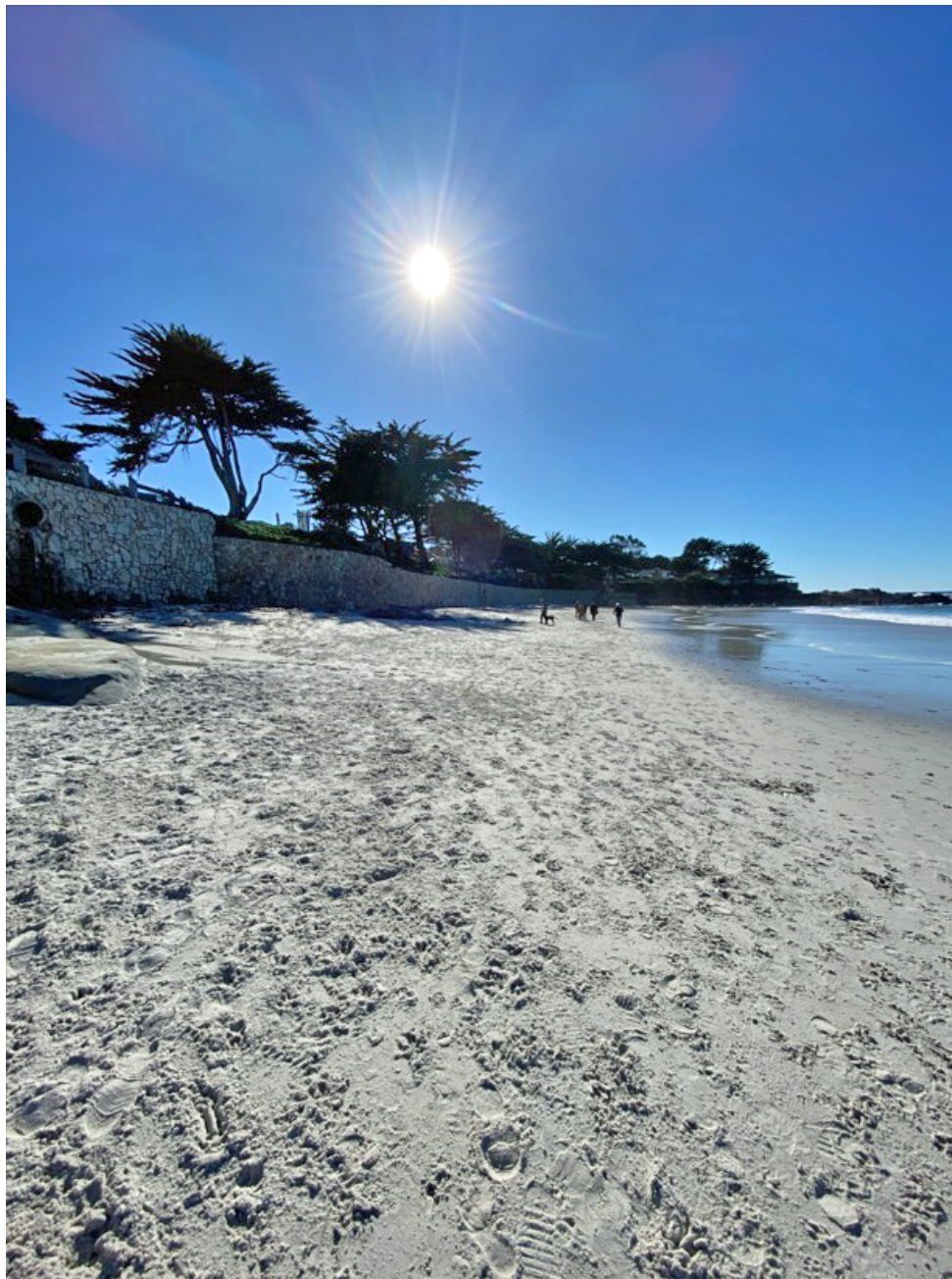
Photograph 8: Showing Seawall S2 on January 30, 2023
