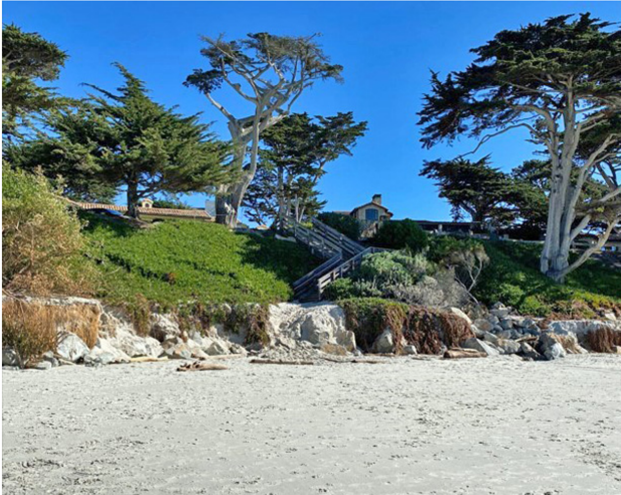
Photograph 79: Showing Beach Access Stairway ST8 on January 30, 2023
