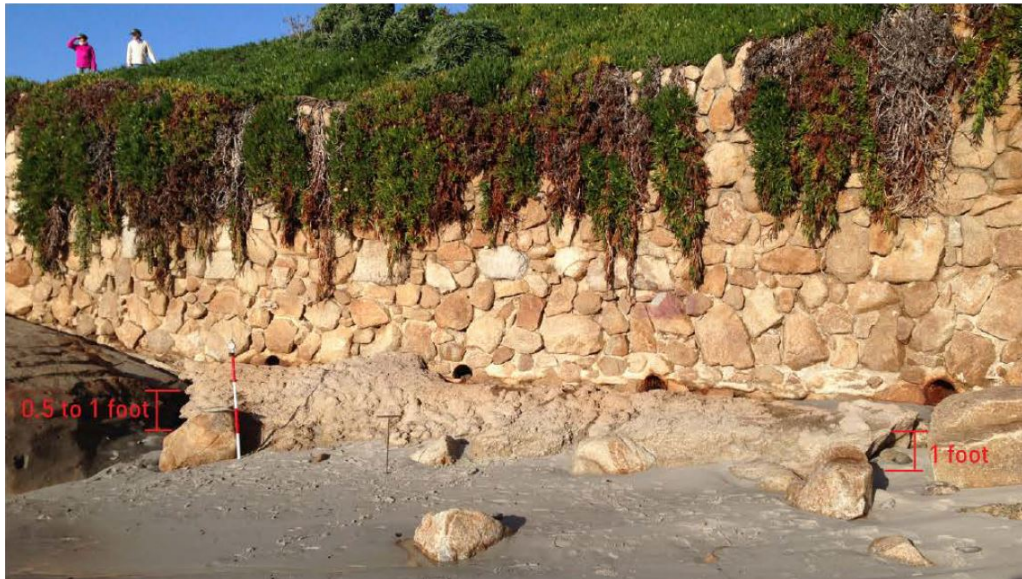
Photograph 24: Southern End of Seawall S3 in February 2016 Photographed by Easton Geology Showing Pumped Concrete Repair of Undermining of Seawall S3
