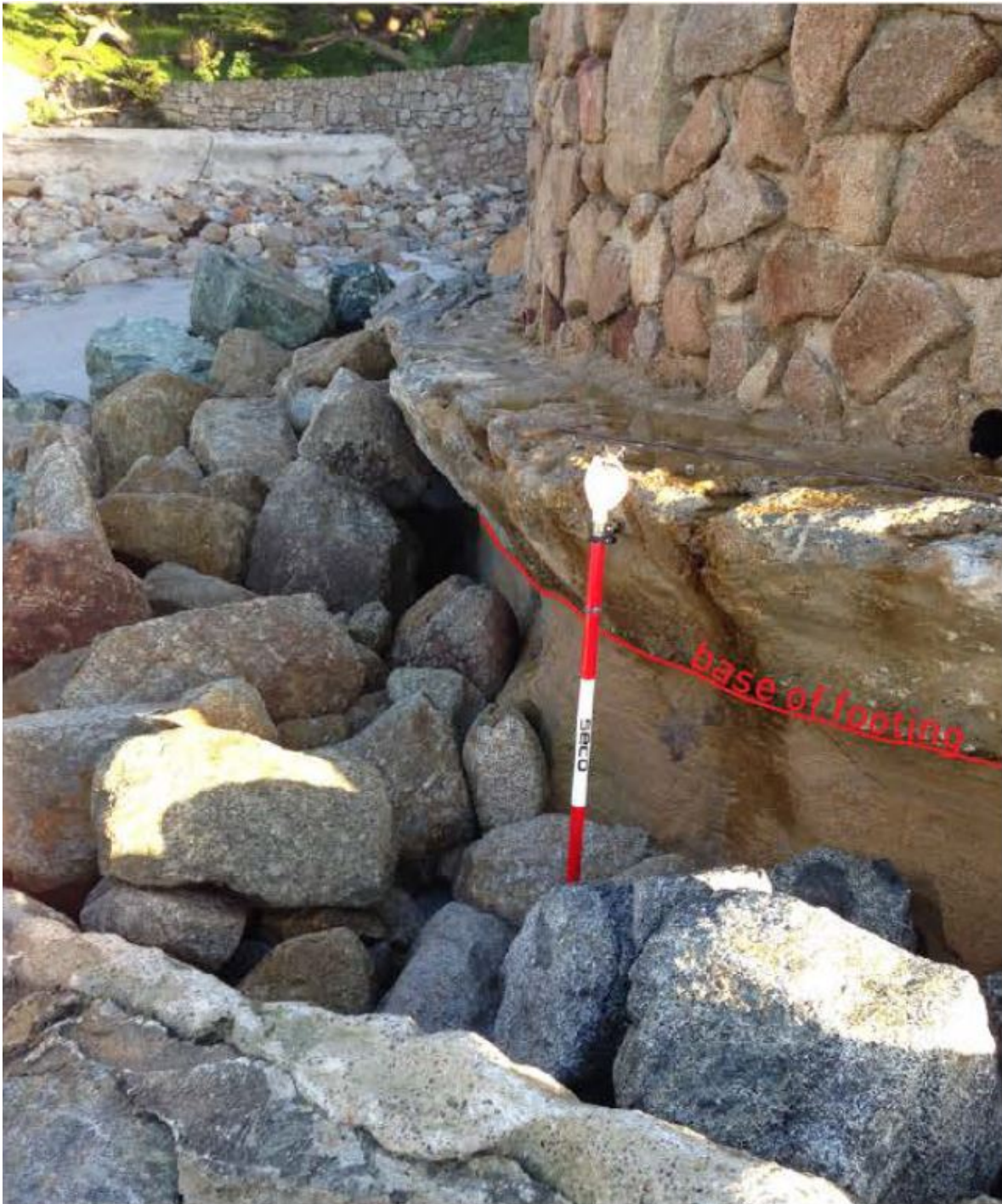
Photograph 30: Seawall S3 Just North from ST4 in February 2016 (Easton Geology)
