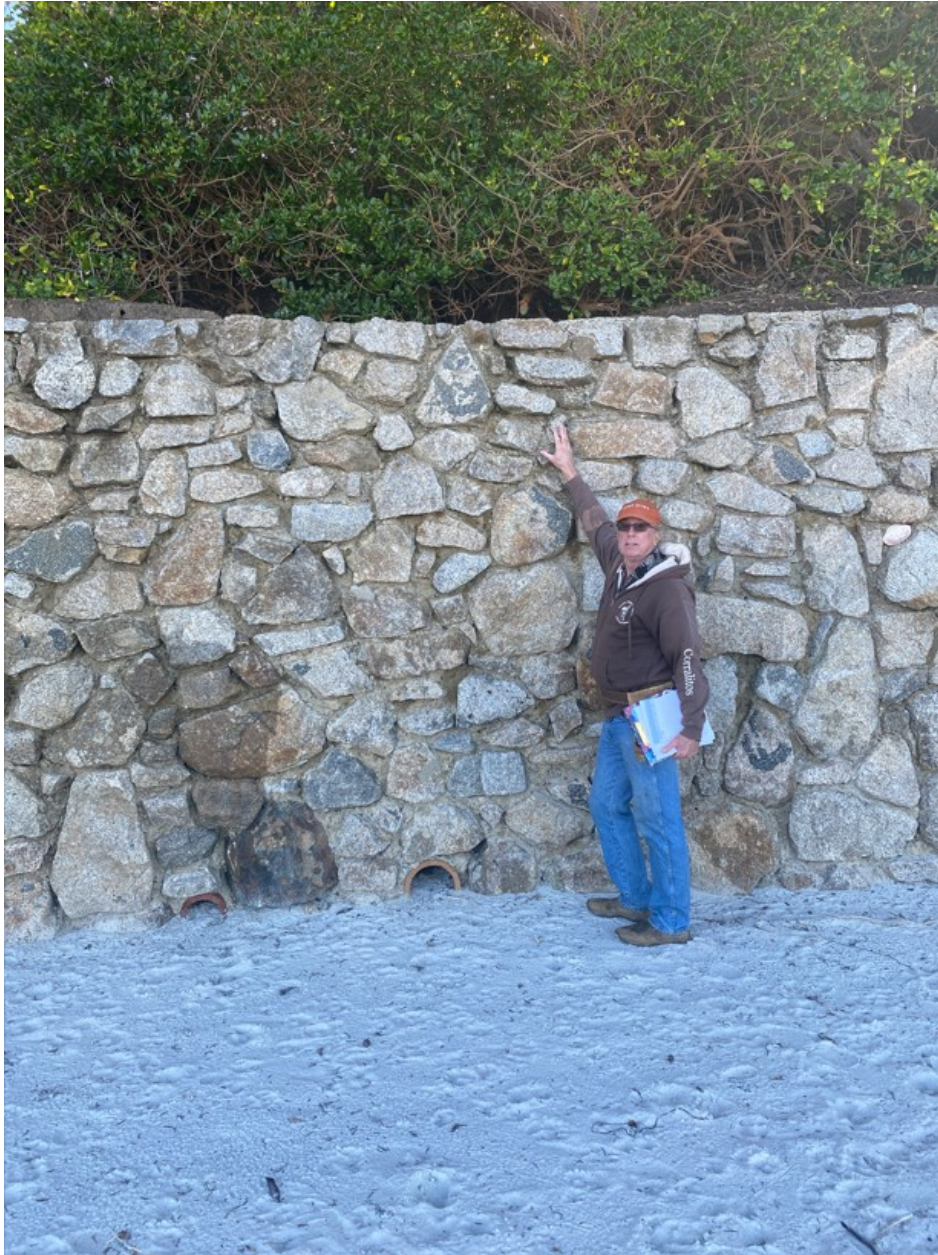
Photograph 9: Seawall S2 on December 22, 2022
