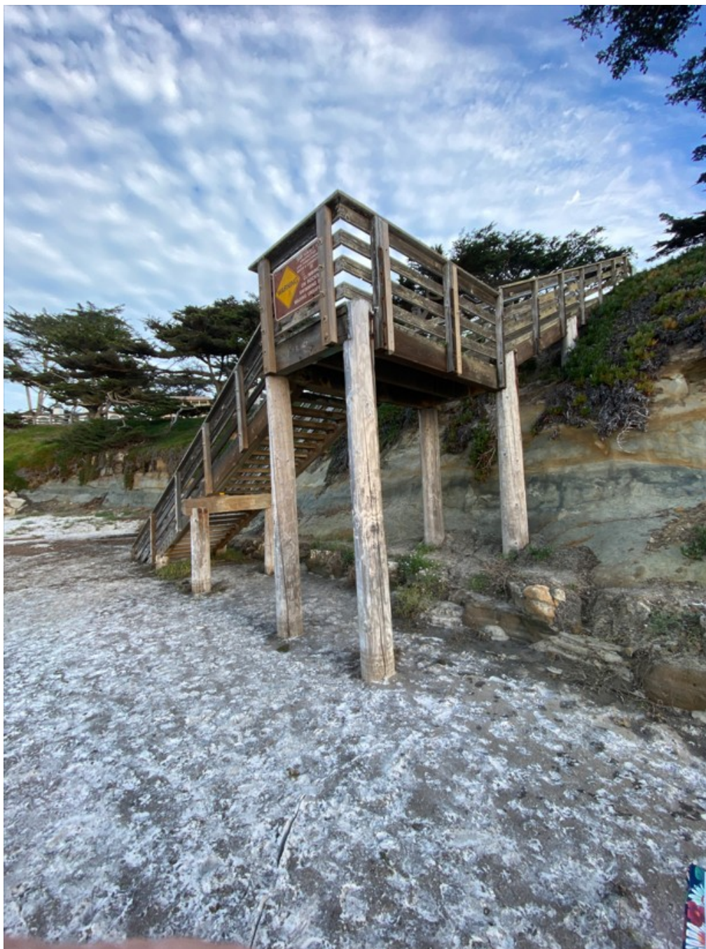
Photograph 38: Showing Public Access Stairway ST4 on December 22, 2022
