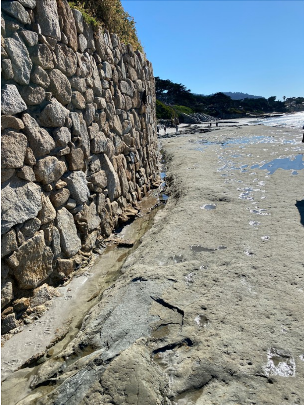
Photograph 71: Seawall S7 Foundation on January 30, 2023
