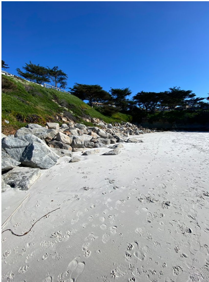
Photograph 49: Showing Revetment R3 Looking South on January 30, 2023
