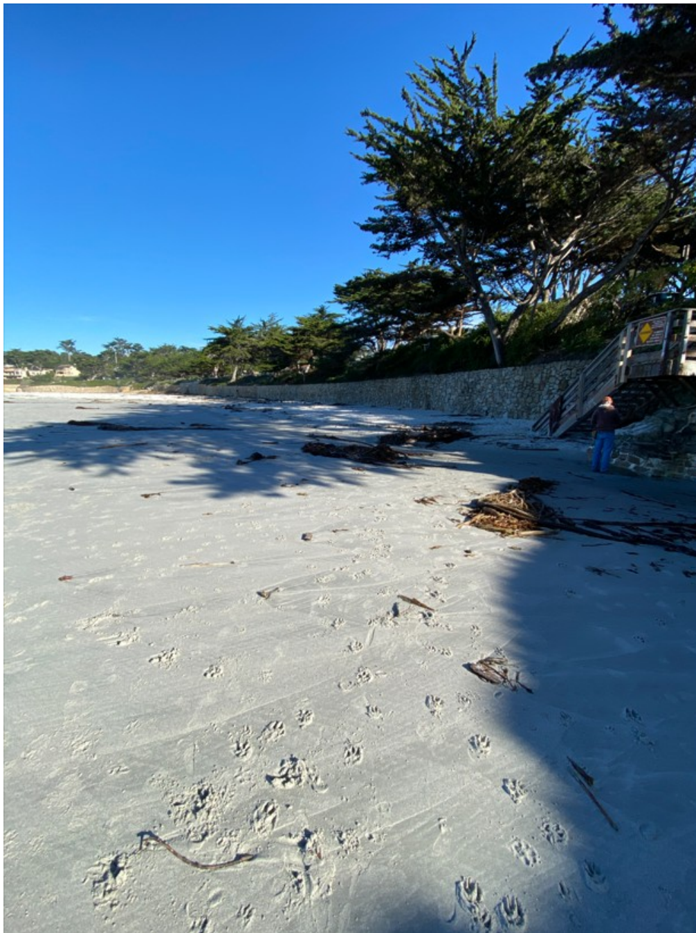
Photograph 3: Seawall S2 on December 22, 2022
