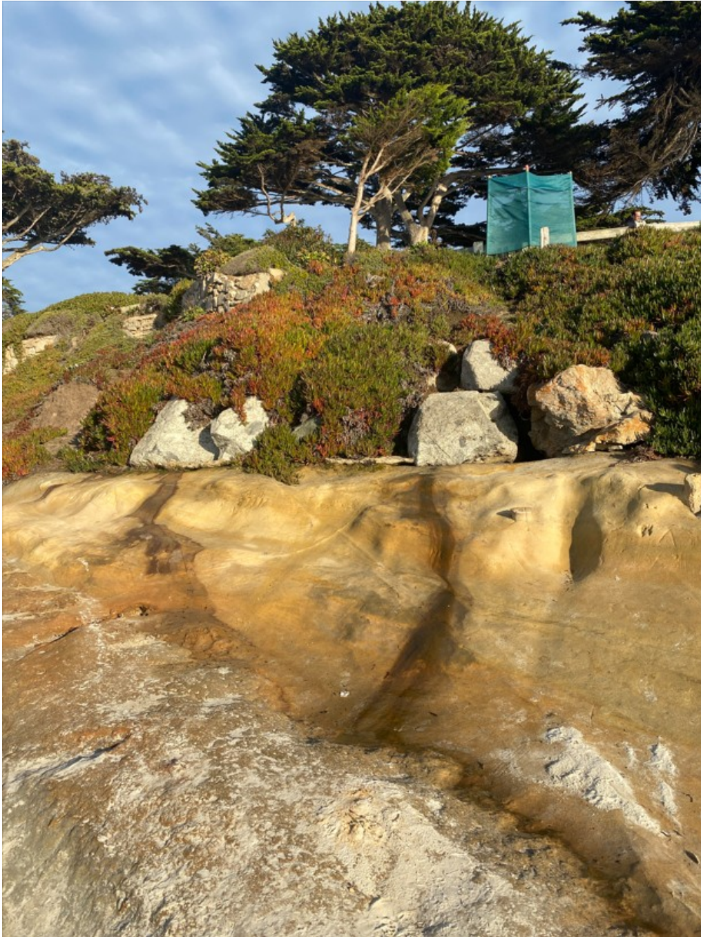
Photograph 37: Showing Unnamed Rip-rap Boulders North of Seawall S4 on December 22, 2022
