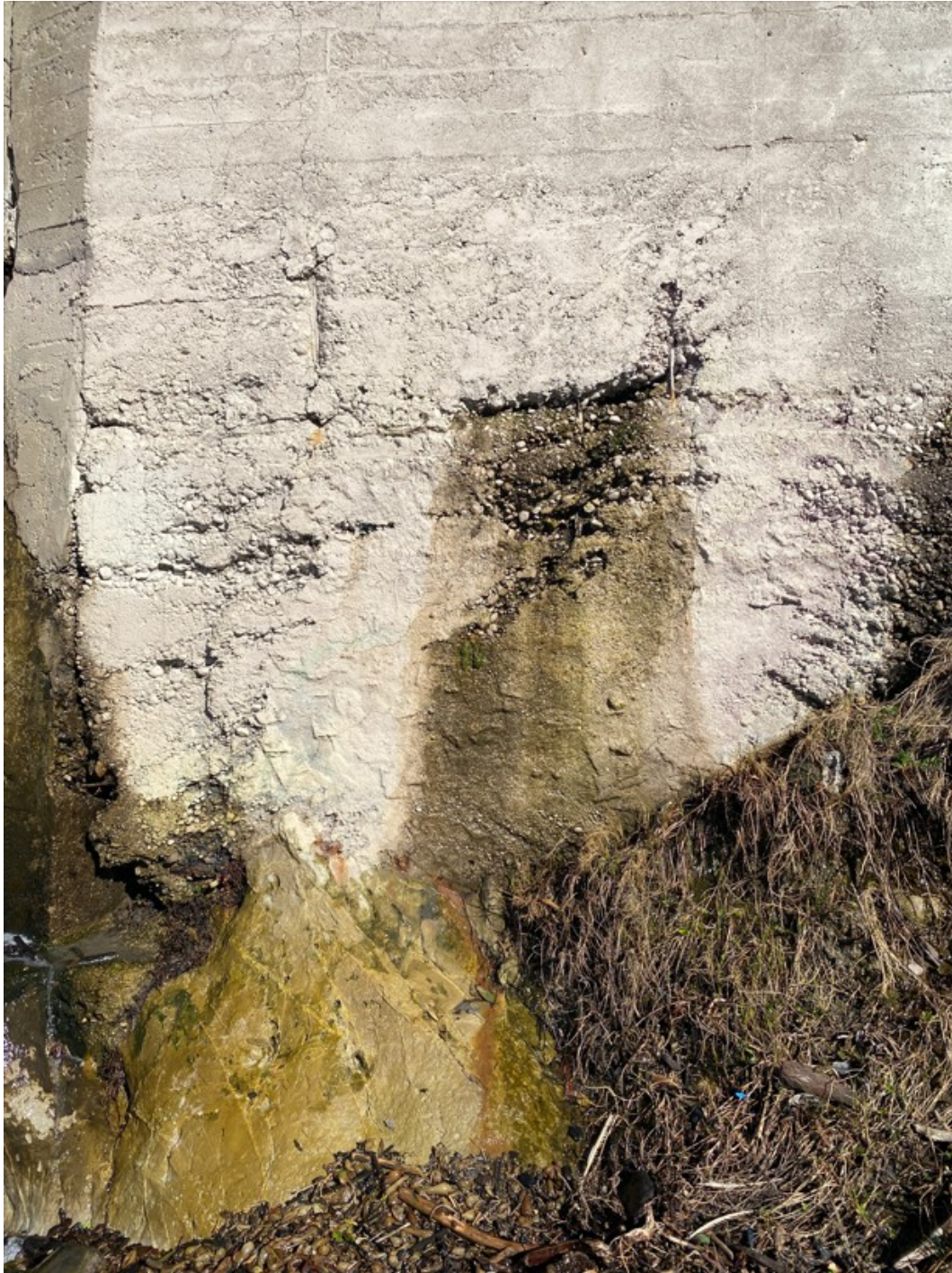
Photograph 93: Central Part of Foundation of Seawall S10 on January 30, 2023
