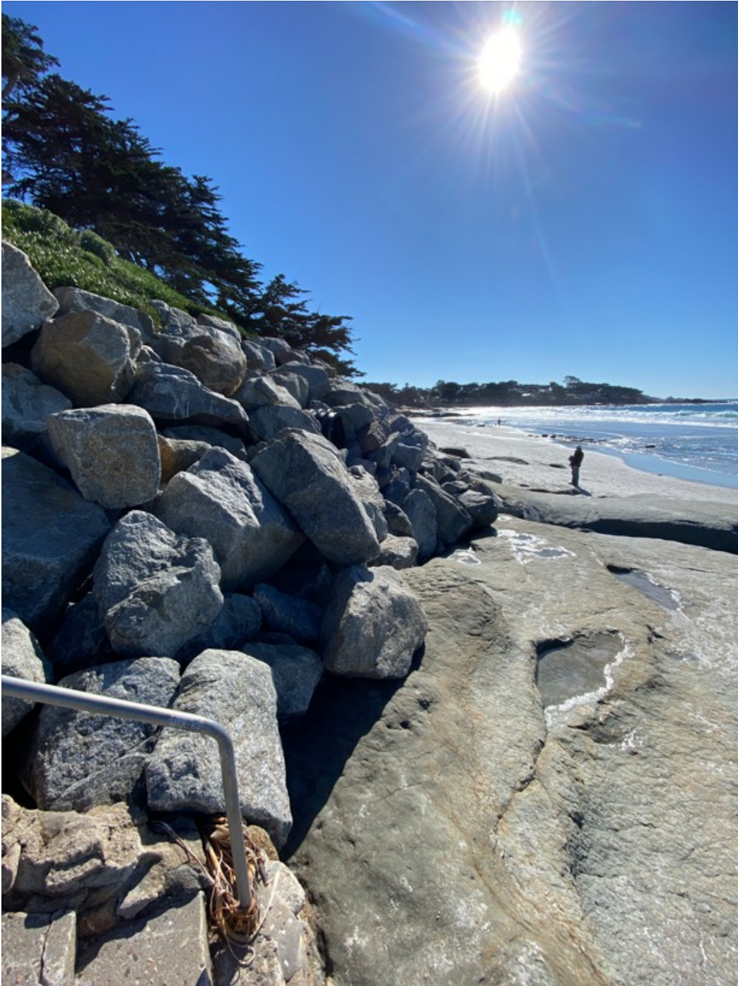
Photograph 55: Another Profile View of Revetment R3 on January 30, 2023
