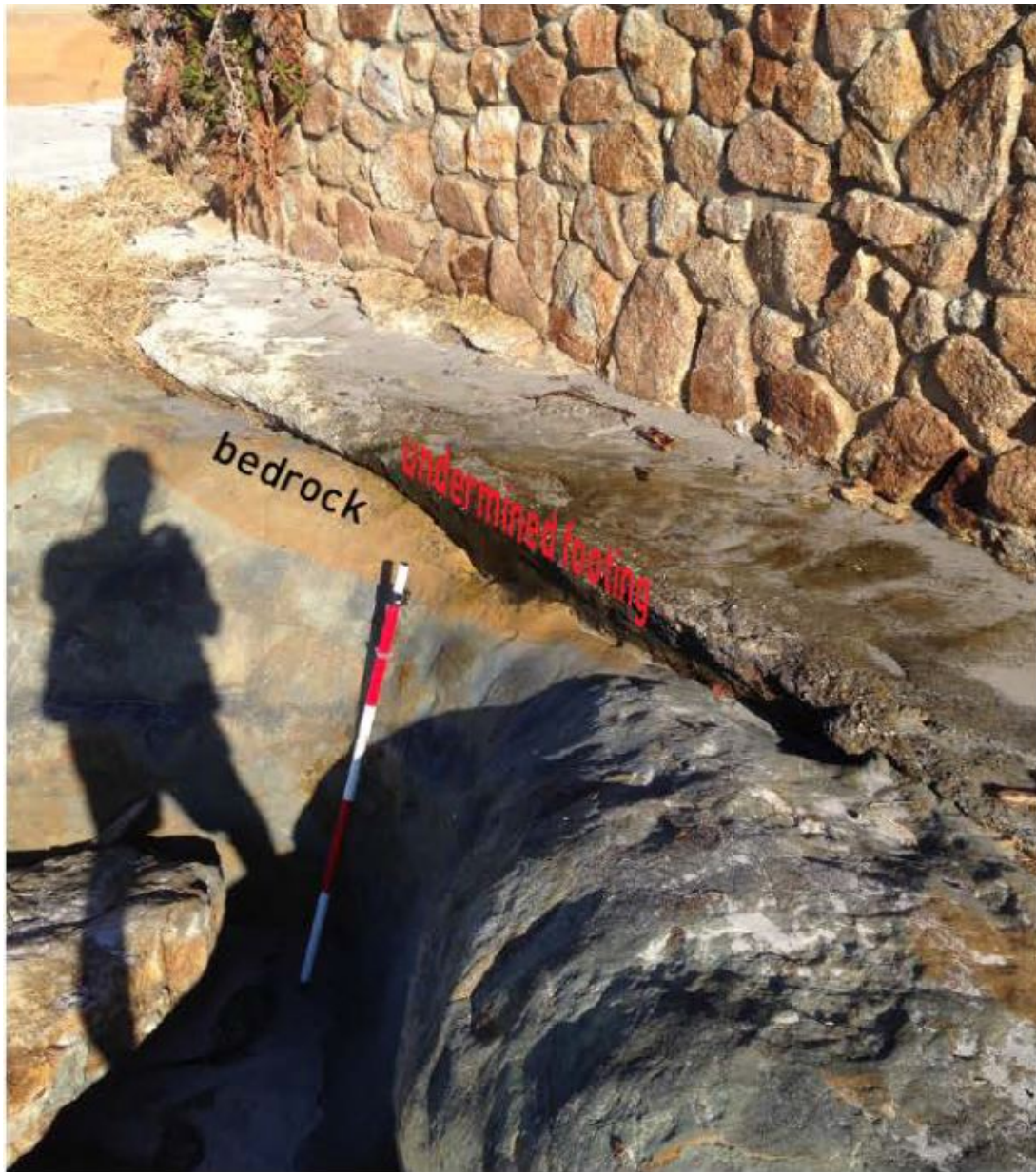
Photograph 12: Easton Geology Photograph of the North End of Seawall S2 in June 2016
