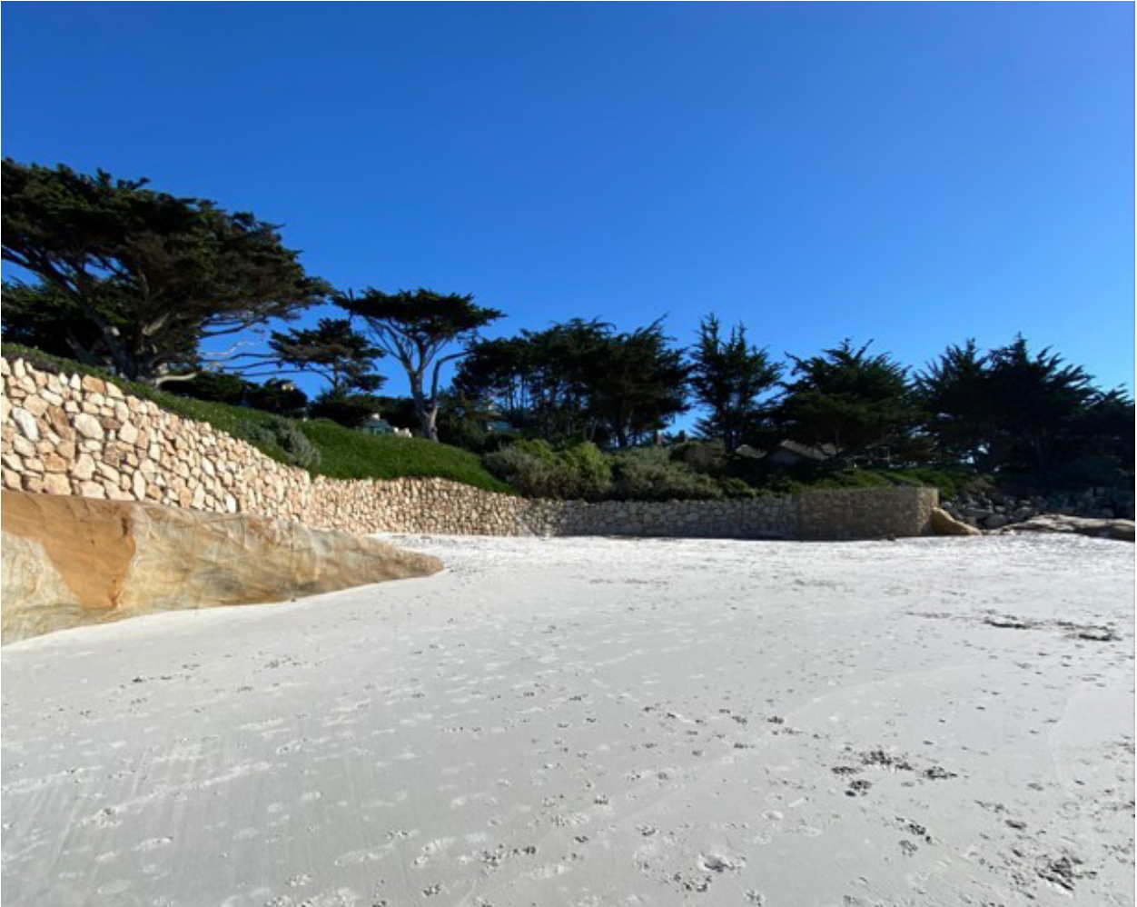
Photograph 35: Showing Seawall S4 on January 30, 2023
