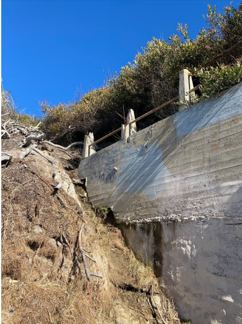
Photograph 94: Seawall S10 on January 30, 2023
