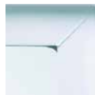
Vinyl sash corner seam
