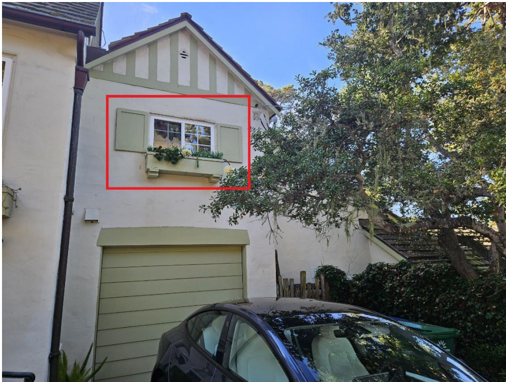
Figure 2: View of the kitchen window on north elevation to be replaced.
