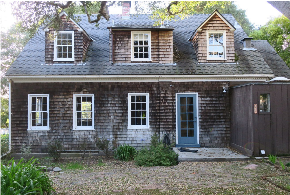
Rear elevation, view looking west. Addition proposed for the non-historic vertical wood laundry room.
