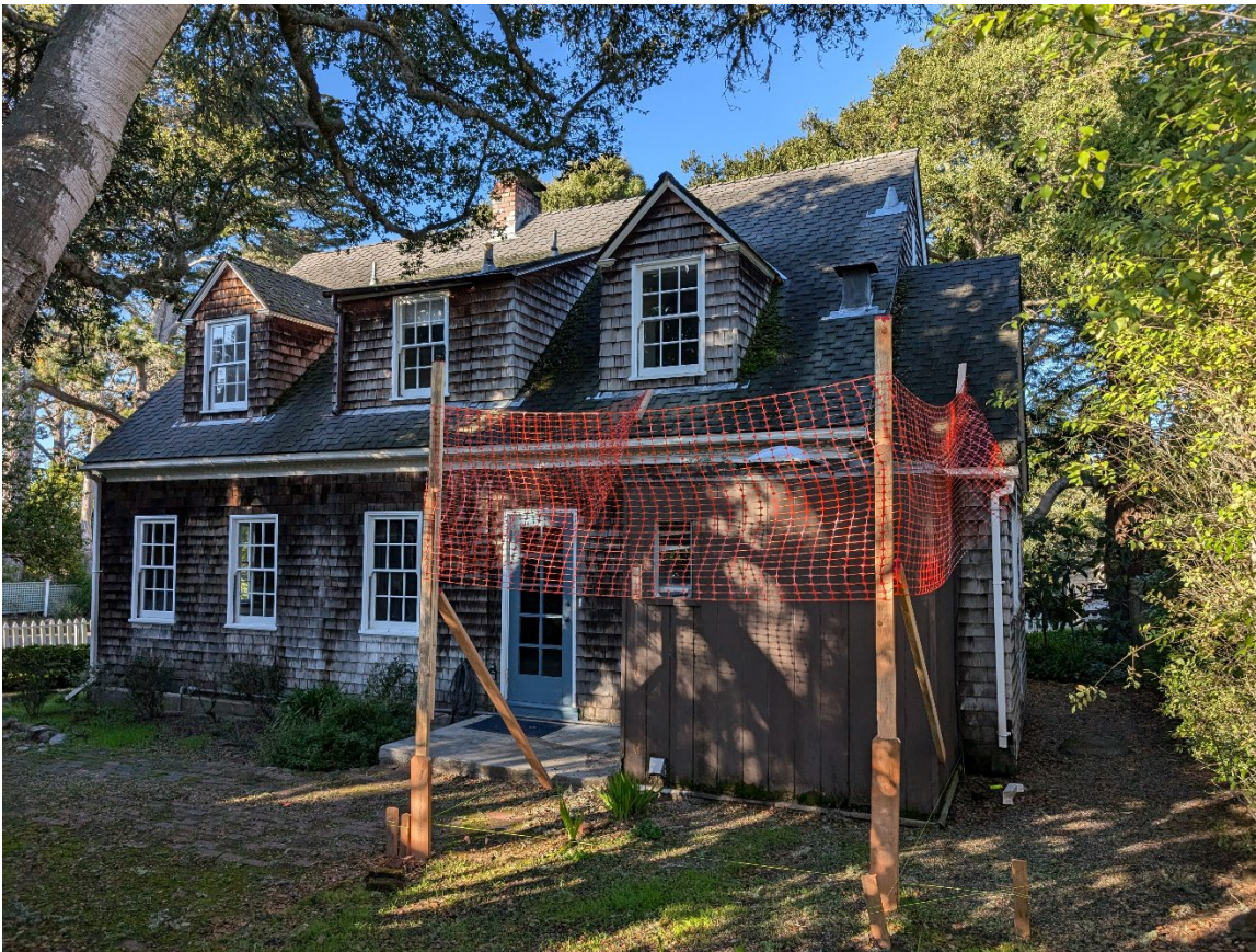
Rear elevation, view looking west. Addition proposed for the non-historic vertical wood laundry room.
