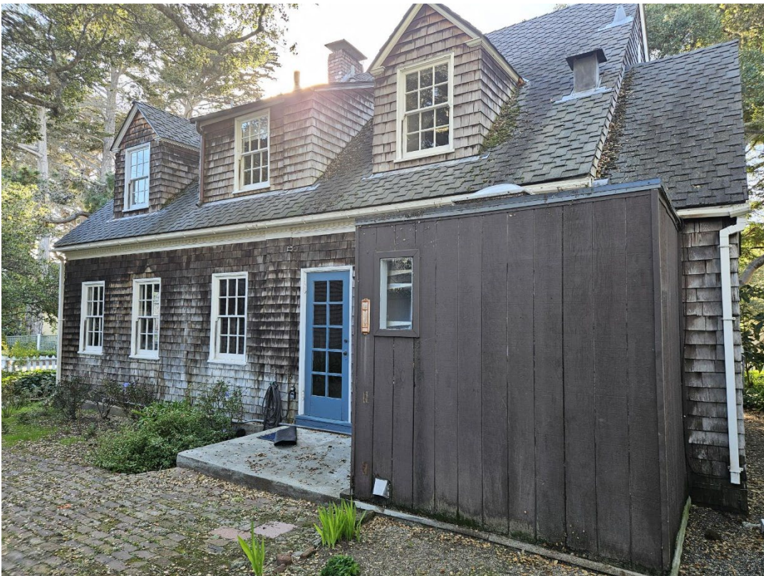
Figure 2: View of the rear elevation and laundry room addition.
