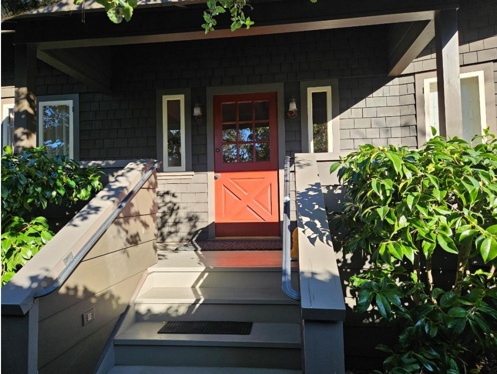
Figure 5: View of front porch.
