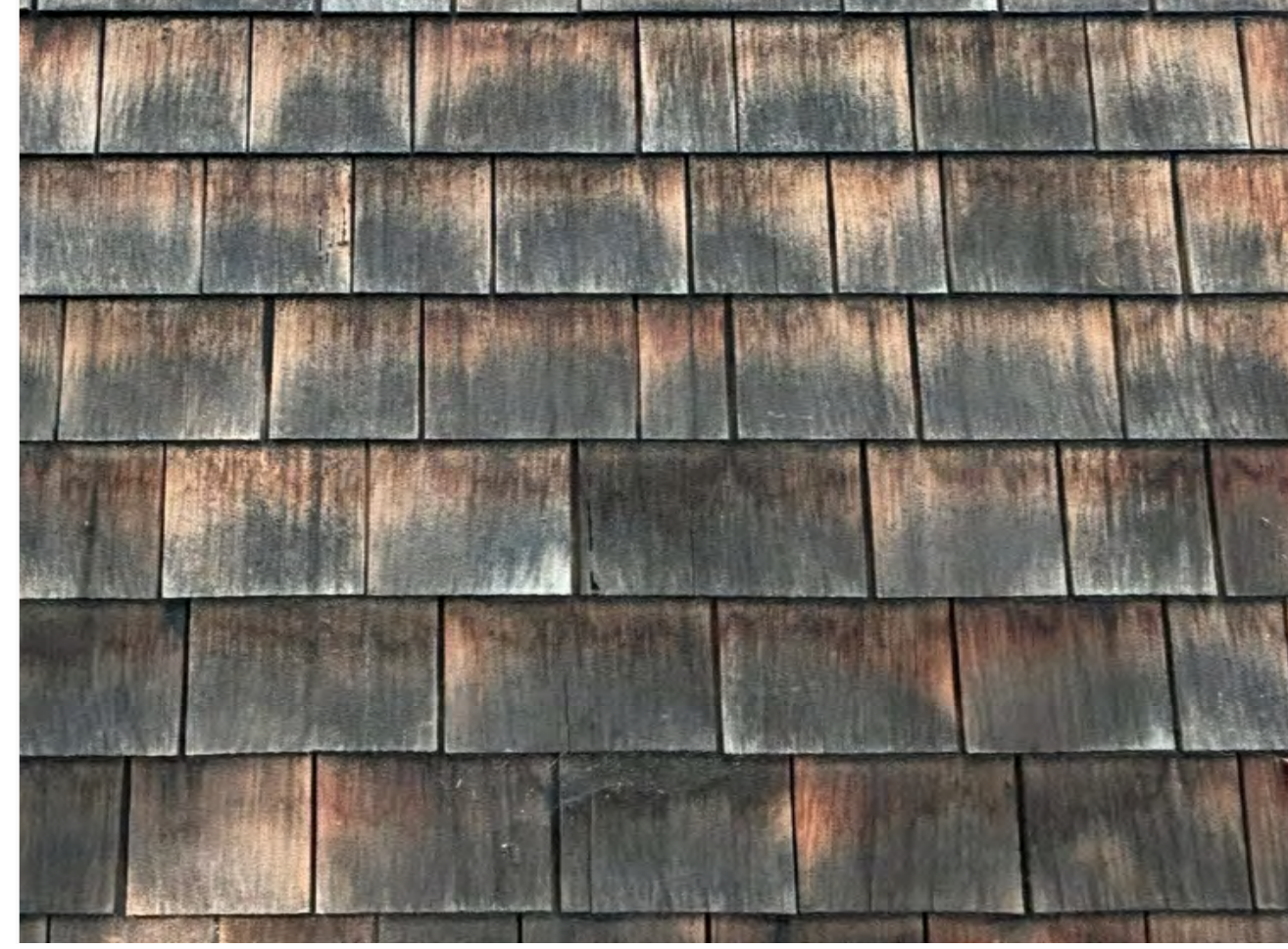
S WOOD SHAKE SIDING
