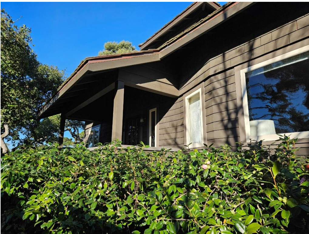
Figure 6: View of front porch showing shed roof.
