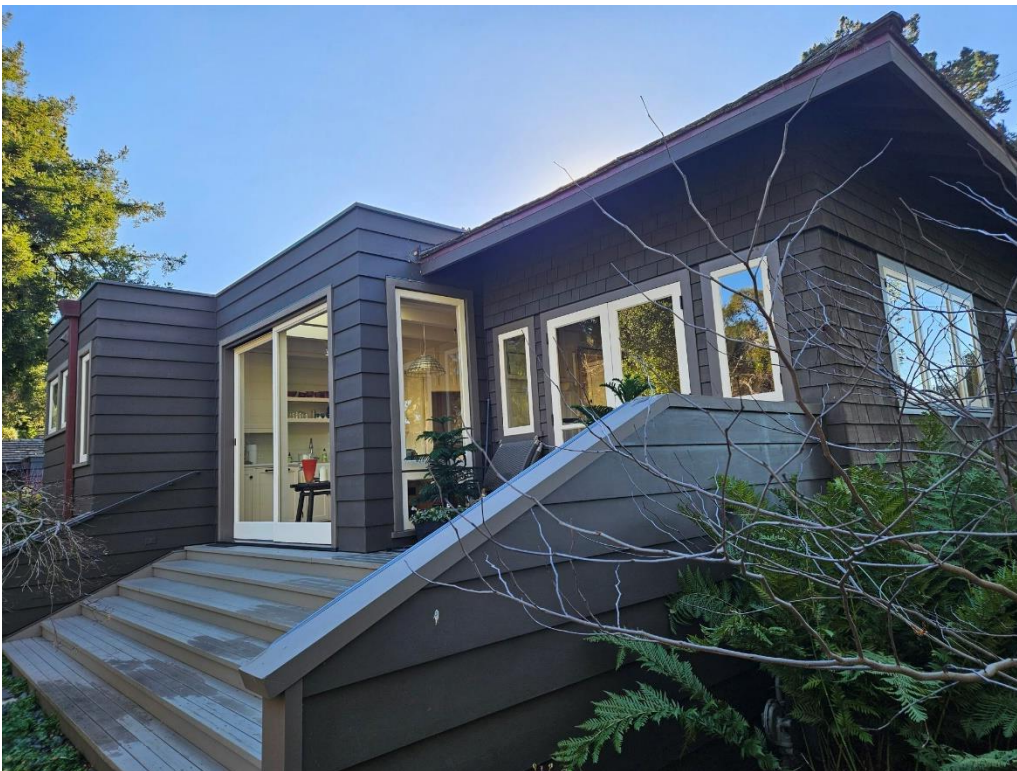
Figure 4: North elevation showing 2010 remodel.
