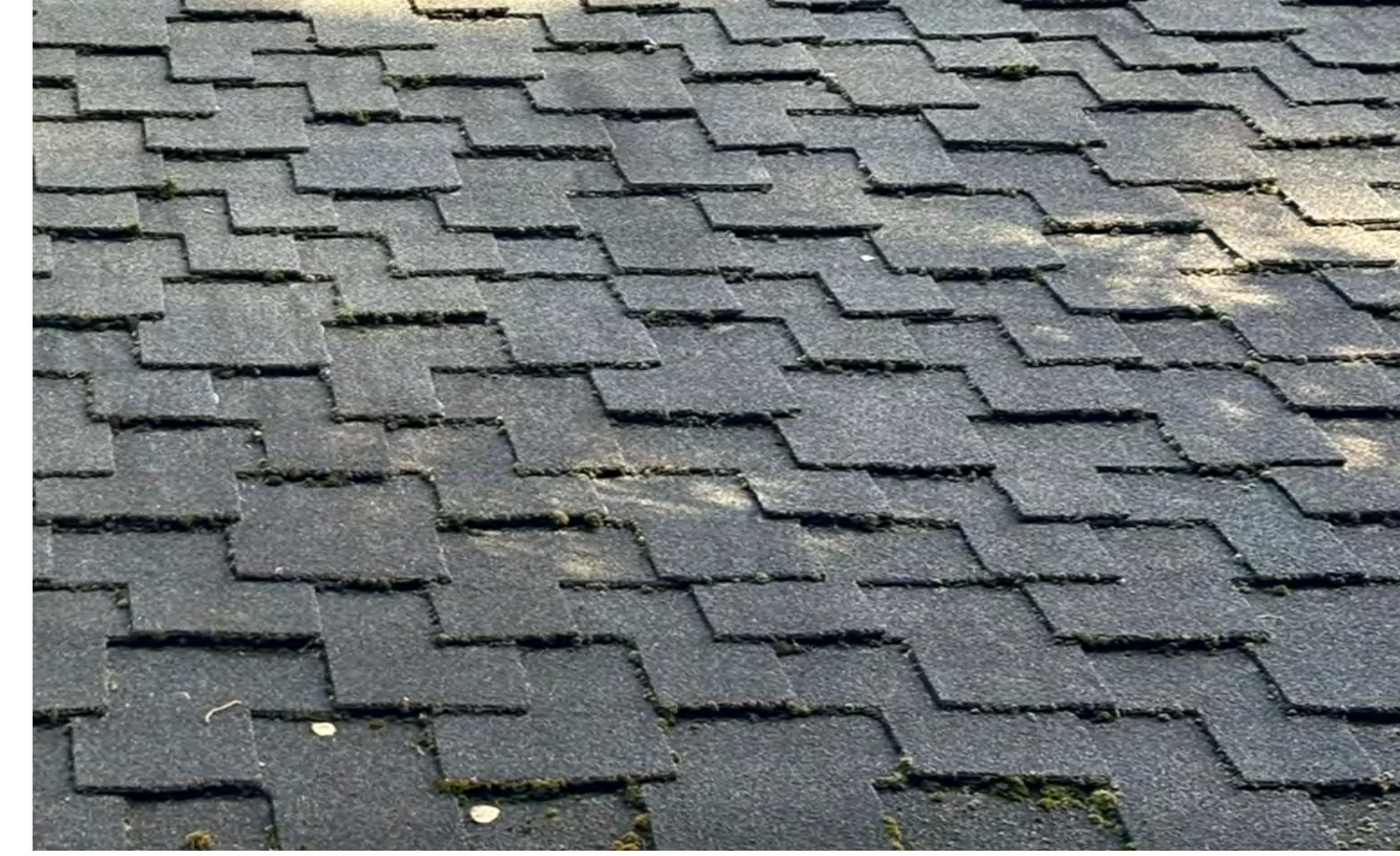
R COMPOSITION SHINGLE ROOFING
