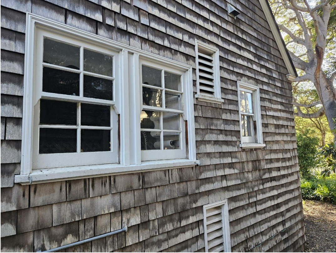
Figure 3: View of north elevation addition and windows to be removed.
