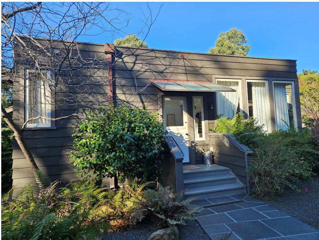
Figure 2: Addition (2010) on east elevation.
