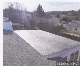
Project Gallery - Flat IB PVC Roofs... gonzalesroofing.com
