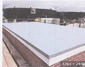
PVC Roofing - Roofing Contractor - O... orezonabuildingcompany.com
