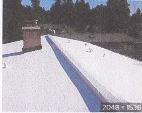
Edmonds Low Slope PVC Roof - IB R... pinnacle Roofing Pros.com
