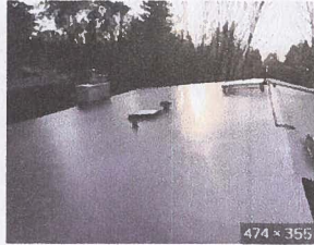
Kirkland IB PVC Roof Project | IB Roof... pinnacle Roofing Pros.com
