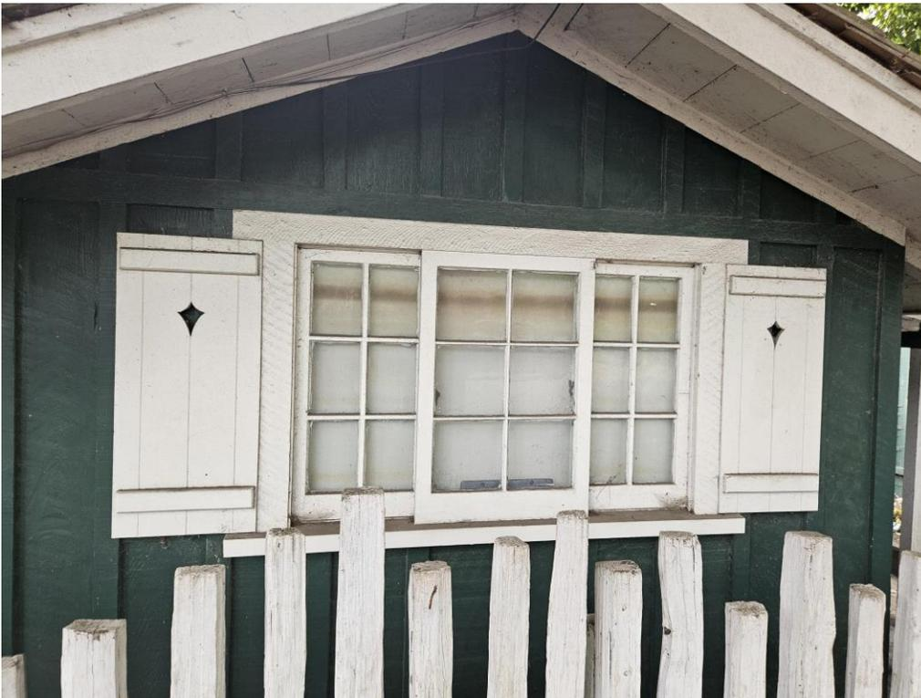
Figure 2: View of sliding wood sash, plank shutters, and extended lintels and sills.
