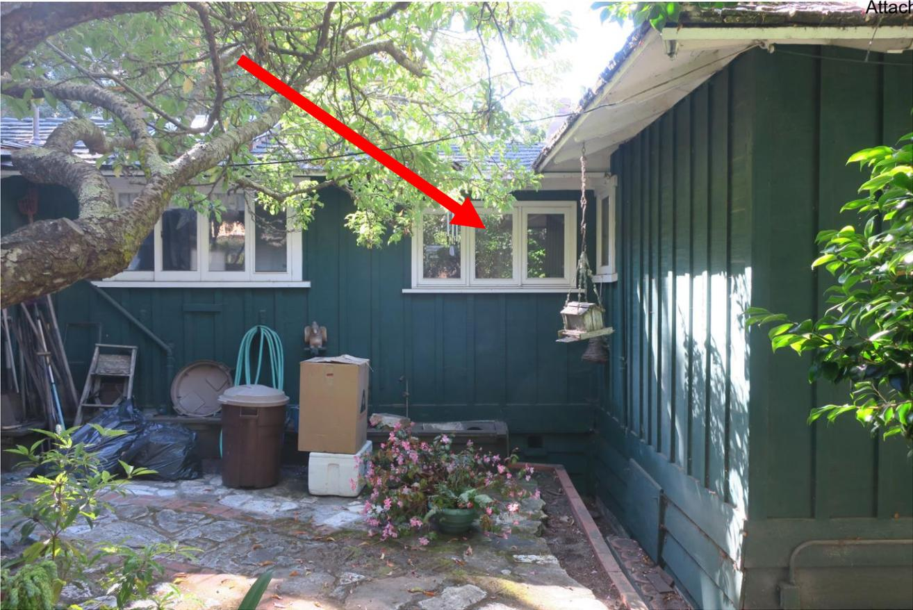
North side elevation, looking south. Arrow indicates non-original window (narrower sill, no extended lintel)
