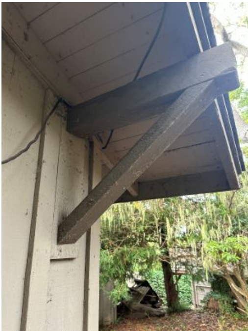
Figure 20 Knee brace at bedroom wing
