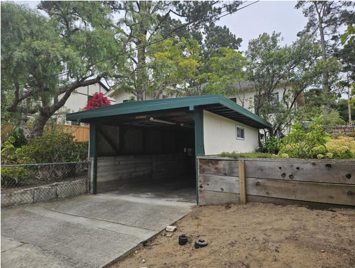
Figure 7: View of carport looking northeast.
