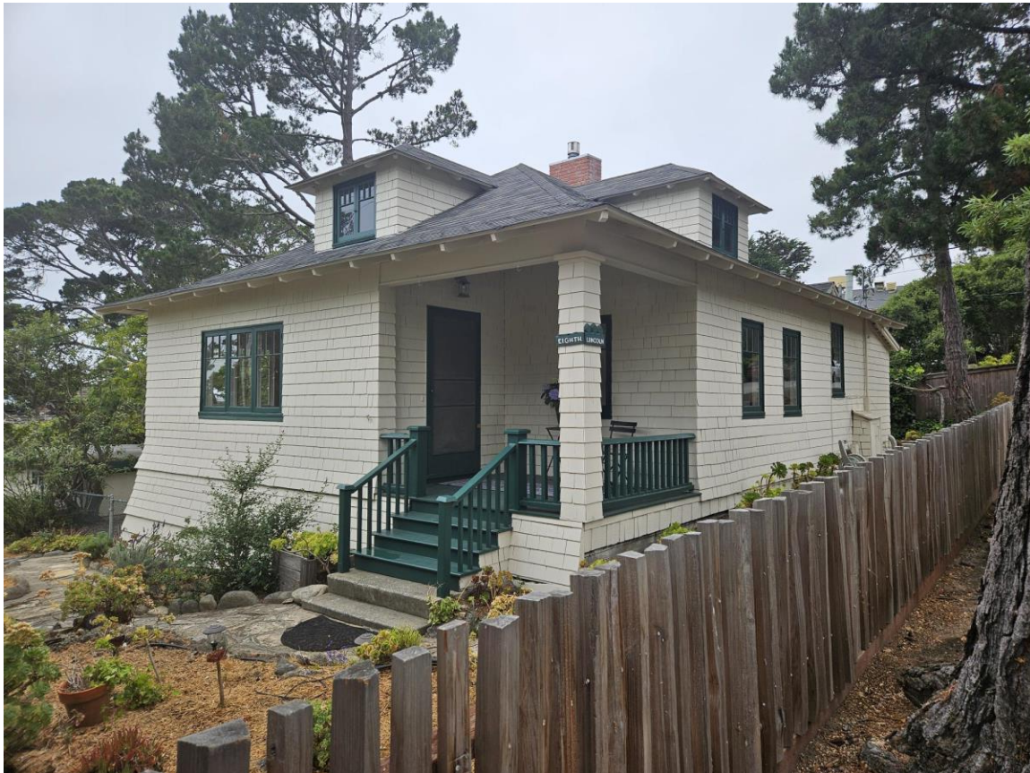
Front elevation looking northwest.
