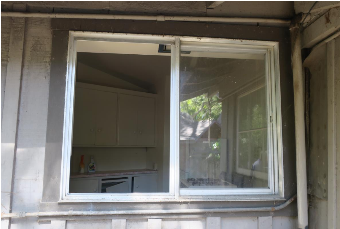
Aluminum slider window, left of service porch on rear elevation.
