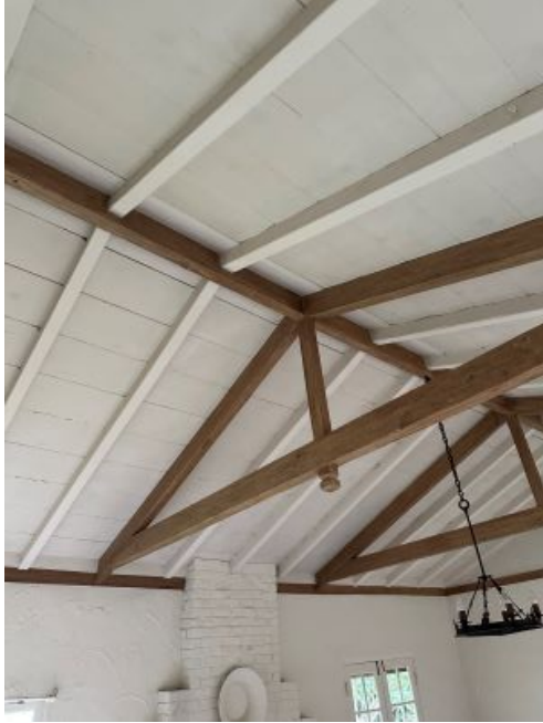
Figure 5 Roof framing in main room
