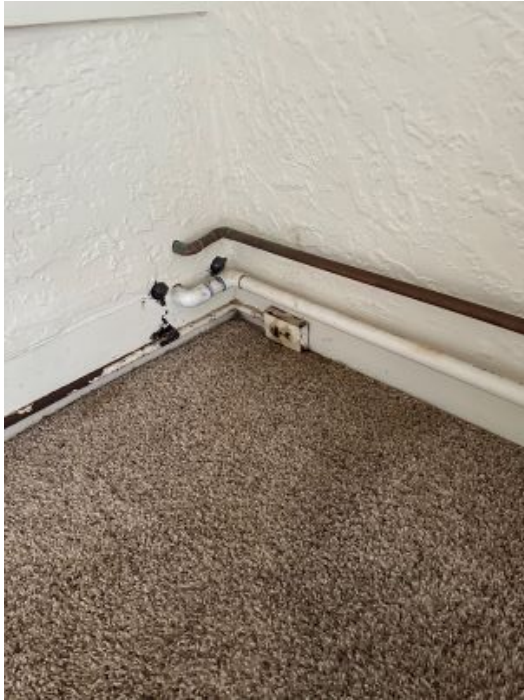
Figure 13 Surface run plumbing and electrical in bedroom
