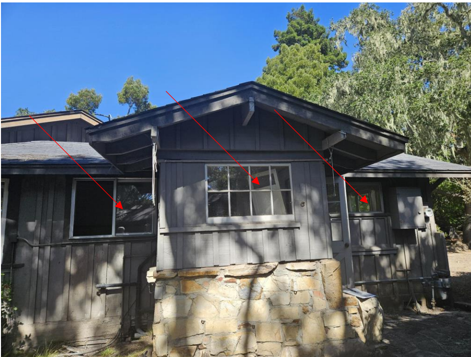
Figure 1: Window changes on south elevation indicated by arrows. From left to right: aluminum slider; multi-pane wood fixed window, and a window partially infilled with board and batten.
