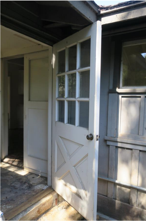
Service porch door, with altered (partially infilled) window opening to the right.
