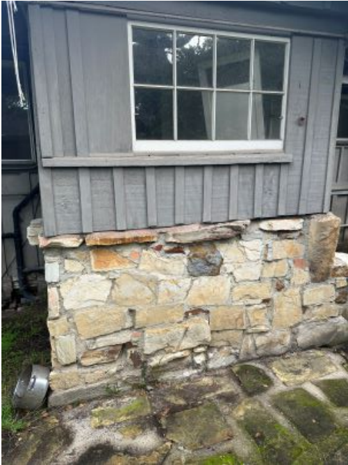
Figure 23 Masonry element at back of house
