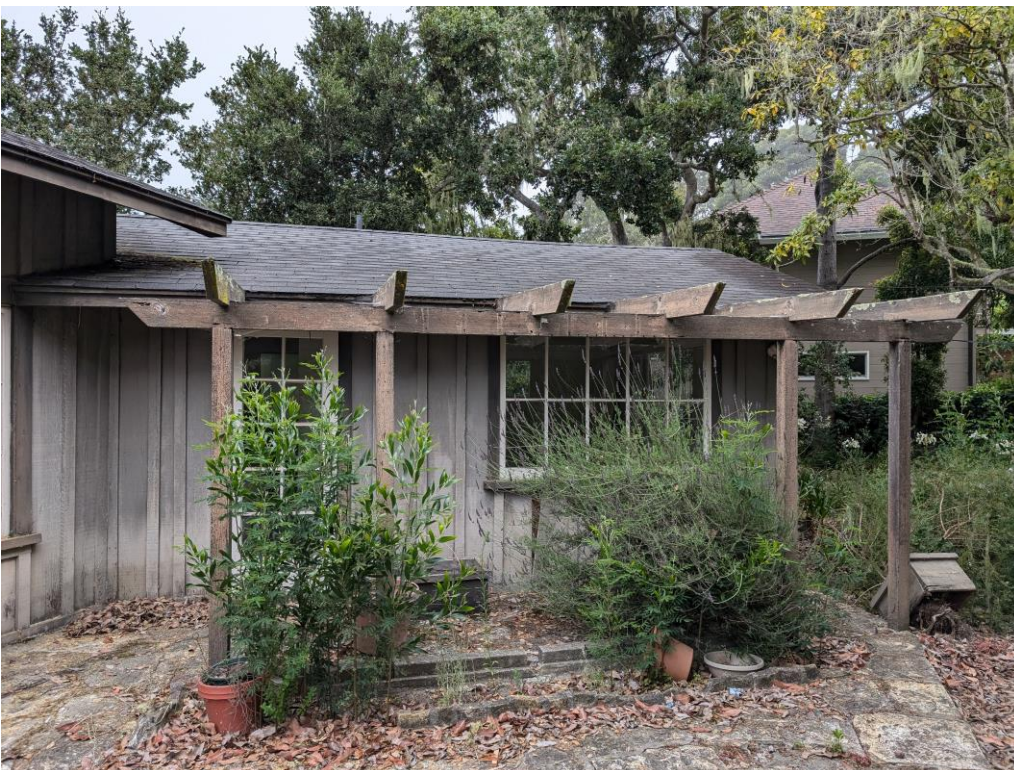
North wing, looking north. Window is fixed.
