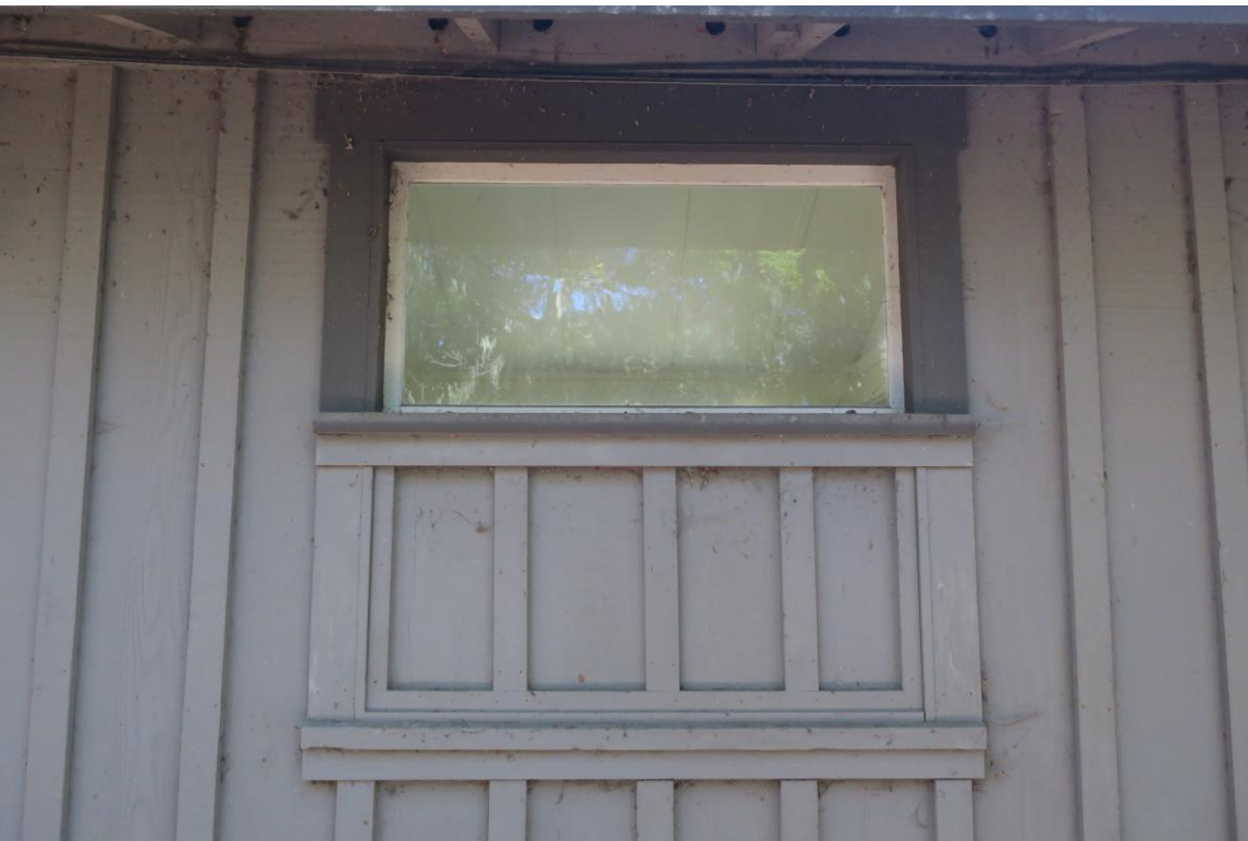
Detail of altered (partially infilled) window on the north wing.
