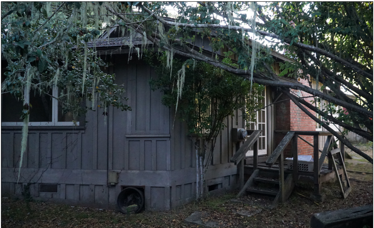
Figure 2. Looking southwest at north and east sides. The space at the corner of the two sides, where a window was formerly present, has been completely filled in with board-and-batten siding.
