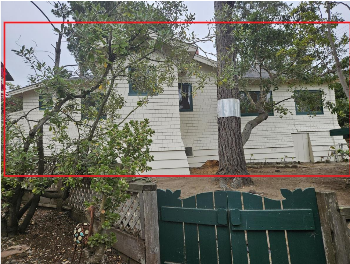
Figure 6: View of the west elevation with additions outlined in red.
