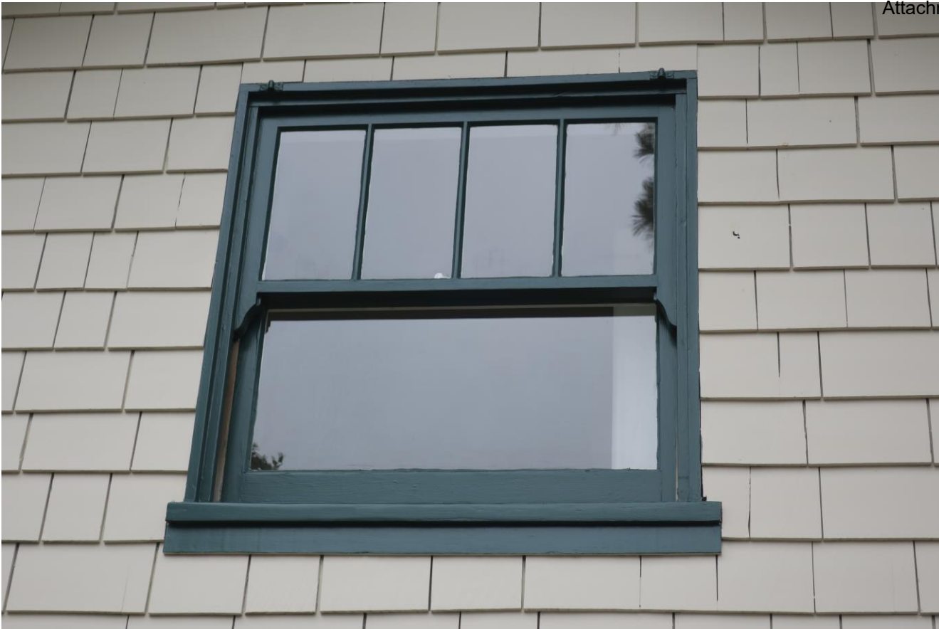
Typical window: Double-hung wood window with upper divided lights.
