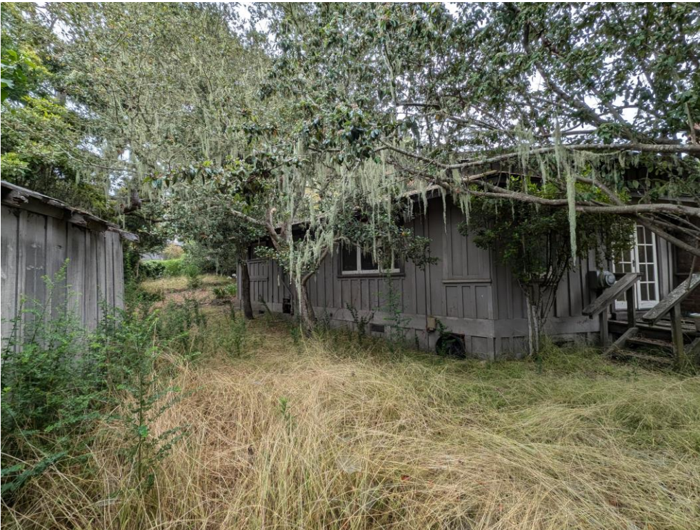
North wing, looking southeast. Note fully infilled window opening at corner. Note detached garage at image left.
