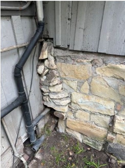
Figure 22 Masonry element at back of house
