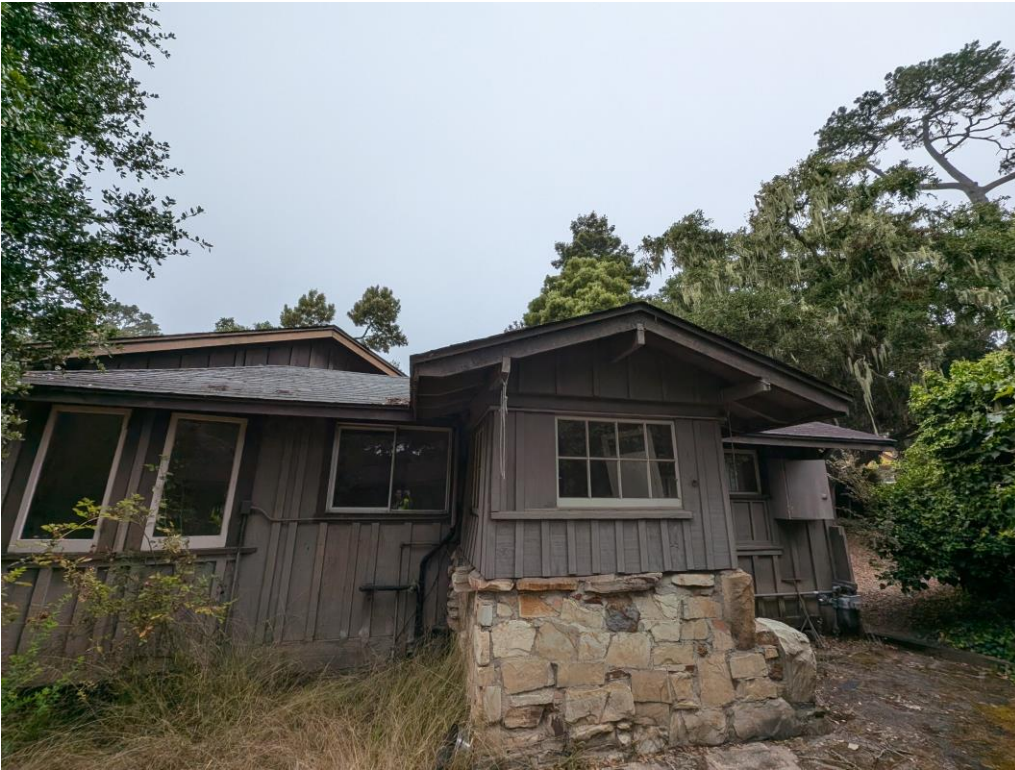
South wing with pentagonal bay at image left (with casement windows), and service porch with stone rubble base in foreground, looking northeast.
