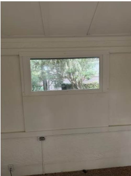
Figure 18 Stucco interior walls at modified window
