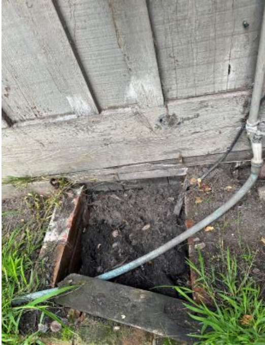
Figure 3 Top of foundation below grade
