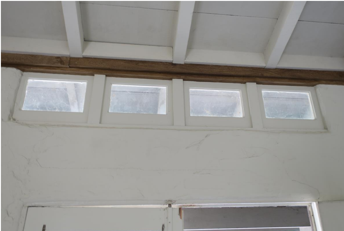
Detail of clerestory windows above front door, as viewed from inside.
