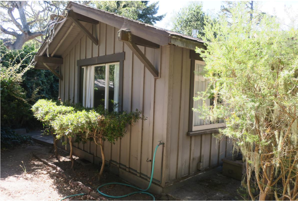
Detail photo of south wing eaves with brackets.
