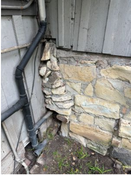
Figure 15 Surface run plumbing waste and gas lines
