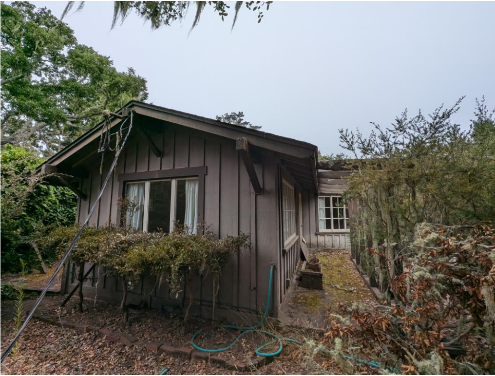
South wing, looking west. Tripartite slider in foreground.
