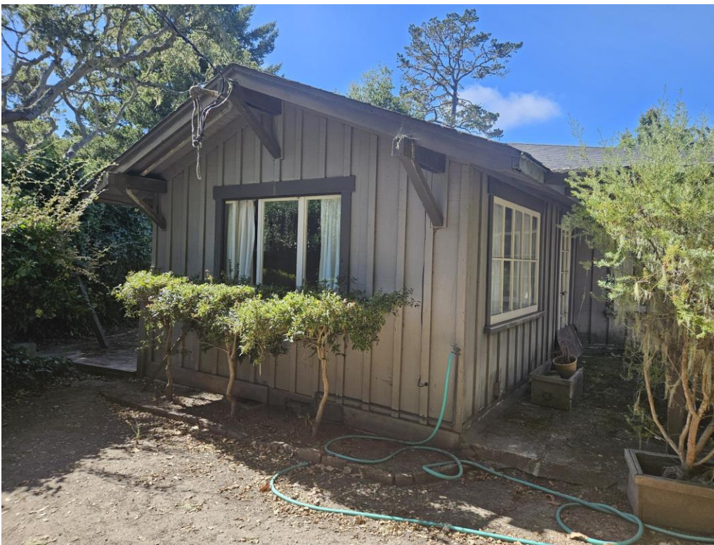
Figure 5: Knee brace brackets in south wing gable.
