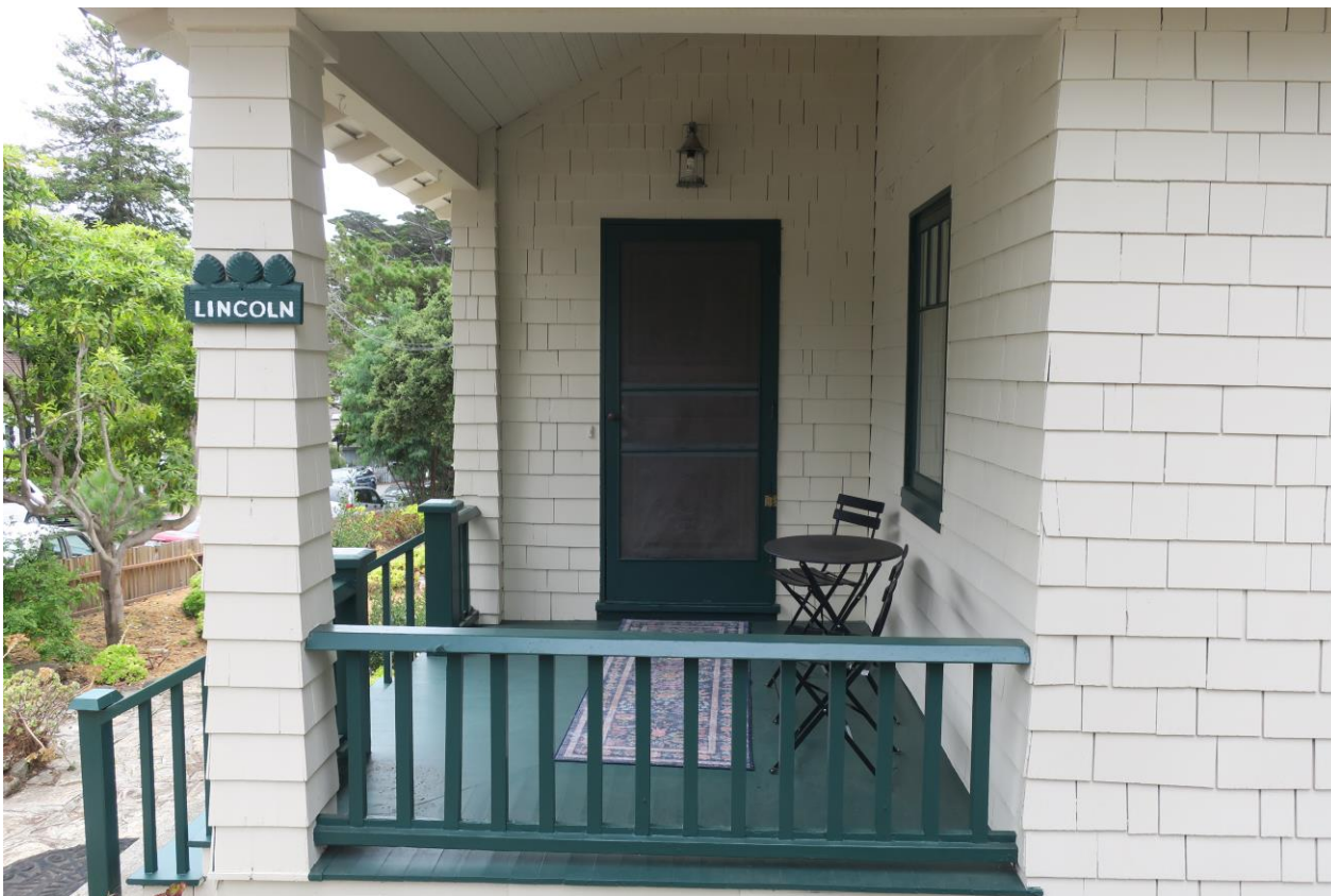
Front entry porch, looking west. Note the entry door was originally south-facing and was re-oriented to the east when the porch was partially infilled.
