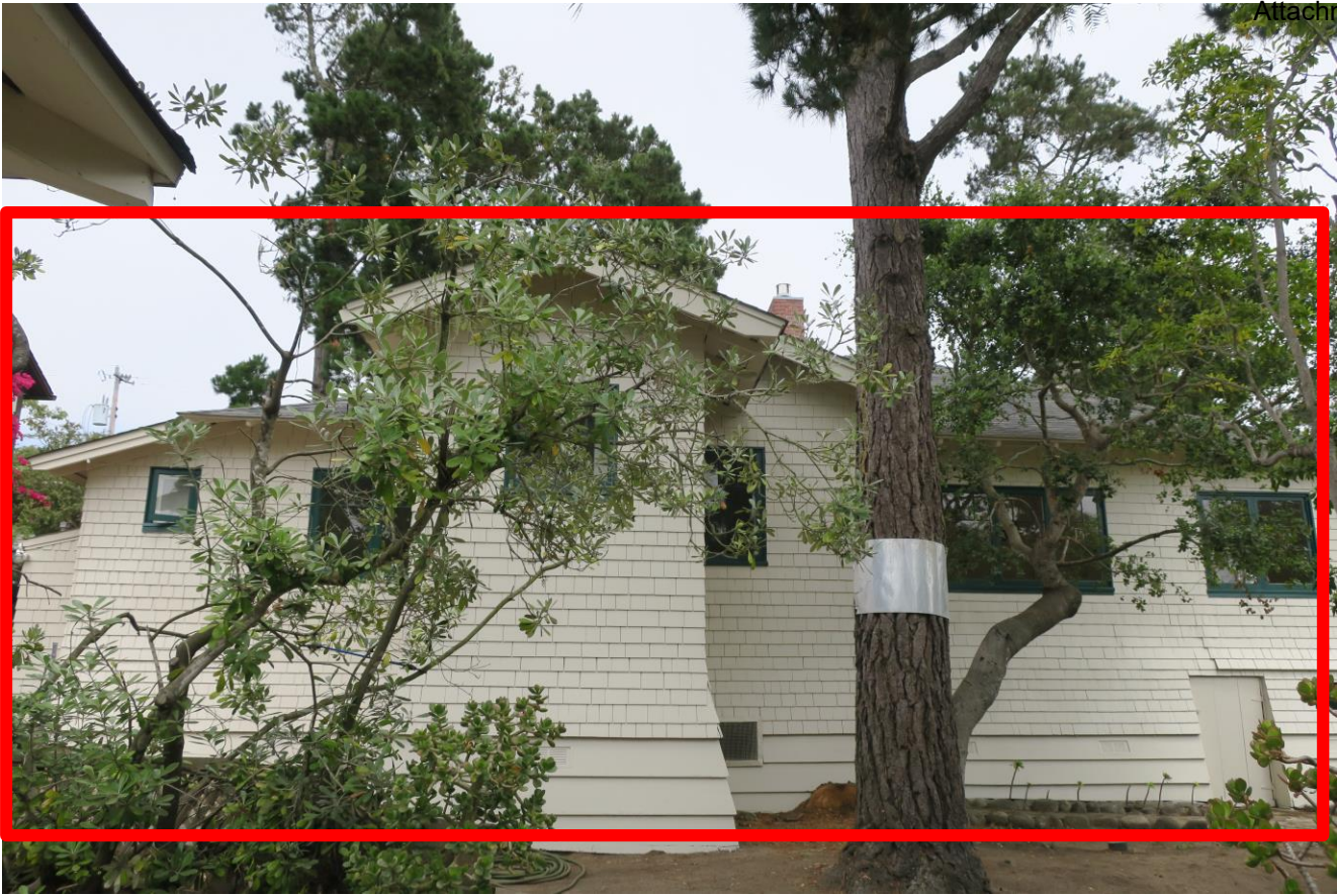
West elevation, looking east; red box indicating non-original volumes.
