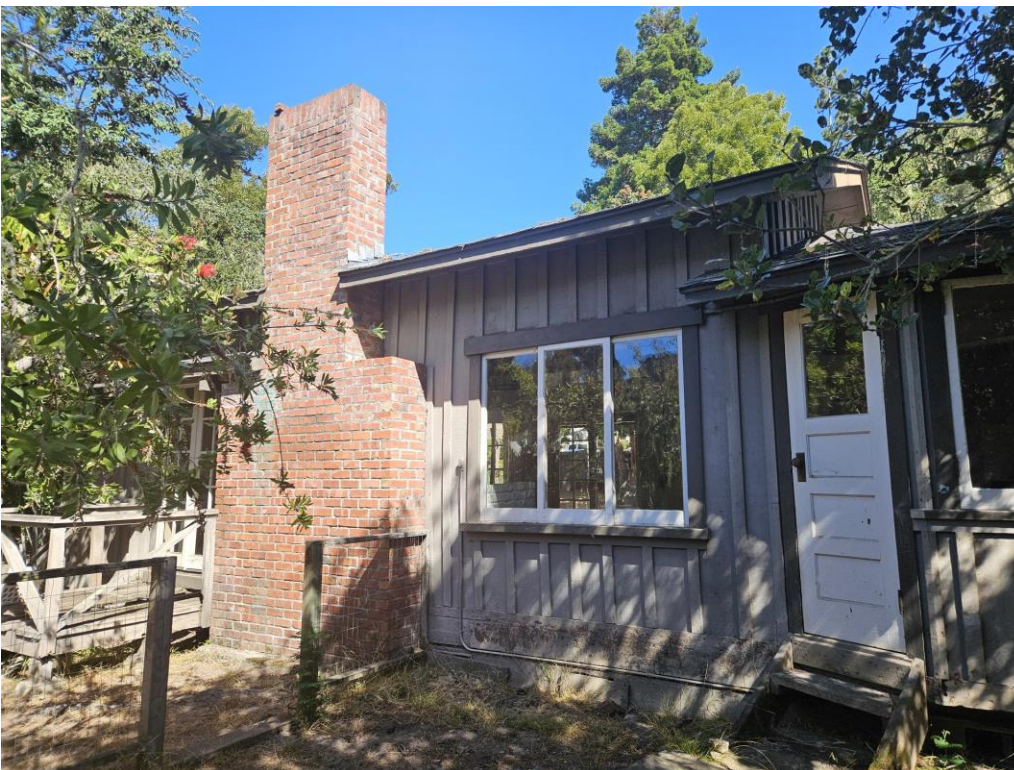
Figure 4: View of rear elevation looking northeast.
