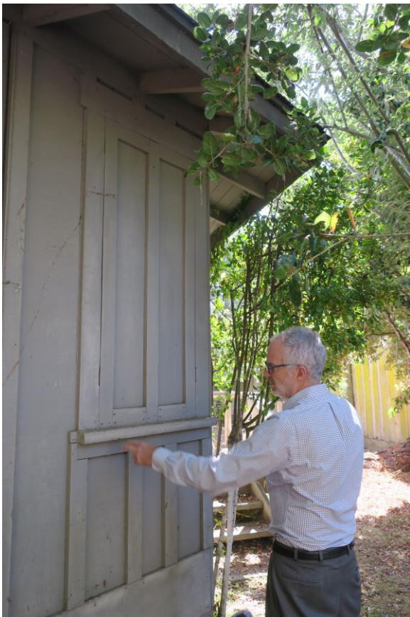
Detail of fully infilled window opening at the rear northwest corner of the house.
