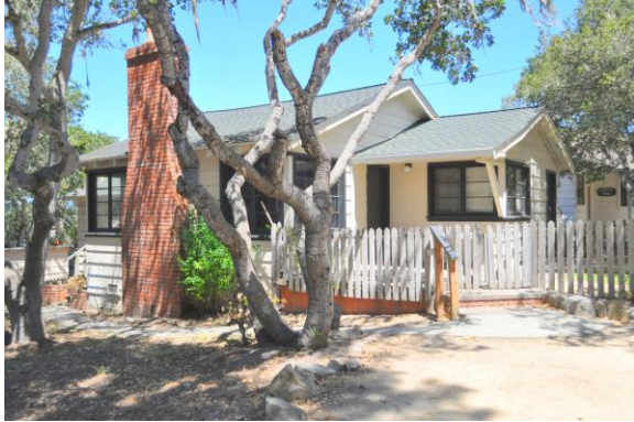
Minimal Traditional house (1935) at Guadalupe Street and Sixth Avenue.
