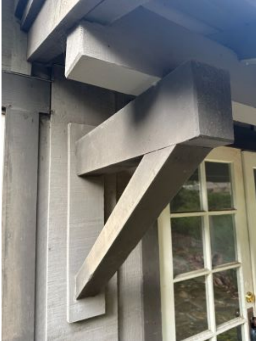
Figure 19 Knee brace at front entry
