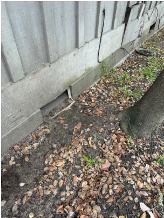
Figure 4 Foundation below grade
