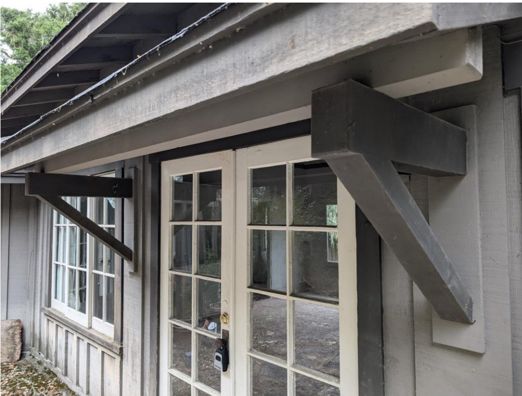
Detail photo of front entry door with narrow shed roof supported by brackets (newer looking).
