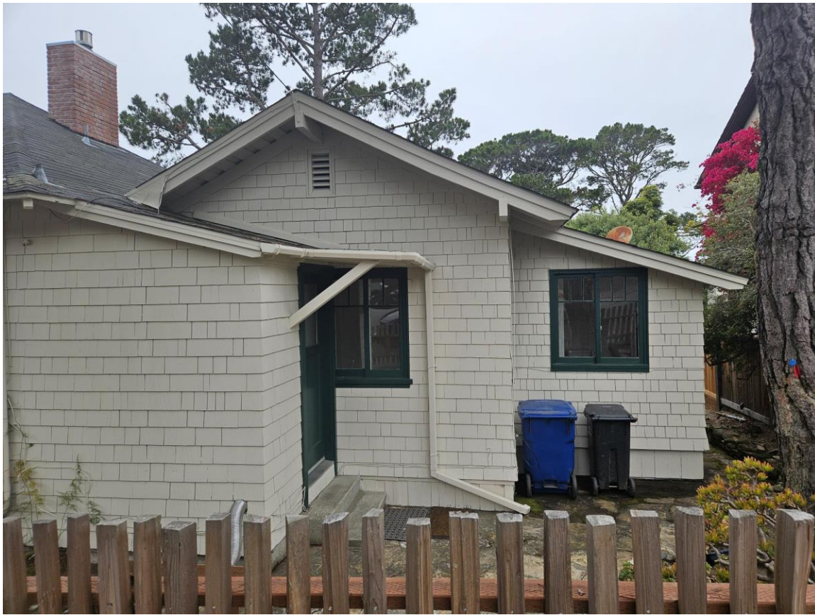
Additions at rear elevation, looking west.
