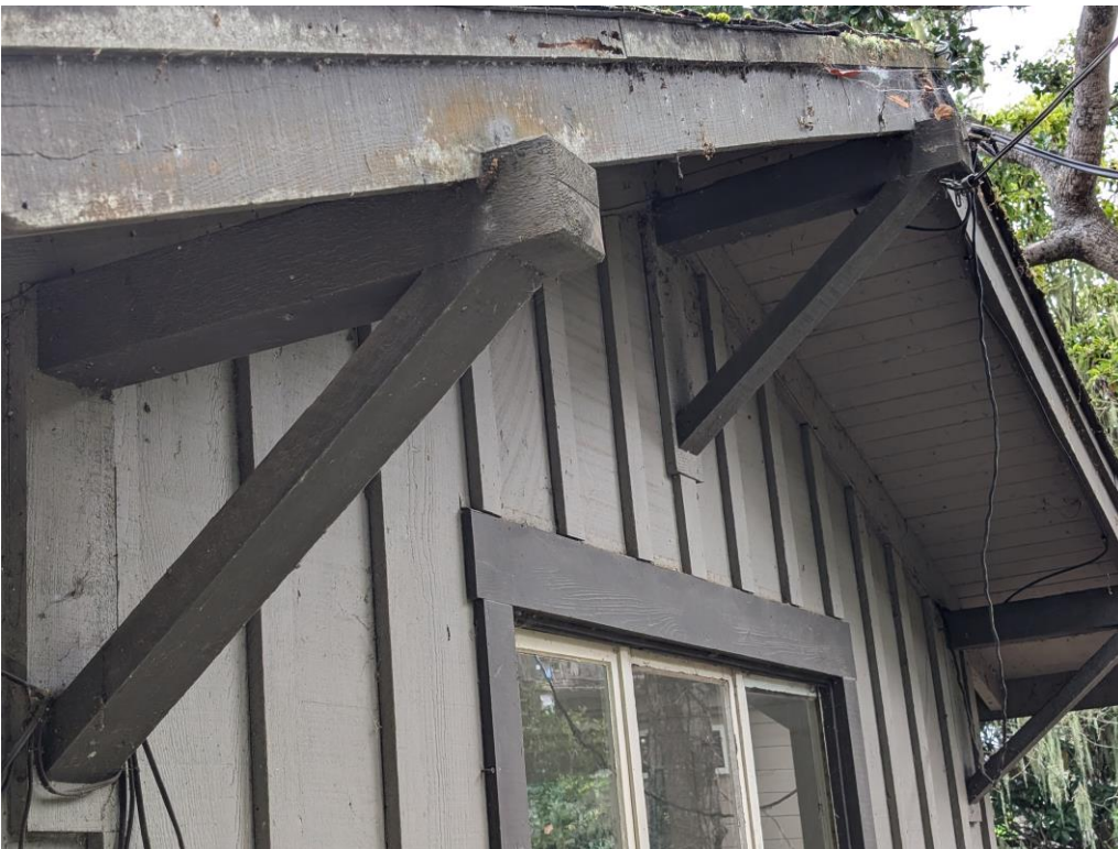
Detail photo of north wing eaves with brackets.
