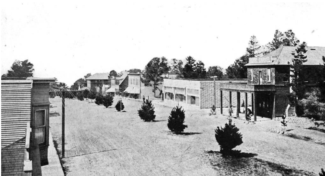
Circa-1910 image of the north side of Ocean Avenue, looking west. The Pine Inn can be seen at the far west end of Ocean Avenue. The one-story Carmel Development Company Building (extant) is at the center of the image, while the Carmel Hotel (demolished) is at image right (Source: Harrison Memorial Library).
