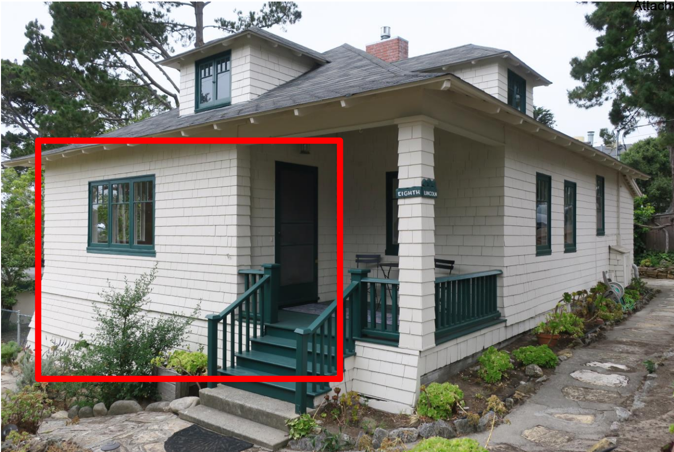
Subject property, looking northwest; red box indicating original front porch since infilled and altered with a new, re-oriented entry door.
