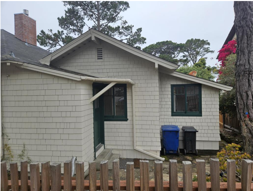
Figure 4: View of the cross-gable and shed roof additions, looking west from Lincoln (east elevation).
