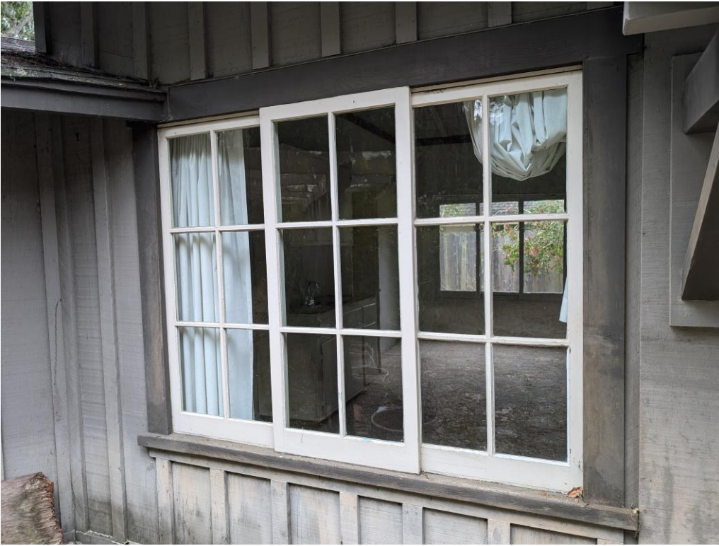
Detail of sliding windows at central volume, left (south) of front door.
