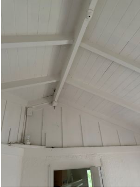
Figure 7 Bedroom with 2x6 ridge board and 2x4 rafters
