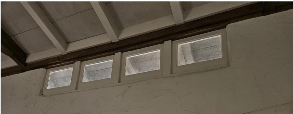
Figure 3: Interior view of fixed clerestory windows.
