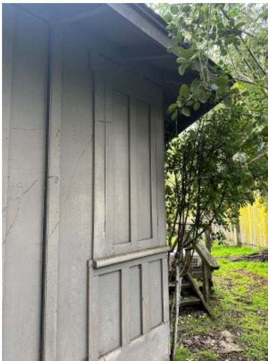
Figure 10 Former window filled in
