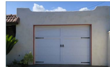
Existing (non-historic) garage doors on accessory structure
