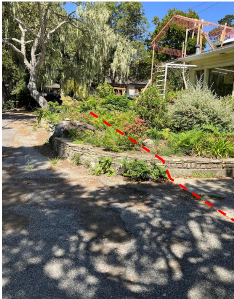
Figure 4b. Portion of subject existing encroachment. RED dashed line indicates approximate location of property line.
