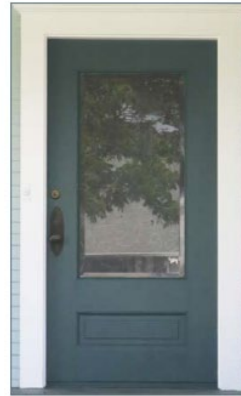
Paneled wood door with glazing
