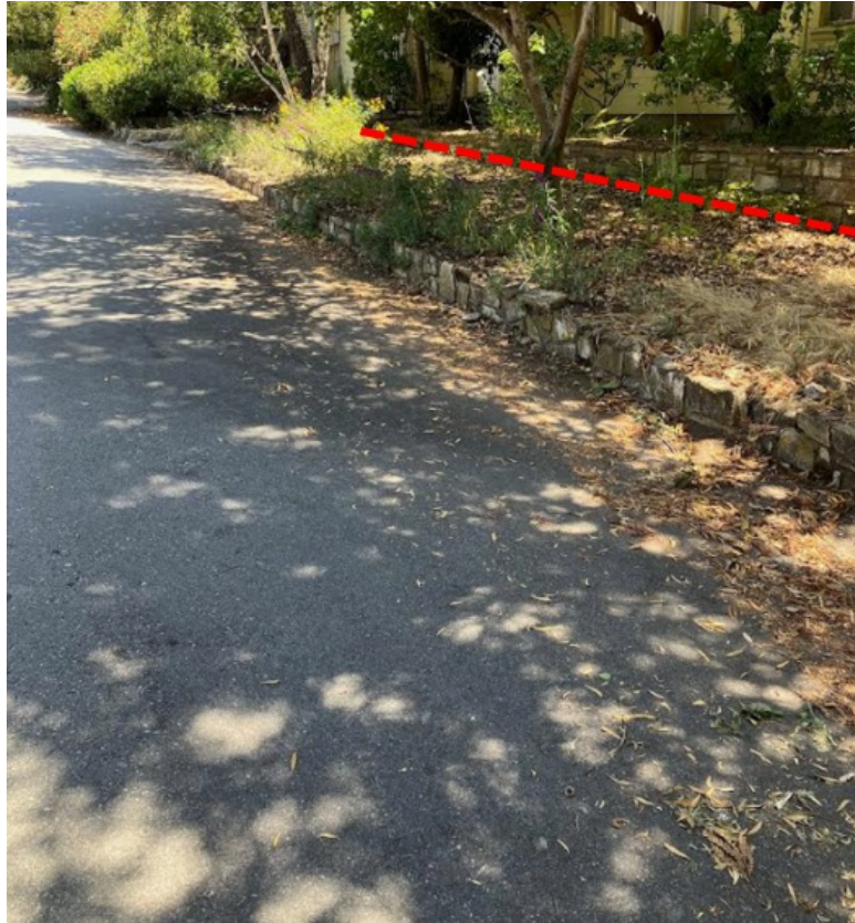
Figure 4d. Portion of subject existing encroachment. RED dashed line indicates approximate location of property line.
