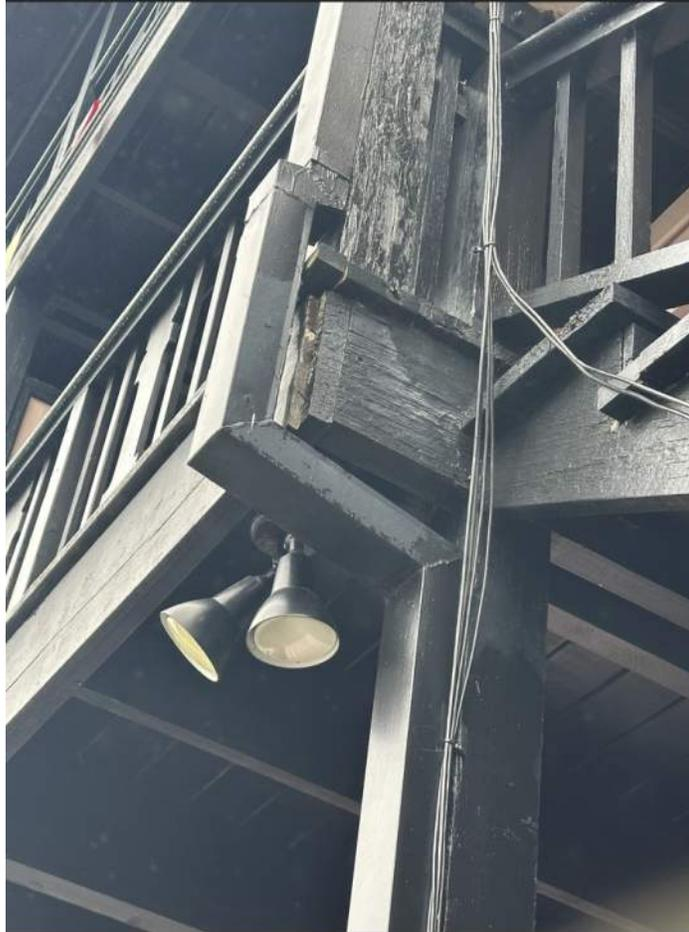
Figure 9- Example of Weathering in Exposed Framing
