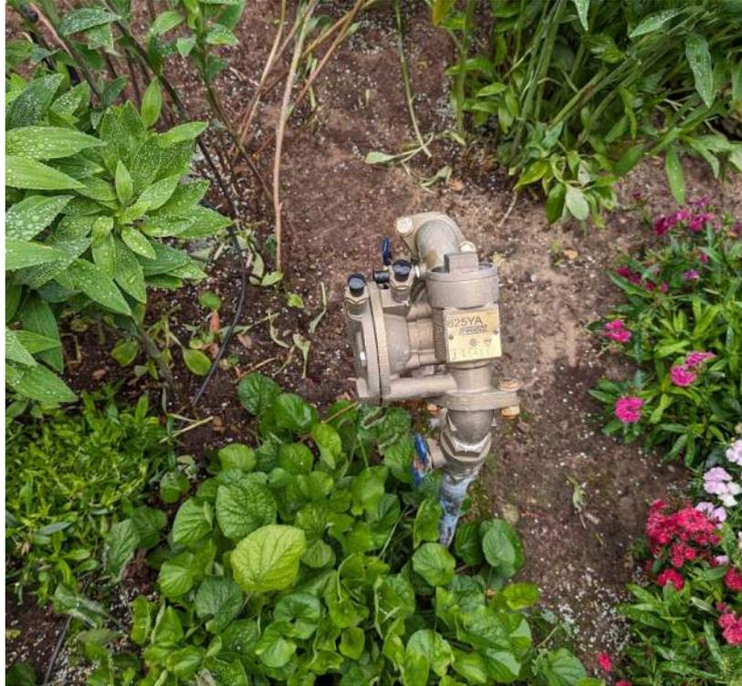
Figure 27 – Water Backflow Preventer
