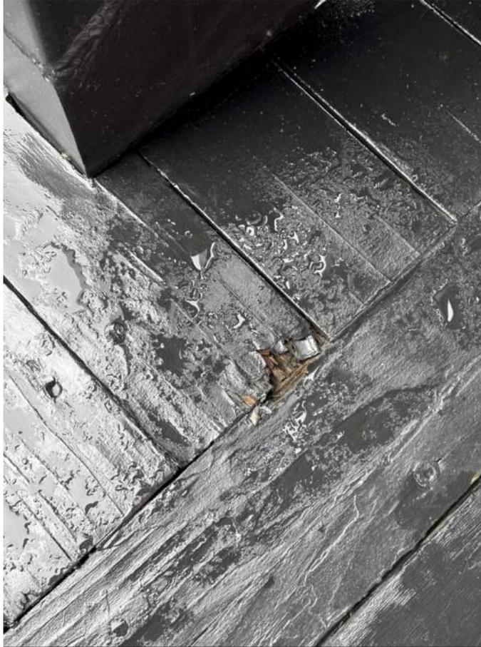
Figure 11- Dry Rot in Exposed Landing Framing at Northmost Building
