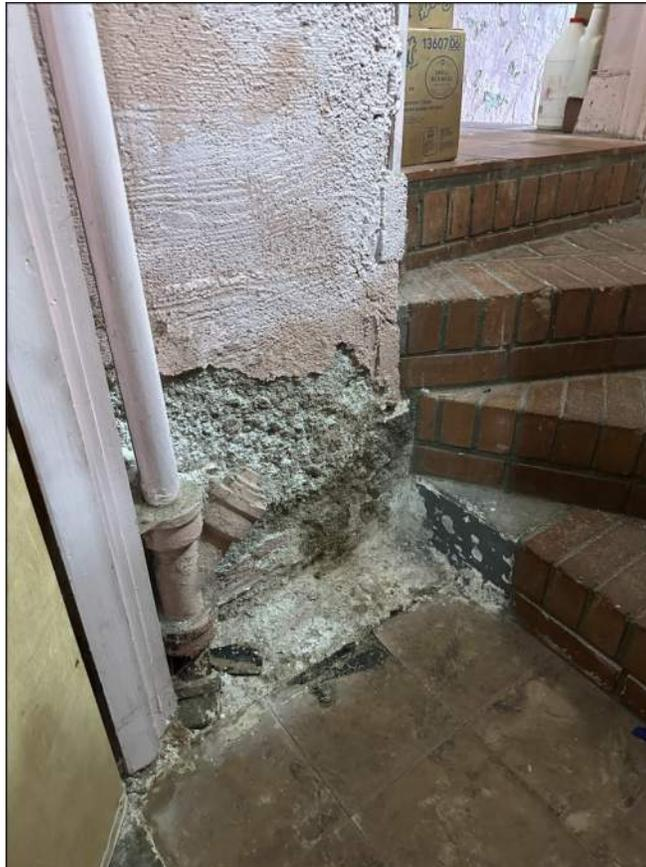
Figure 7- Additional Efflorescence and Weak Concrete in South Wall of Pre-1957 Structure
