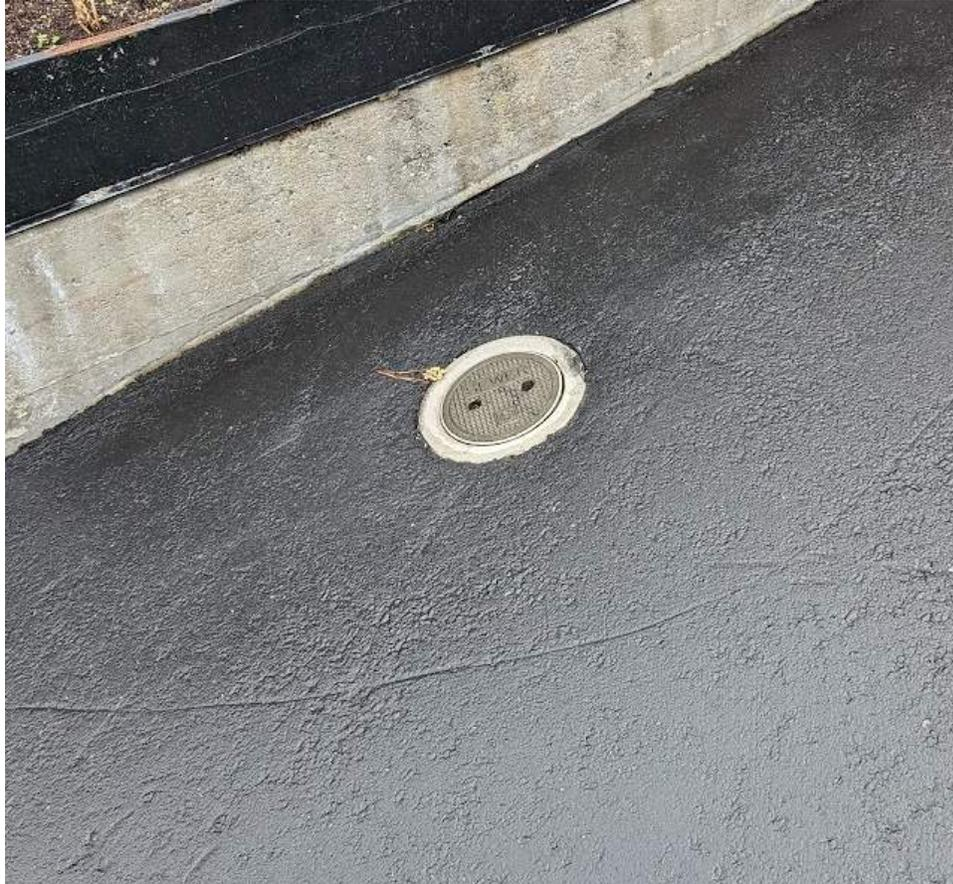
Figure 26 – Sanitary Sewer Cleanout
