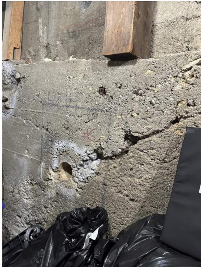
Figure 4- Void Vein in East Wall of Pre-1957 Structure
