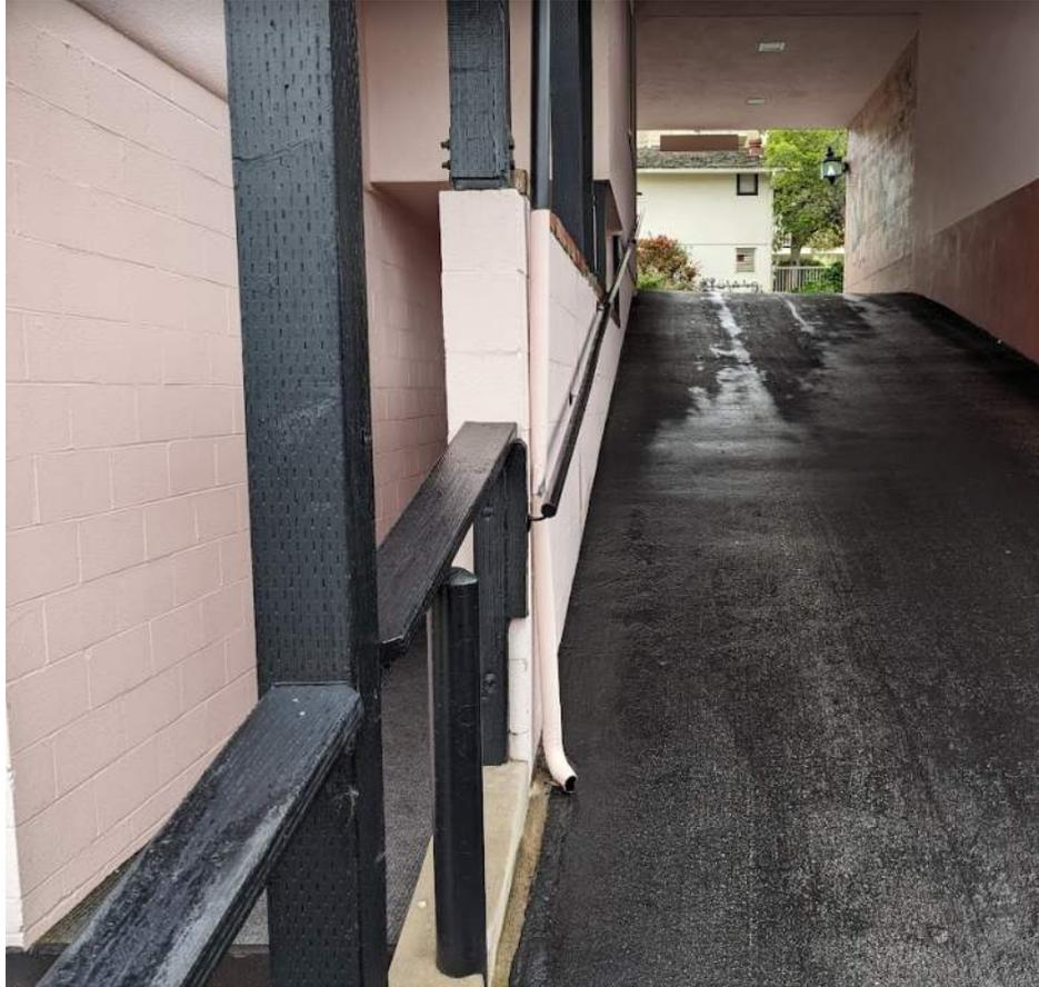
Figure 29 – Downspout onto Driveway
