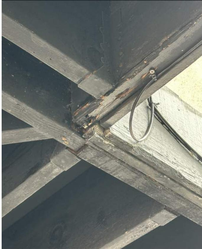
Figure 10- Dry Rot in Exposed Framing at Northmost Building
