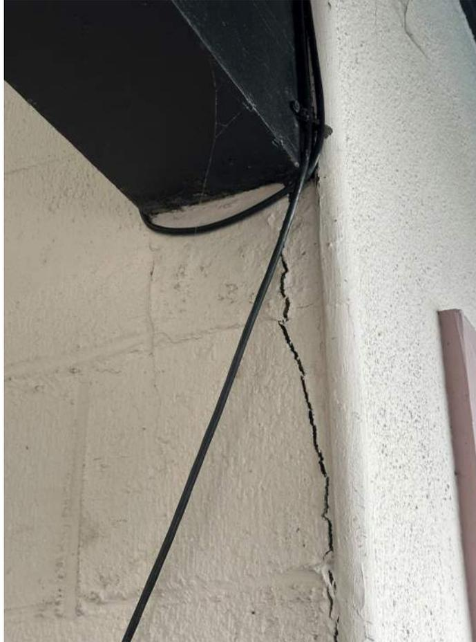
Figure 13- Fractured CMU Support Wall at Cantilevered 6x12
