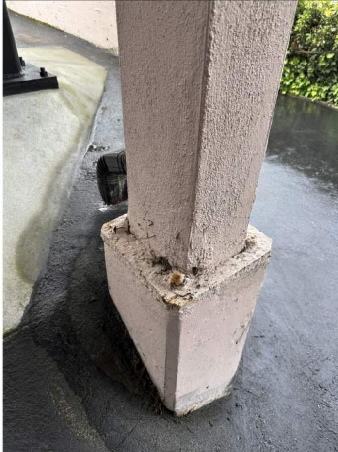
Figure 12- Corroded Base Plate and Anchors
