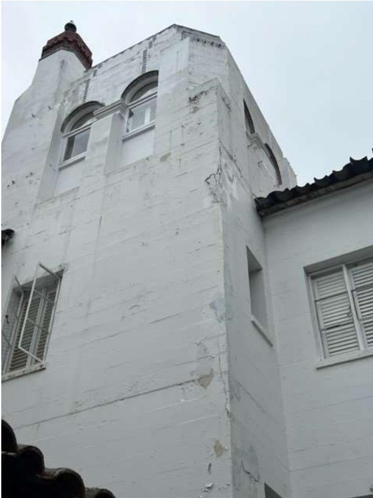
Photo #13, Concrete and plaster cracking as seen from Seventh Avenue courtyard
