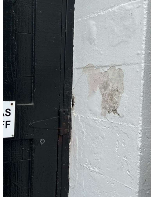
Photos #3-4, Plaster/paint damage at Lincoln Street service entrance
