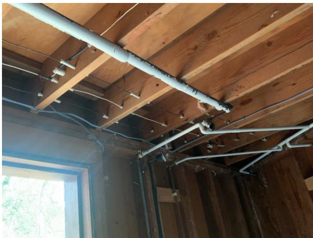
Knob and Tube Wiring
