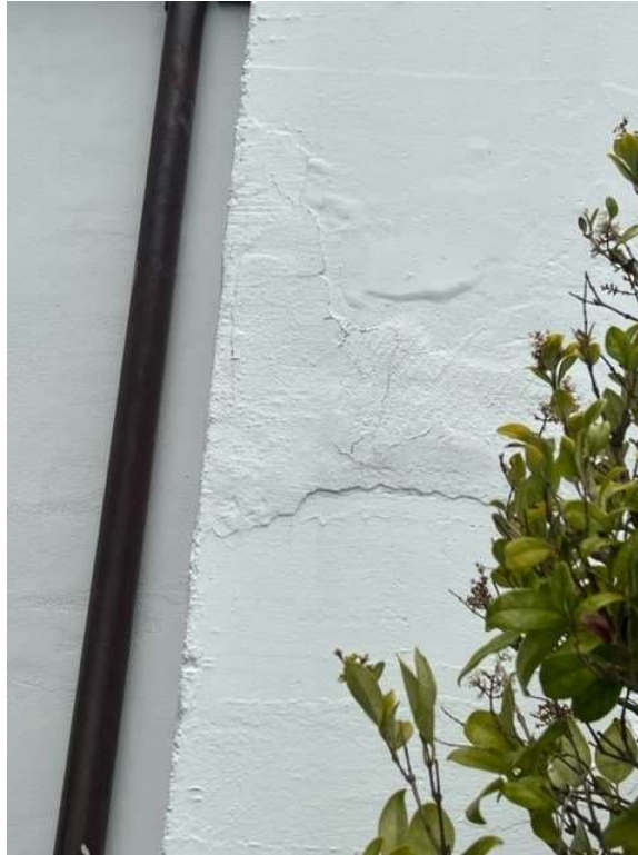
Photo #6, Patch over cracking plaster at Lincoln Street façade
