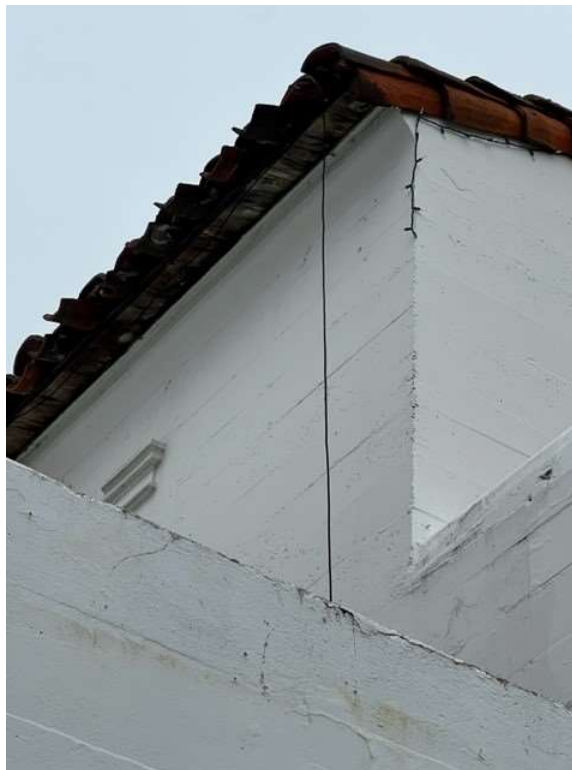
Photo #5, Typical deterioration of exposed wood at underside of eave (viewed from Lincoln Street)
