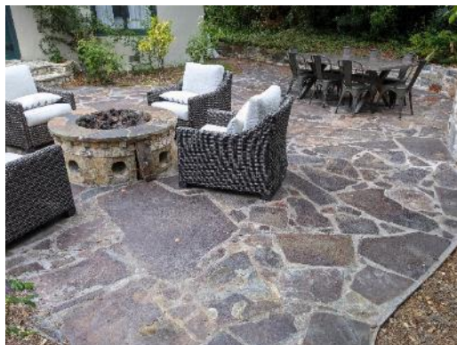
Patio stonework will be regraded to direct water away from the home.
