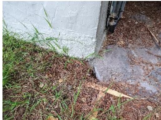
Drainage system to be installed by drainage contractor. Regrade hardscape to move water away from the house. This will address moisture in the crawl space.
