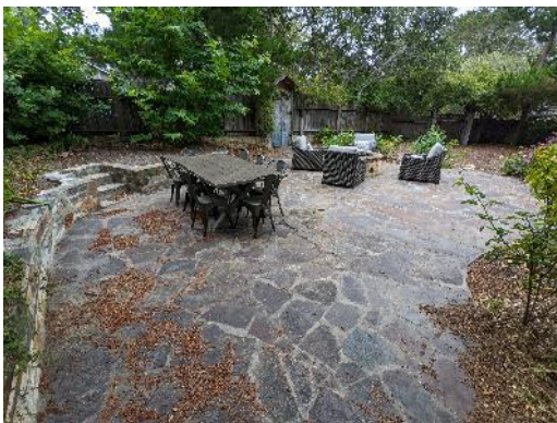
Patio stonework will be regraded to direct water away from the home.
