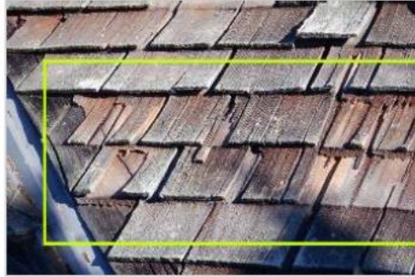
The main house roof is in disrepair; a new cedar shake roof is needed per the inspection report.
