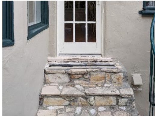
Broken landing and step stonework will be repaired.
