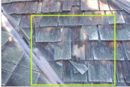
The main house roof is in disrepair; a new cedar shake roof is needed per the inspection report.
