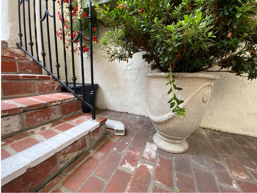
Photo 16, temporary surfact drainage at courtyard
