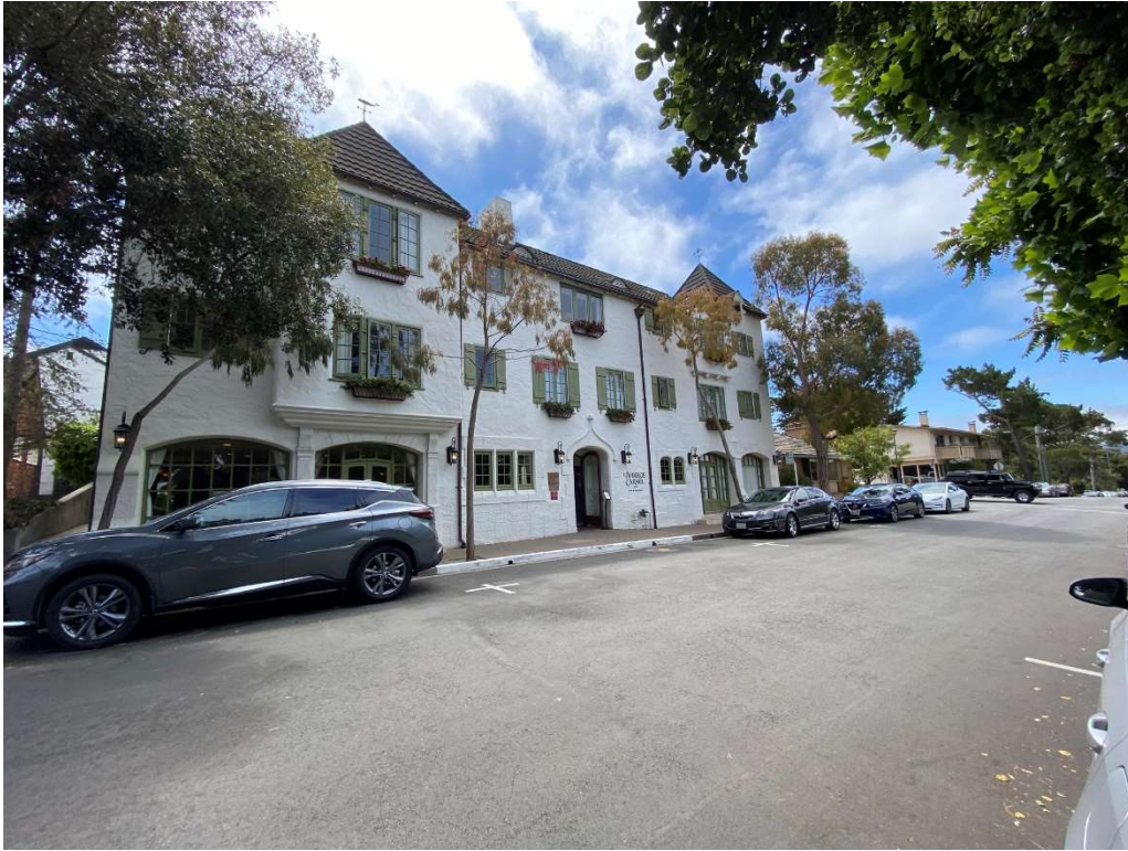
Photo #1, Main façade looking South along Monte Verde
