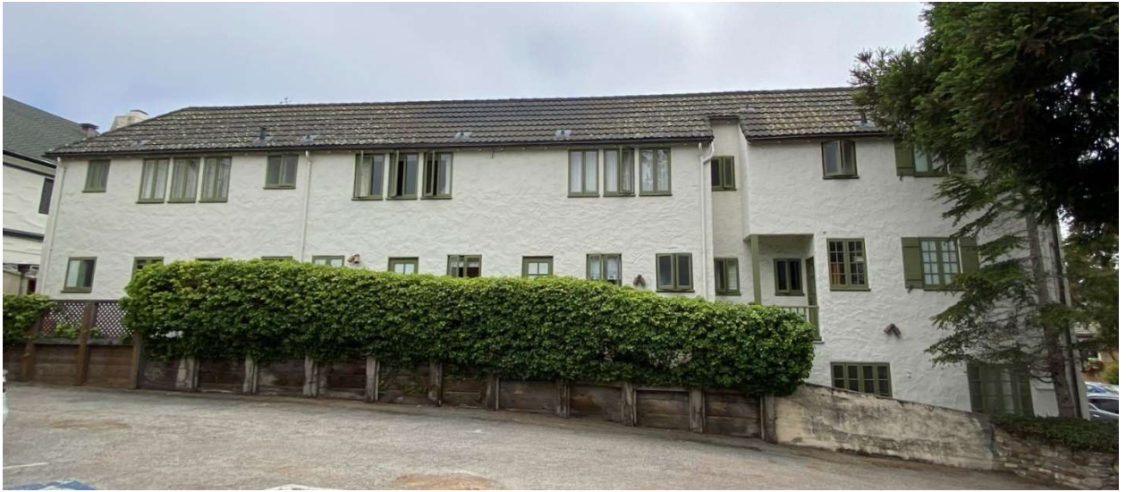
Photo #3, North elevation looking from City Hall parking lot
