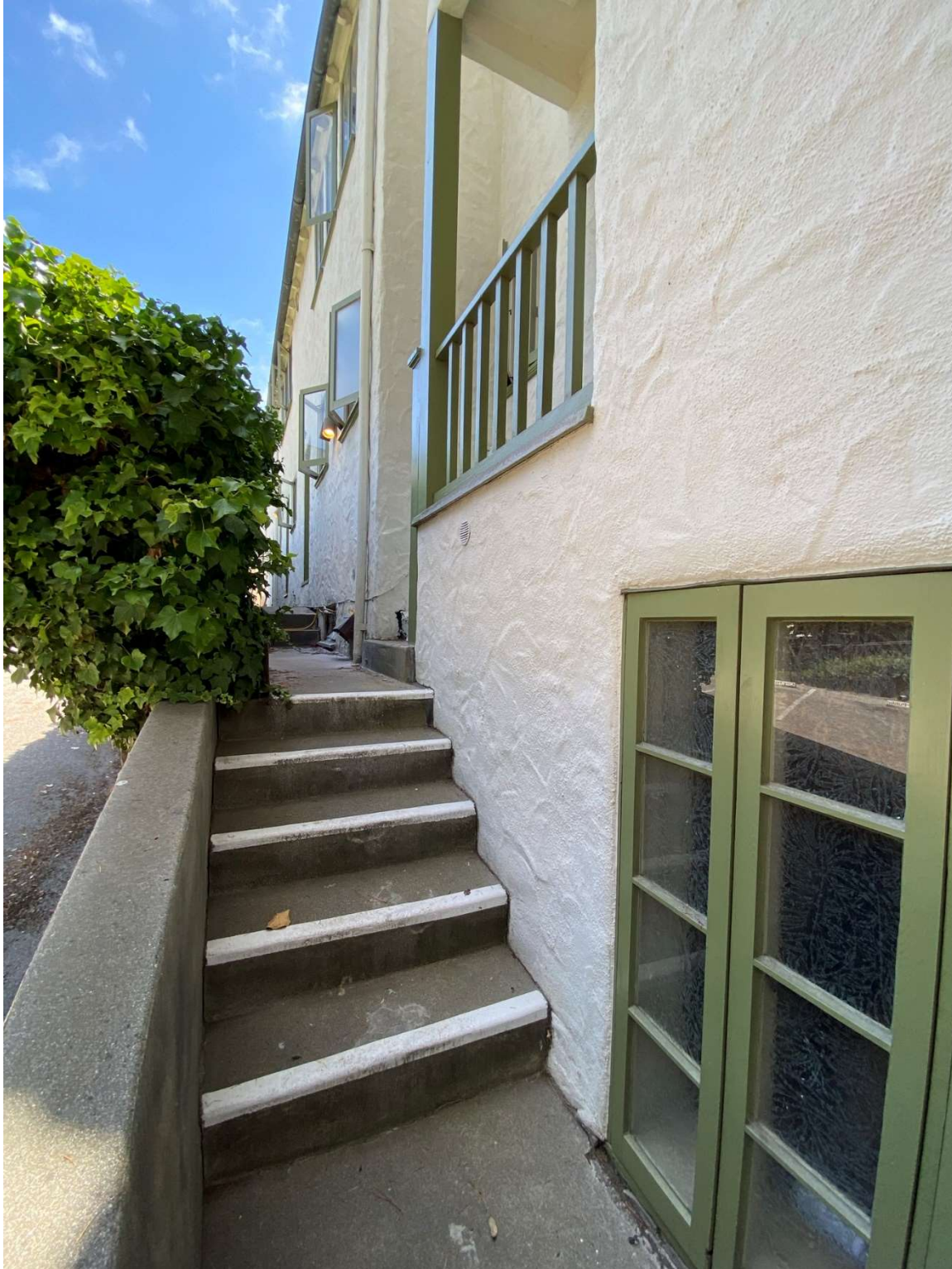
Photo 15, Existing retaining wall
