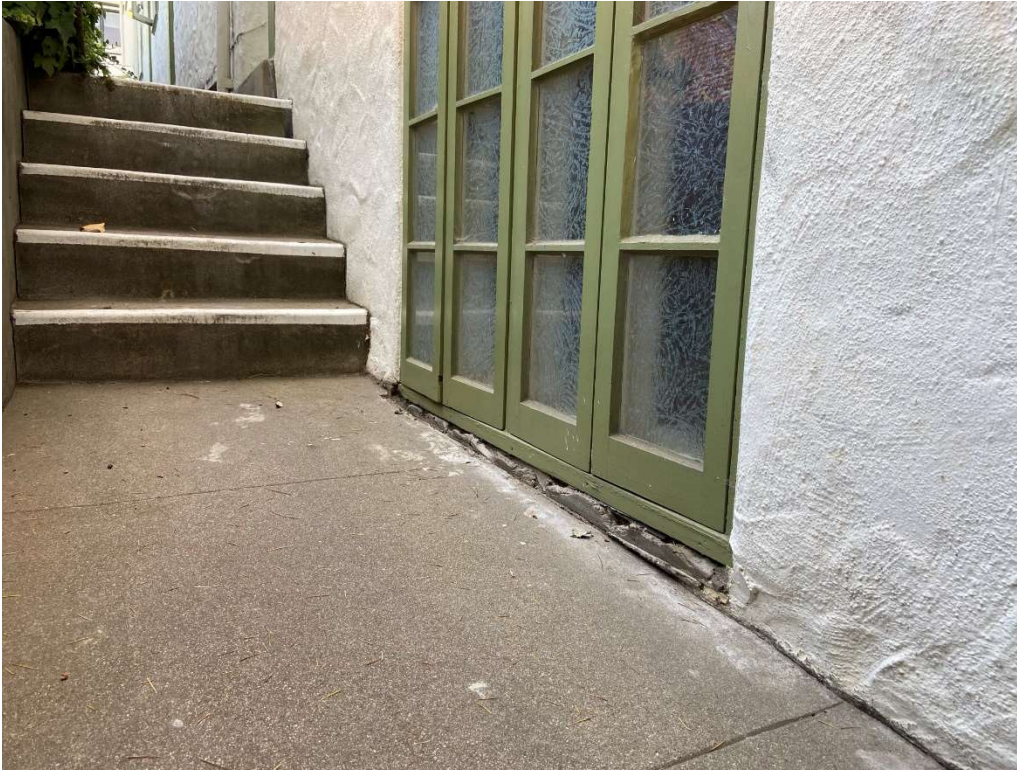
Photo #11 window sill at North side of building
