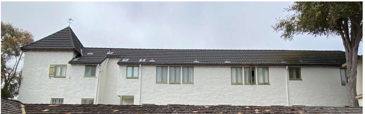
Photo #4, Partial South elevation looking from Seventh Avenue
