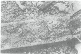
Fig. 6 d. View looking down towards the sill. The subframes appeared very rusted, but were in good condition once debris was vacuumed and surface rust was removed, in place, with chemical compounds. Where necessary, epoxy and steel filler was used to patch depressions in order to make the subframe serviceable again.
