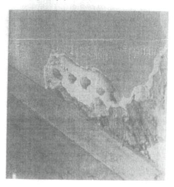
Fig. 4. The builders of this mid-18th century house installed the baseboard moulding first, then applied a mud and horse hair plaster (called paling) to the masonry wall. Line was used for the finish plaster. Also shown are the backing marks which prepared the wall for a subsequent layer of plaster. Photo: Kay Weeks
