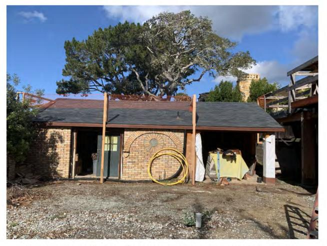
Photo 2. South elevation of existing garage. East portion to be converted to a pergola.
