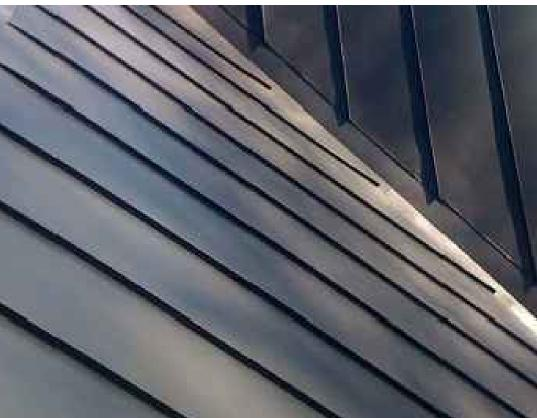
STANDING SEAM METAL ROOFING MANUFACTURER: CUSTOM-BUILT METALS COLOR: MIDNIGHT BRONZE CLASS A, SLOPED ROOF
