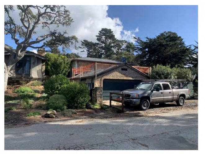
Photo 1. Existing gable roof on garage to be replaced with flat roof
