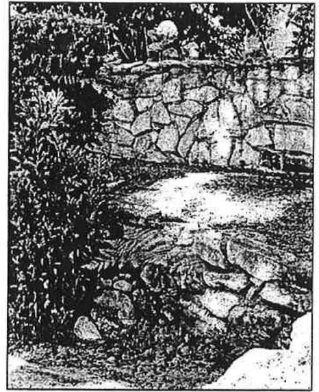
Each individual wall should not exceed four feet in height. Terrace or step walls on steeper slopes and locate plantings in front of each terrace when feasible.
