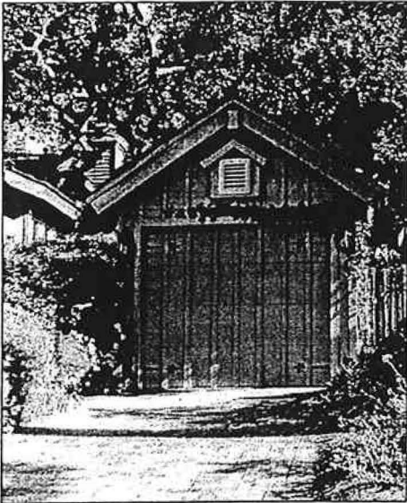
Preferred: This overhead door matches the board and batten siding of the garage itself.
