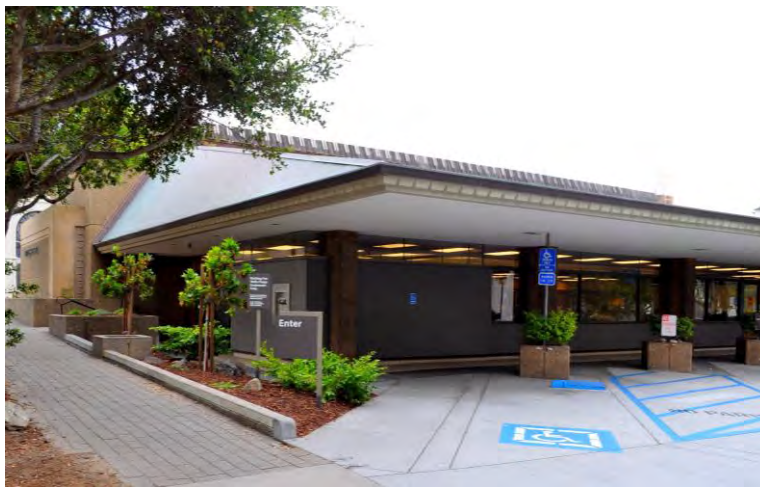
Wells Fargo Bank (1965) by Olof Dahlstrand on San Carlos Street, between Ocean and Seventh Avenues.
