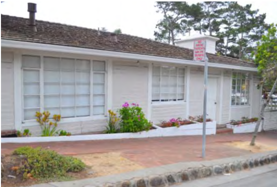
Carmel Village Inn (1954) by James Pruitt at NE Ocean and Junipero Avenues.
