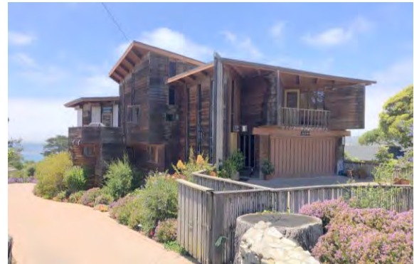
Golub House by Albert Henry Hill (1972) by Albert Henry Hill at San Antonio Street near Fourth Avenue.
