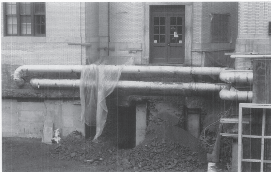
Figure 3. Concrete pier underpinning to an existing building may be necessary when adjacent construction occurs. In this example, pits are hand dug beneath the foundation of the historic building to provide space for wood forms. After concrete is poured into the forms, the space between the top of the pier and the bottom of the original foundation is packed with a quicksetting grout. The historic building owner should retain an independent engineer to ensure that the underpinning plan adequately protects the historic structure. Photo: Professor Arpad Horvath, Department of Civil and Environmental Engineering, University of California, Berkeley.
