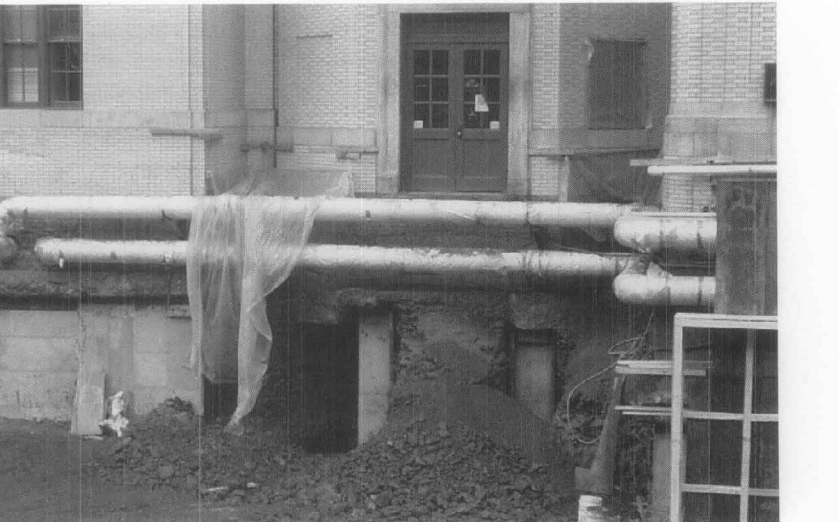
Figure 3. Concrete pier underpinning to an existing building may be necessary when adjacent construction occurs. In this example, piles are hand dug beneath the foundation of the historic building to provide a secure base for new columns. After the concrete is poured into the holes, the top of the pier and the bottom of the original foundation is packed with a quicksetting grout. The historic building owner should retain an independent engineer to ensure that the underpinning plan adequately protects the historic structure. Photo: Professor Arpad Horvath, Department of Civil and Environmental Engineering, University of California, Berkeley.
