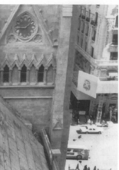
Figure 4. Dropped equipment, tools, and material all present risks when new construction rises above neighboring historic structures. In this case, the historic slate roof was completely covered with sheets of exterior grade plywood. Photo: National Park Service files.
