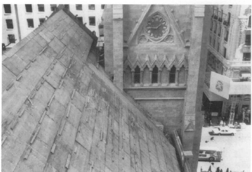
Figure 4. Dropped equipment, tools, and material all present risks when new construction rises above neighboring historic structures. In this case, the historic slate roof was completely covered with sheets of exterior grade plywood. Photo: National Park Service files.
