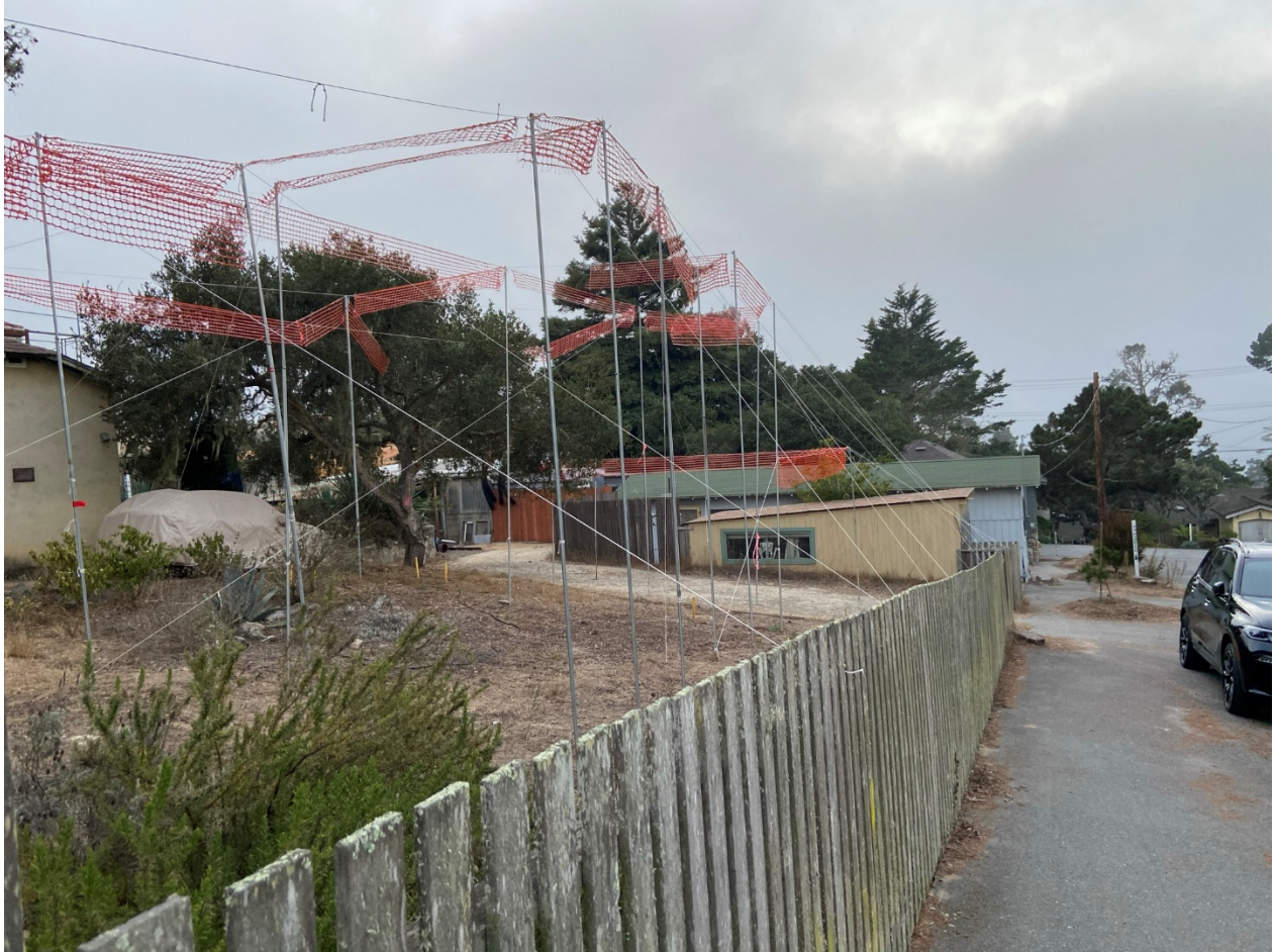
Figure 2. Southeast Elevation from 5 th Avenue
