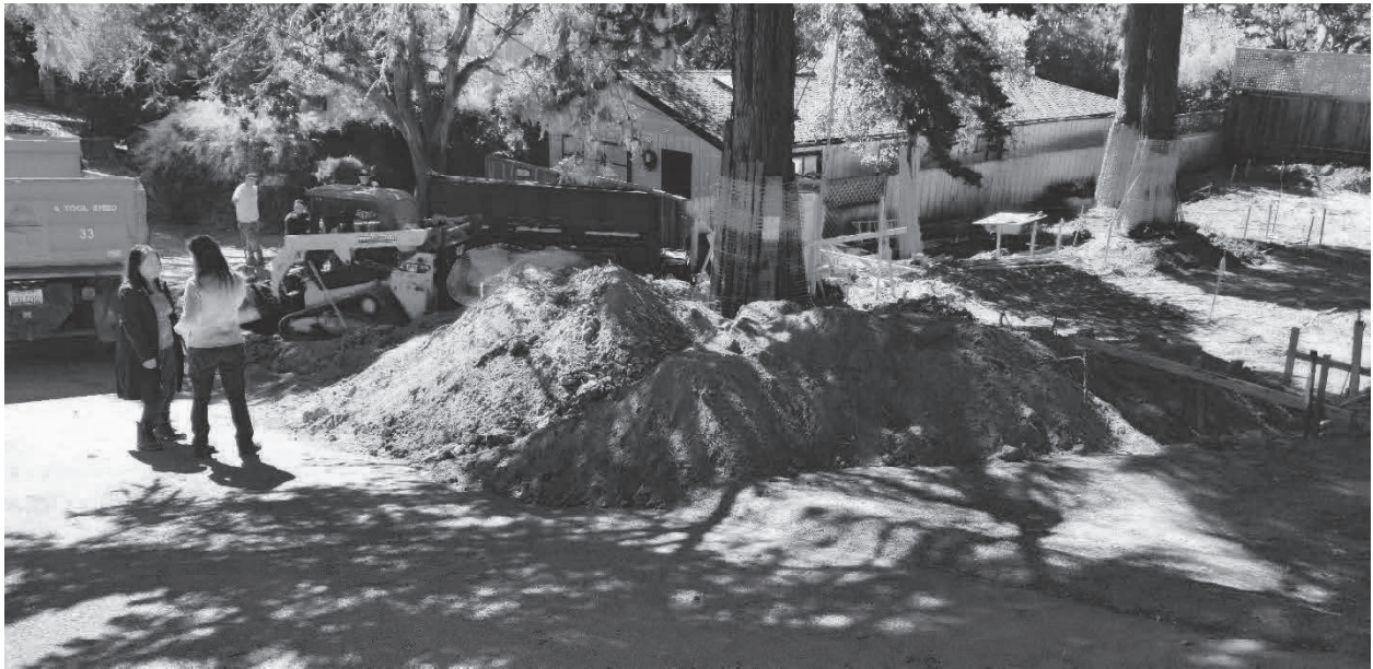
Figure 4: Looking southwest from street, note large pile of soil.
