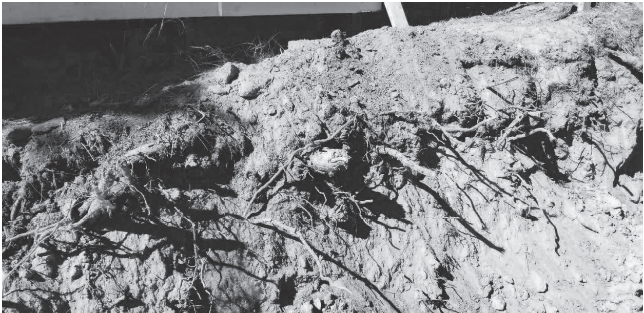
Figure 8: Roots seen on southern wall ripped rather than cut cleanly.
