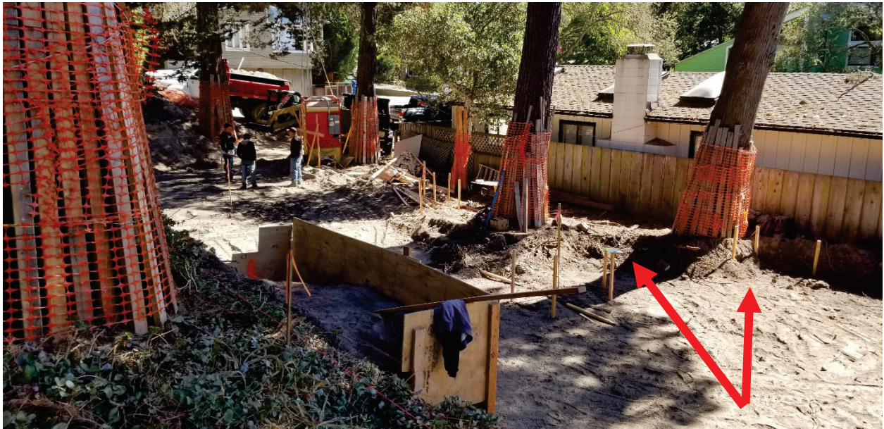
Figure 5: Looking southeast from Tree #7, red arrows note how close excavation was preformed near trees 4 and 5.
