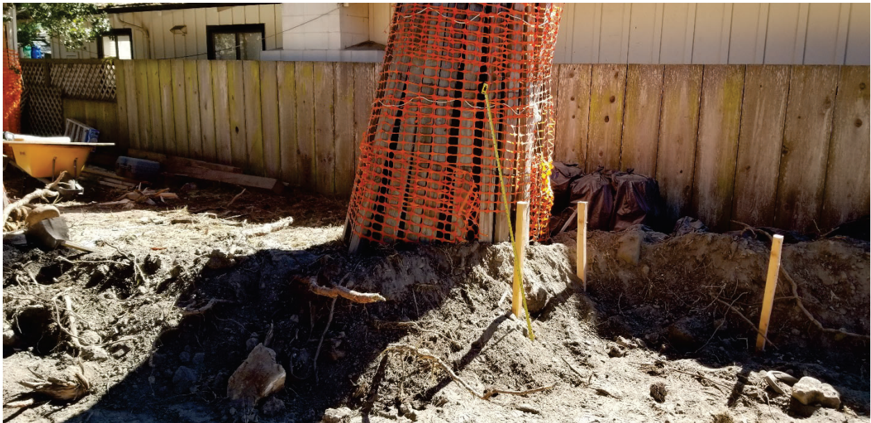
Figure 6: Looking south at Tree #5, Note roots ripped from ground with in 1-foot of trunk.
