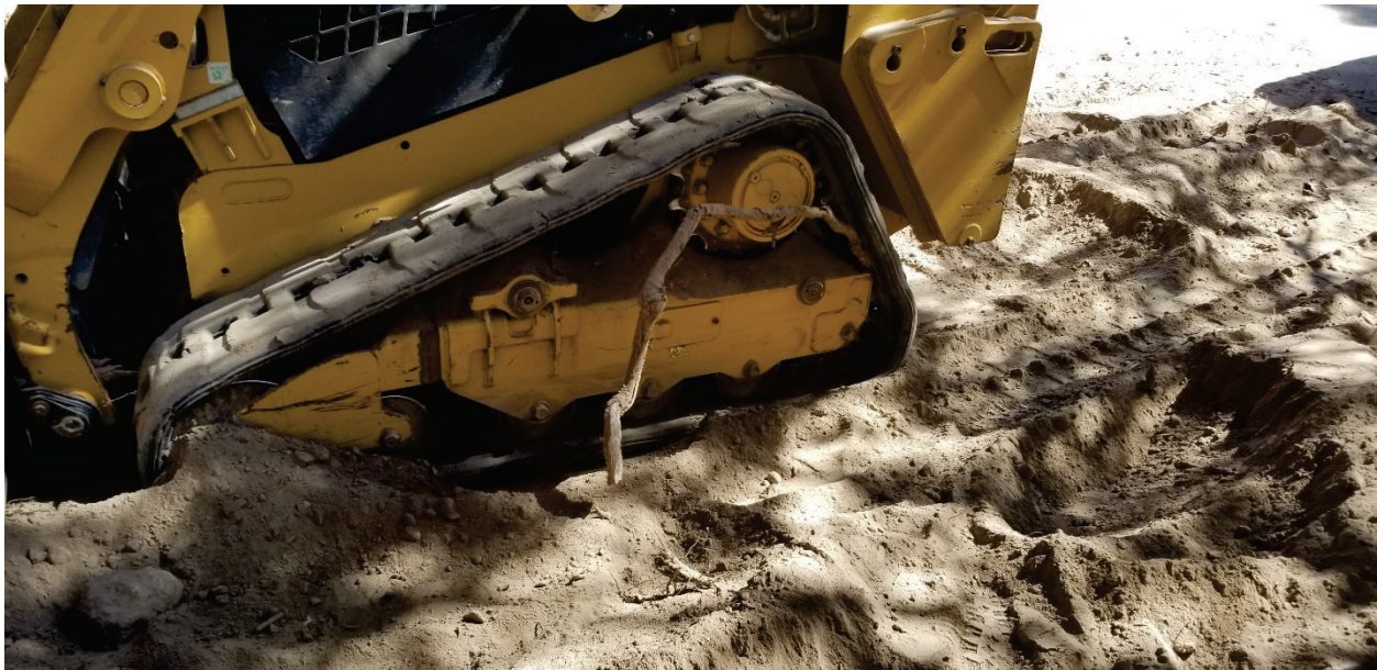
Figure 7: Skid-steer loader operating on site, note roots stuck in tracks an indication that little to no caution of roots was taken during excavation.
