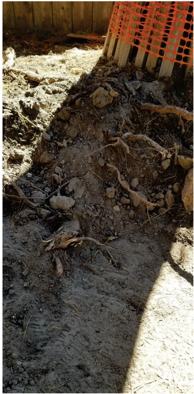
Figure 10: Torn remnants of roots with in 1-foot of trunk.
