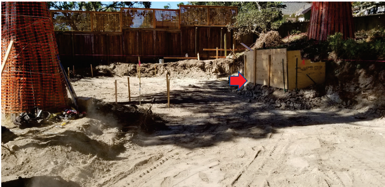
Figure 3: Looking west inside excavation area, red arrow shows box that was constructed around exposed roots of tree #7.
