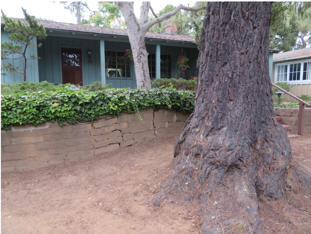
Photo 3. Four-foot diameter Monterey pine tree showing retaining wall damage
