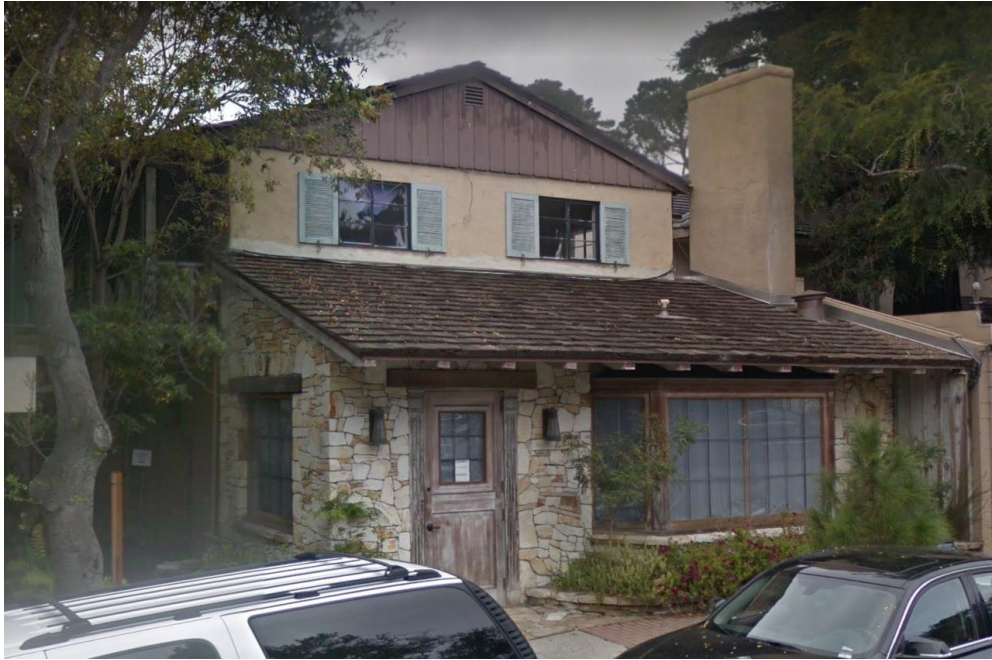
Front East Elevation of Gypsy Moon Café Fronting on Mission Street
