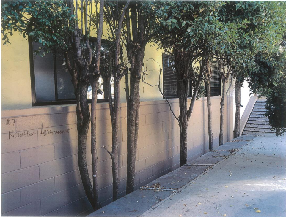
View from the top of the Glass Roof Toward the 2 nd -Floor Residential Apartments to the South of Outdoor Patio #1
