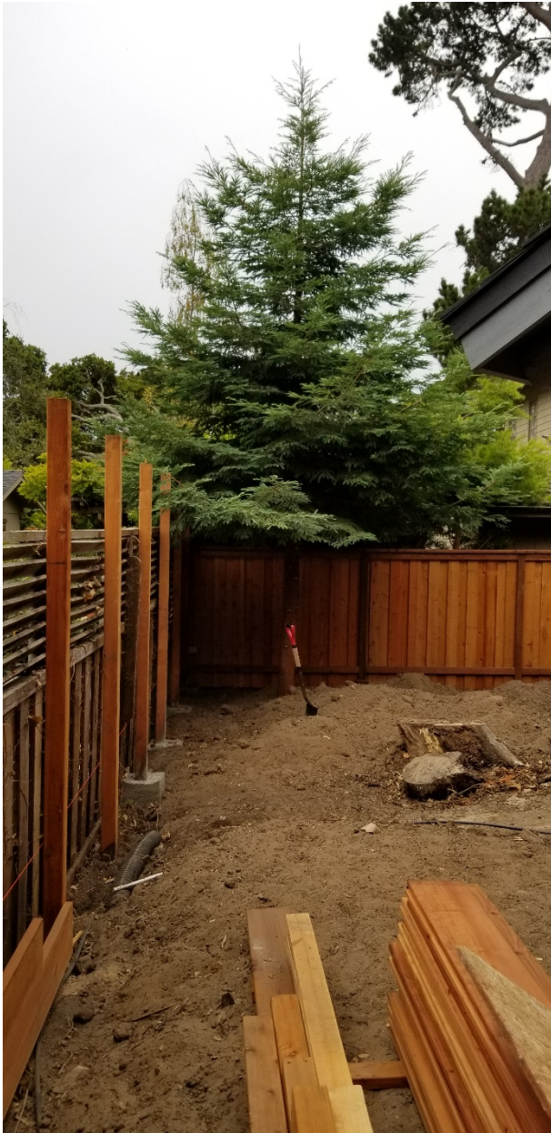
Figure 9: Tree-6 seen looking west, note soil deposited on root system.
