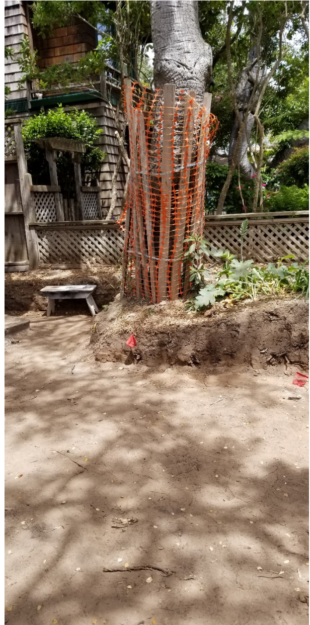
Figure 2: Excavation shown around tree 1, approximately 75% of the root zone was removed to a depth of almost 2-feet.
