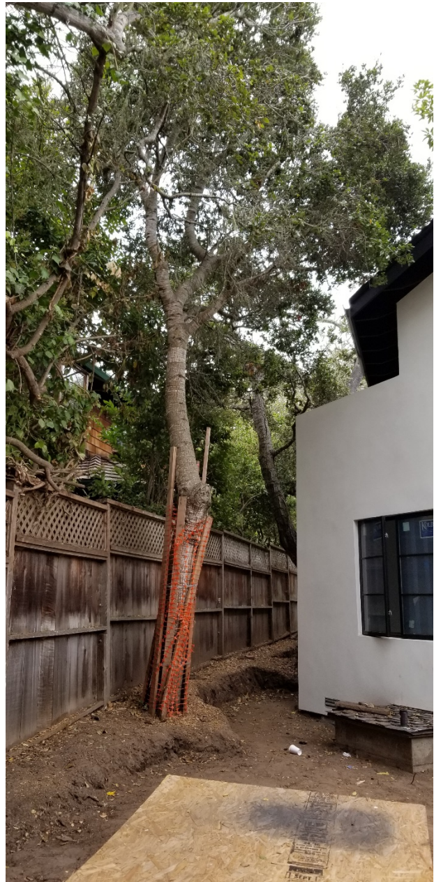
Figure 14: Tree-11 seen looking east, note 50% of root system removed to a depth of almost 2-feet.
