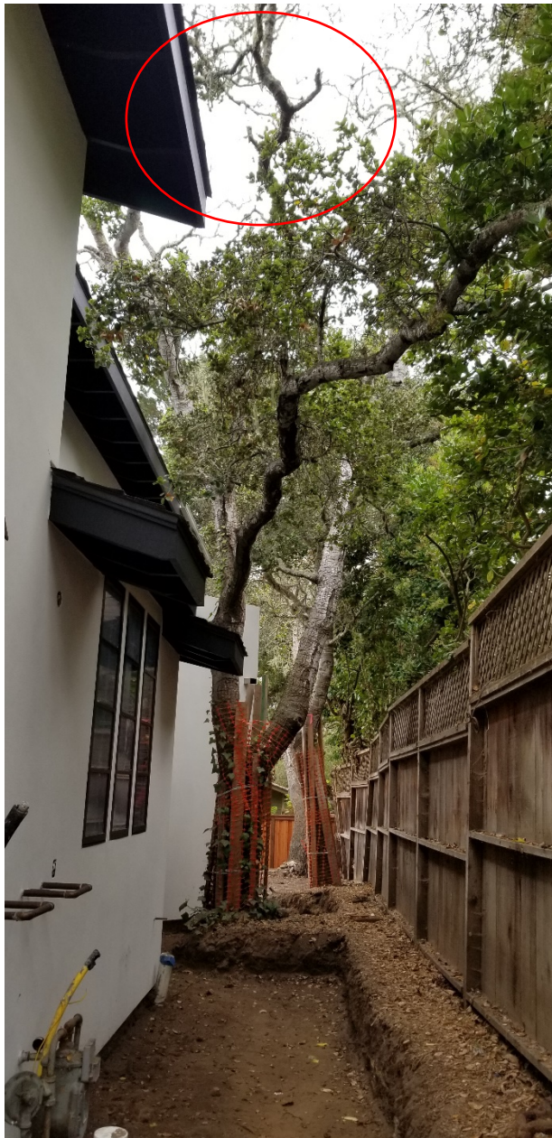
Figure 15: Tree-12 seen looking west. Decline in canopy noted by red circle. 75% of root system can be seen removed to a depth of almost 2-feet.
