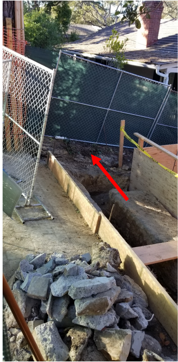
Figure 3: Excavation near west side of tree. red arrow indicates the location of the large buttress root.
