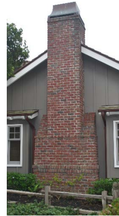
A chimney that is attached to the side of a building should appear to have a direct means of support.
