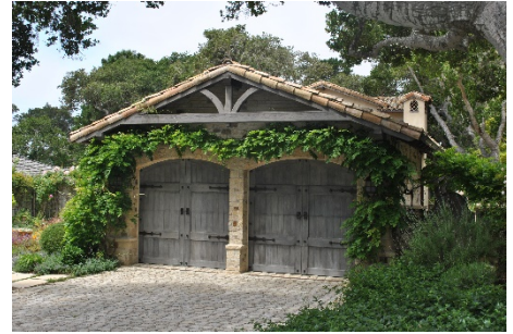
The use of simple wood details that appear to be true structural elements is appropriate.
