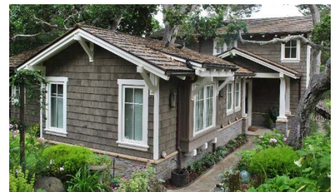
Stone treatments should wrap around the full exterior of a building, and should not be limited to just the street elevation.
