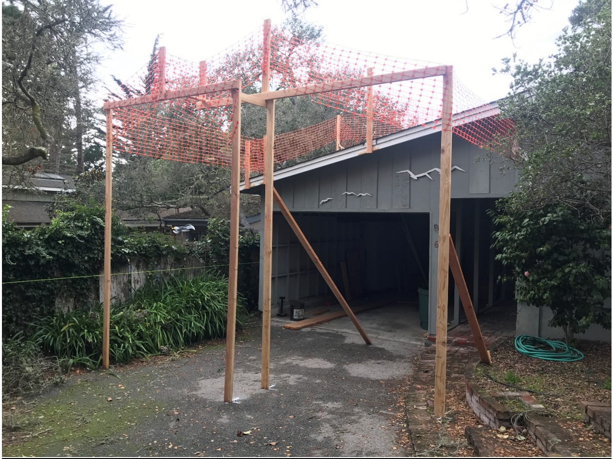
Figure 3: Story Poles for proposed master bedroom addition.
