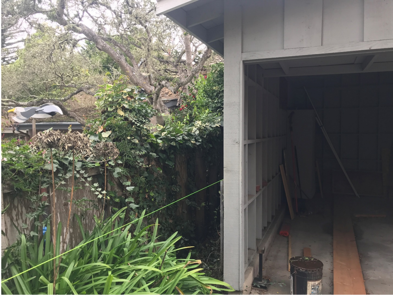
Figure 4: Non-conforming carport wall. The subject wall does not meet the composite setback requirements. The wall shall remain intact for the duration of construction, and any removal shall require the wall to be brought into a compliant location. The yellow/green string in the photo indicates the location of the 3' setback.
