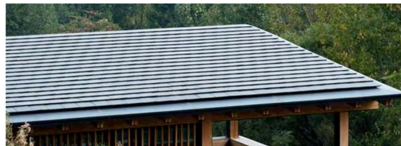
Roofing Class 'A' Composite Slate Roof in Light Gray Color with Flat Seam Zinc Eaves
