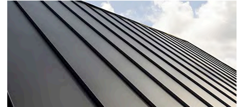
Sloped Roof Standing Seam Metal Roof
