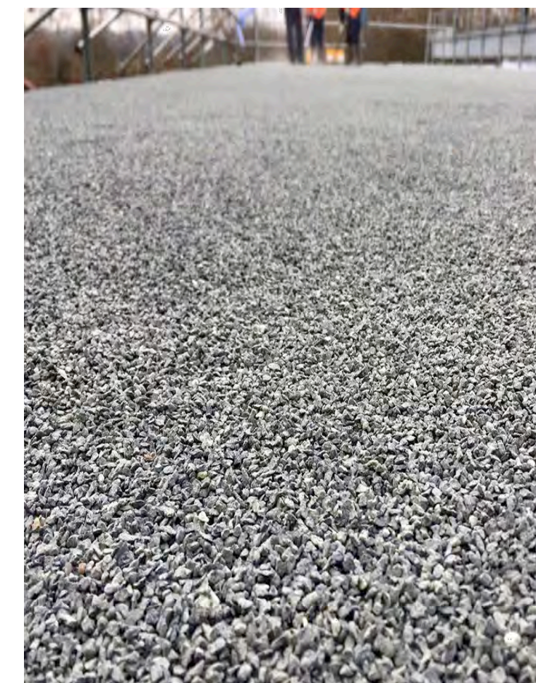
Flat Roof TPO w/ Gravel Ballast
