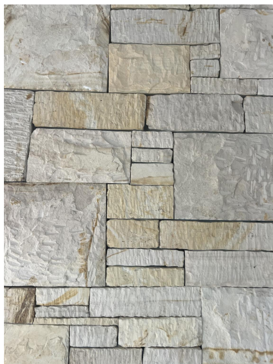
CARMEL STONE @ ENTRY AND CHIMNEY
