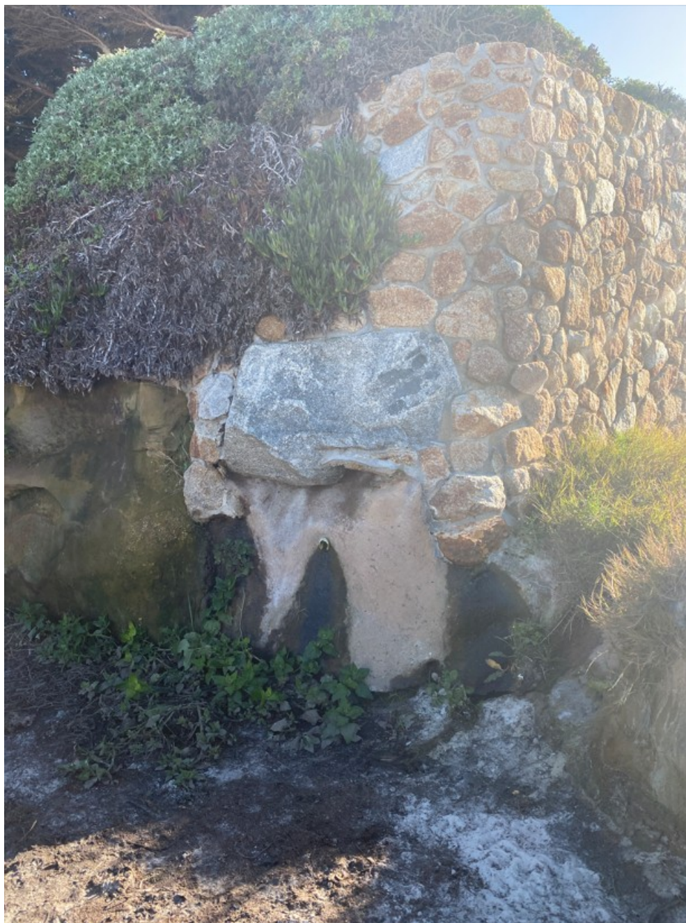
Photograph 13: North End of Seawall S2 on December 22, 2022
