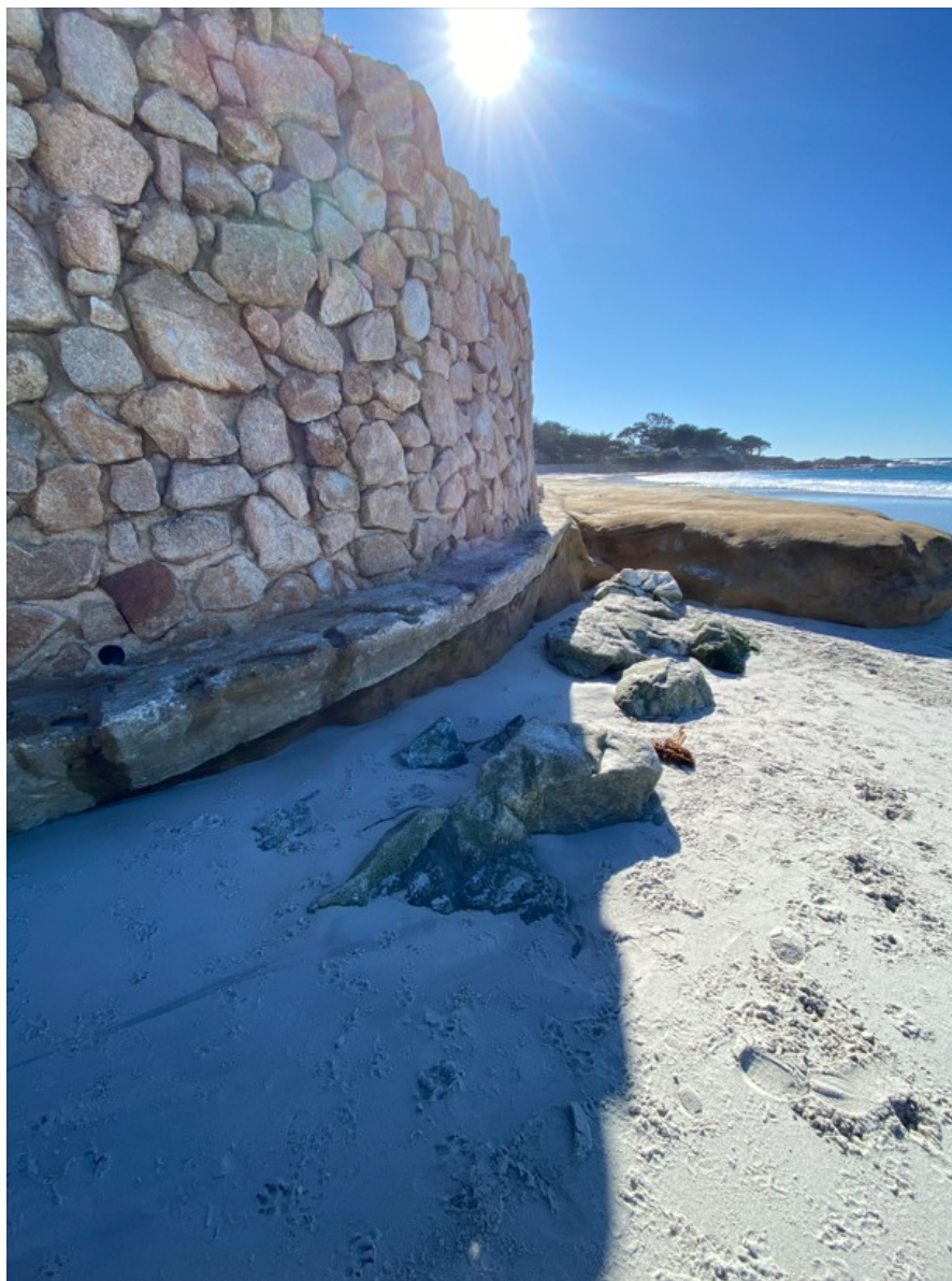
Photograph 31: Looking South at Seawall S3 Adjacent to ST3 on January 30, 2023
