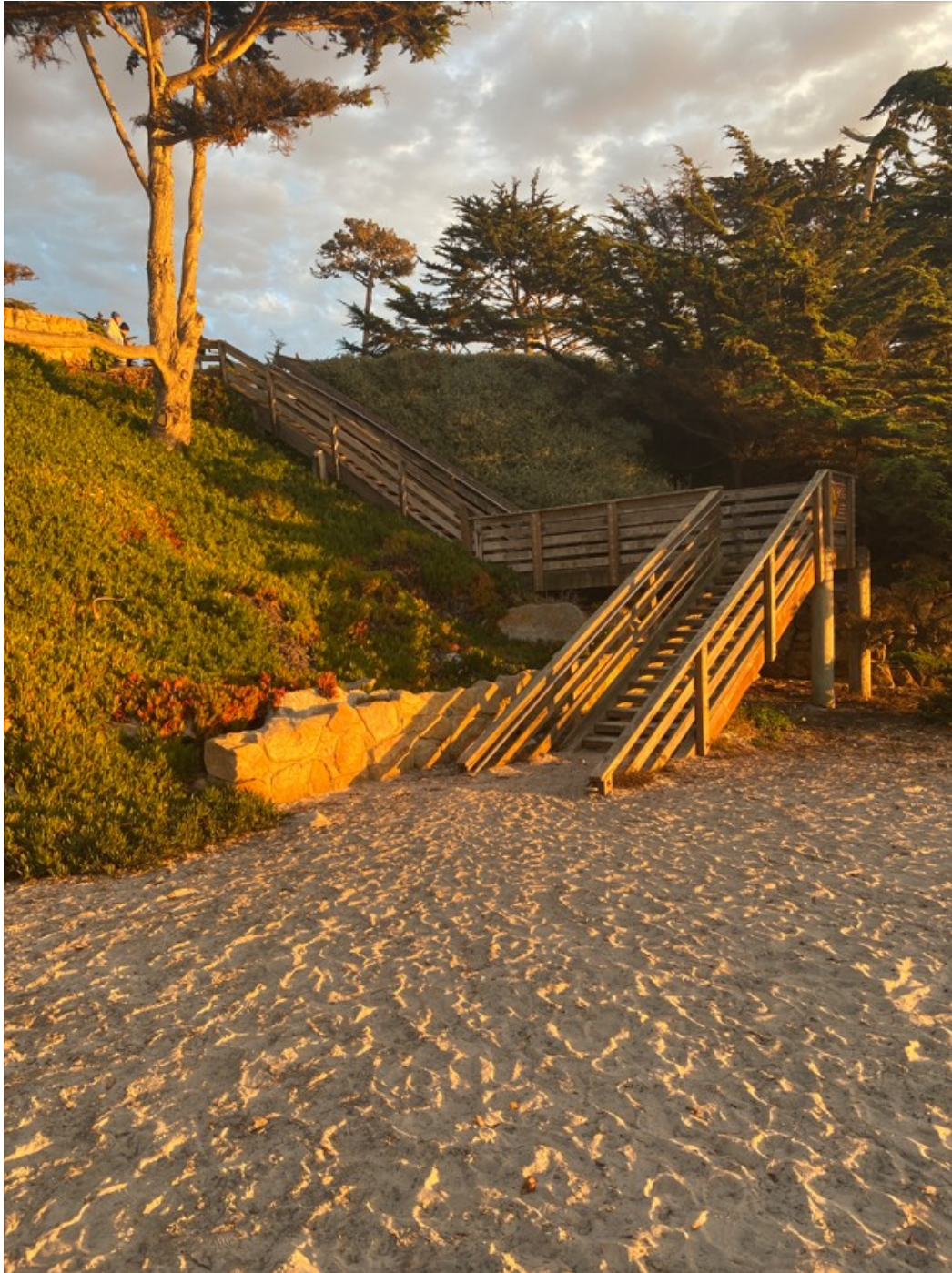
Photograph 72: Stairway ST7 on December 22,2022
