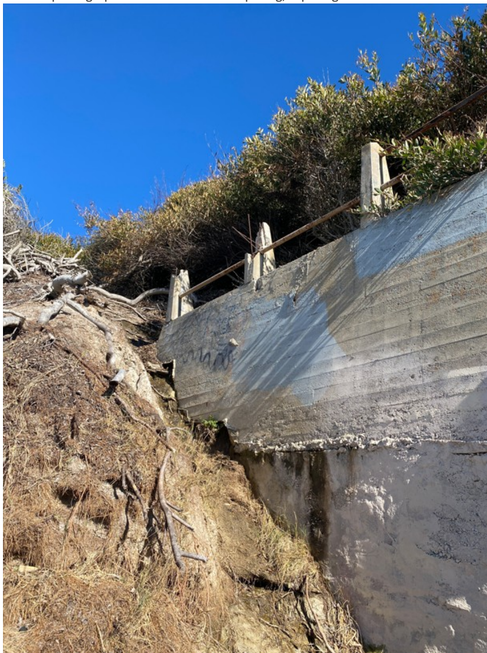
Photograph 94: Seawall S10 on January 30, 2023
