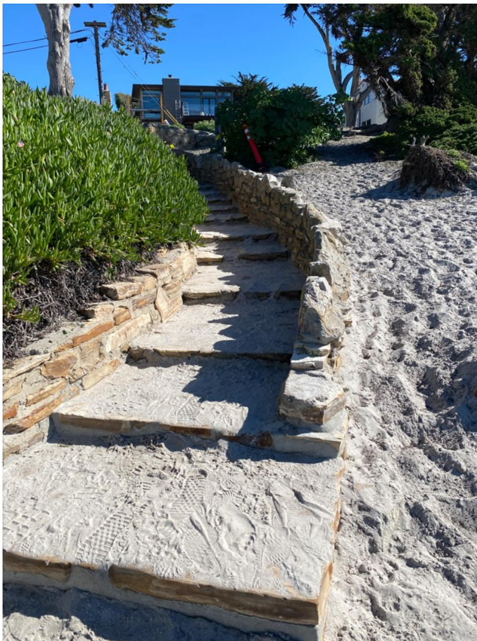
Photograph 86: Stairway ST9 on January 30, 2023
