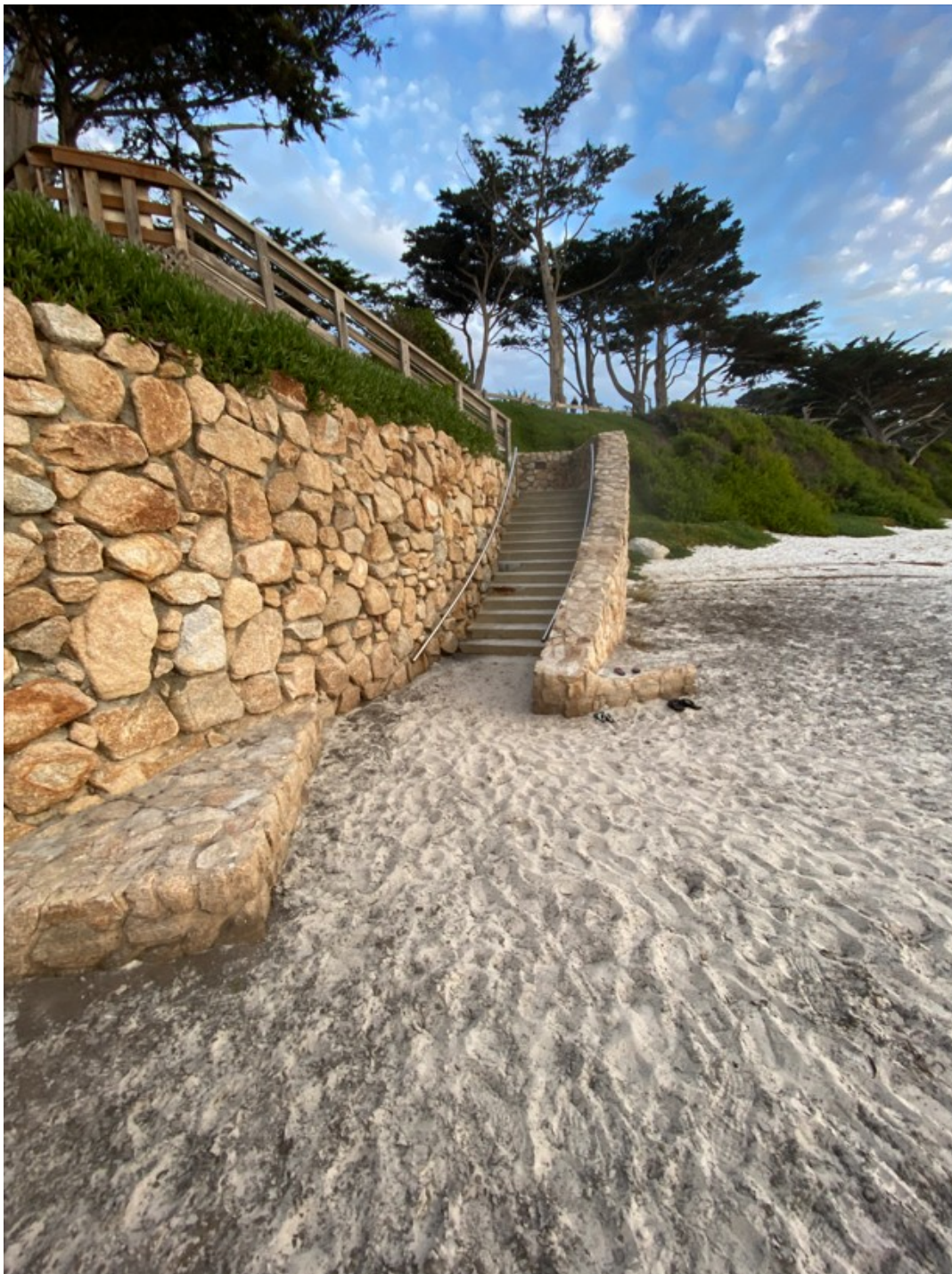
Photograph 64: Showing Stairway ST6 on December 22, 2022
