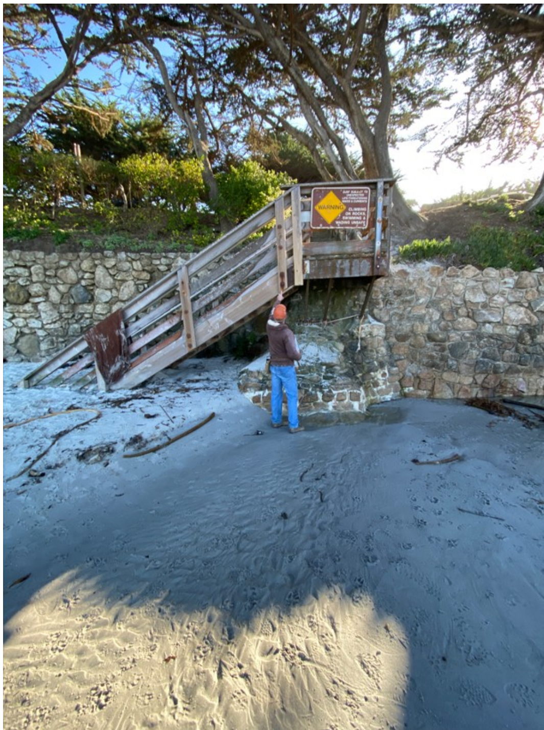
Photograph 4: Stairway ST1 on December 22, 2022
