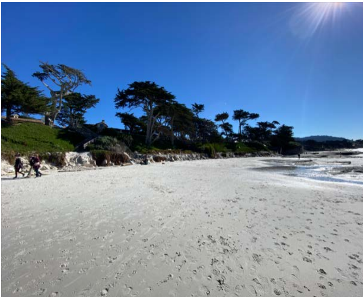
Photograph 78: Central Portion of Revetment R5 on January 30, 2023
