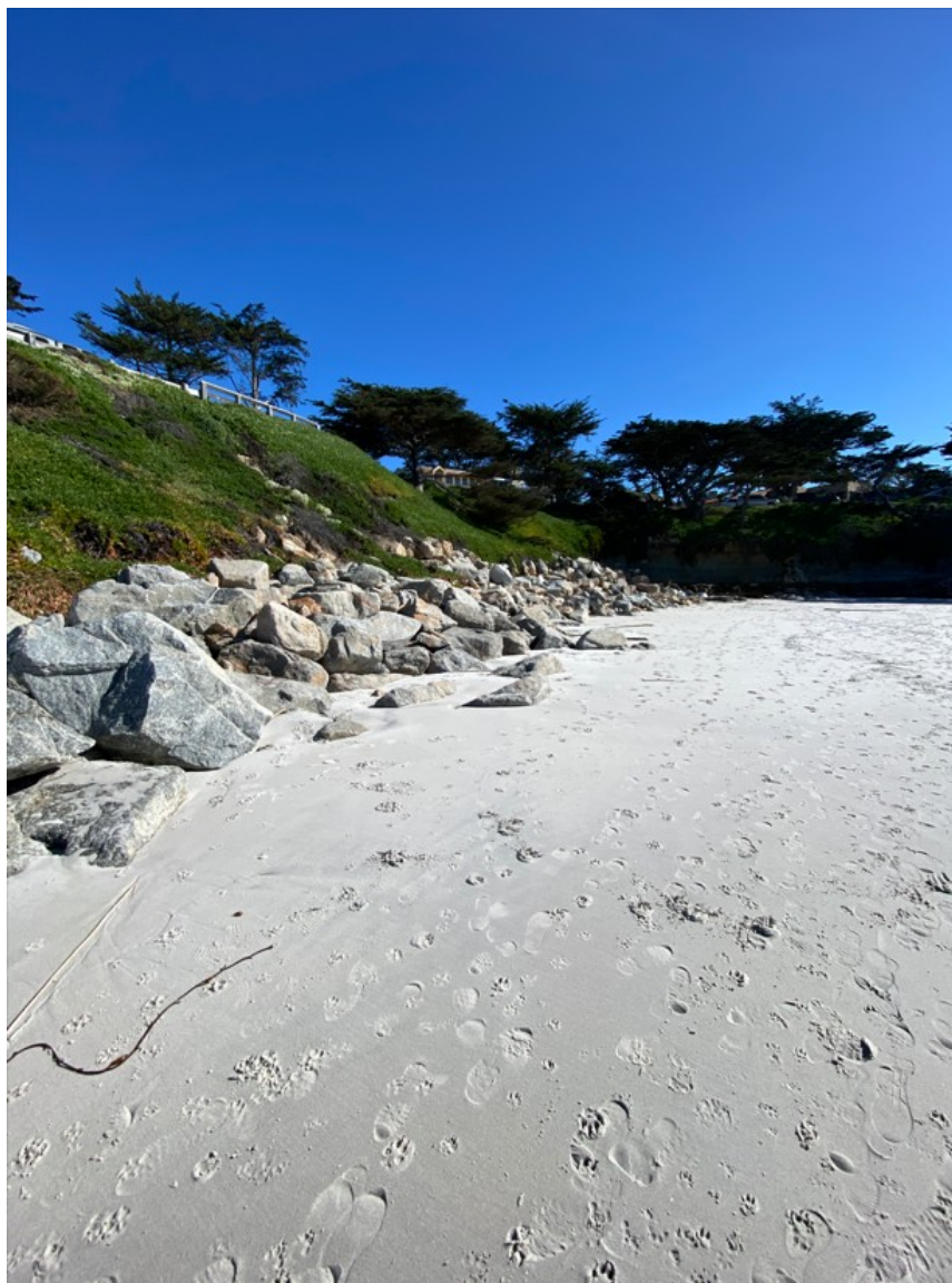
Photograph 49: Showing Revetment R3 Looking South on January 30, 2023
