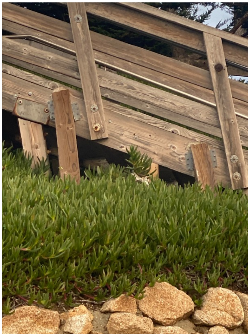
Photograph 65: Showing Recent Maintenance on Stairway ST6 on December 22, 2022
