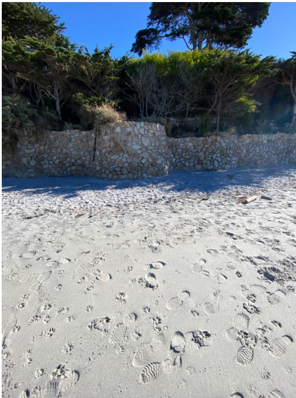
Photograph 98: Central Portion of Privately Owned Seawall S13 Center on January 30, 2023
