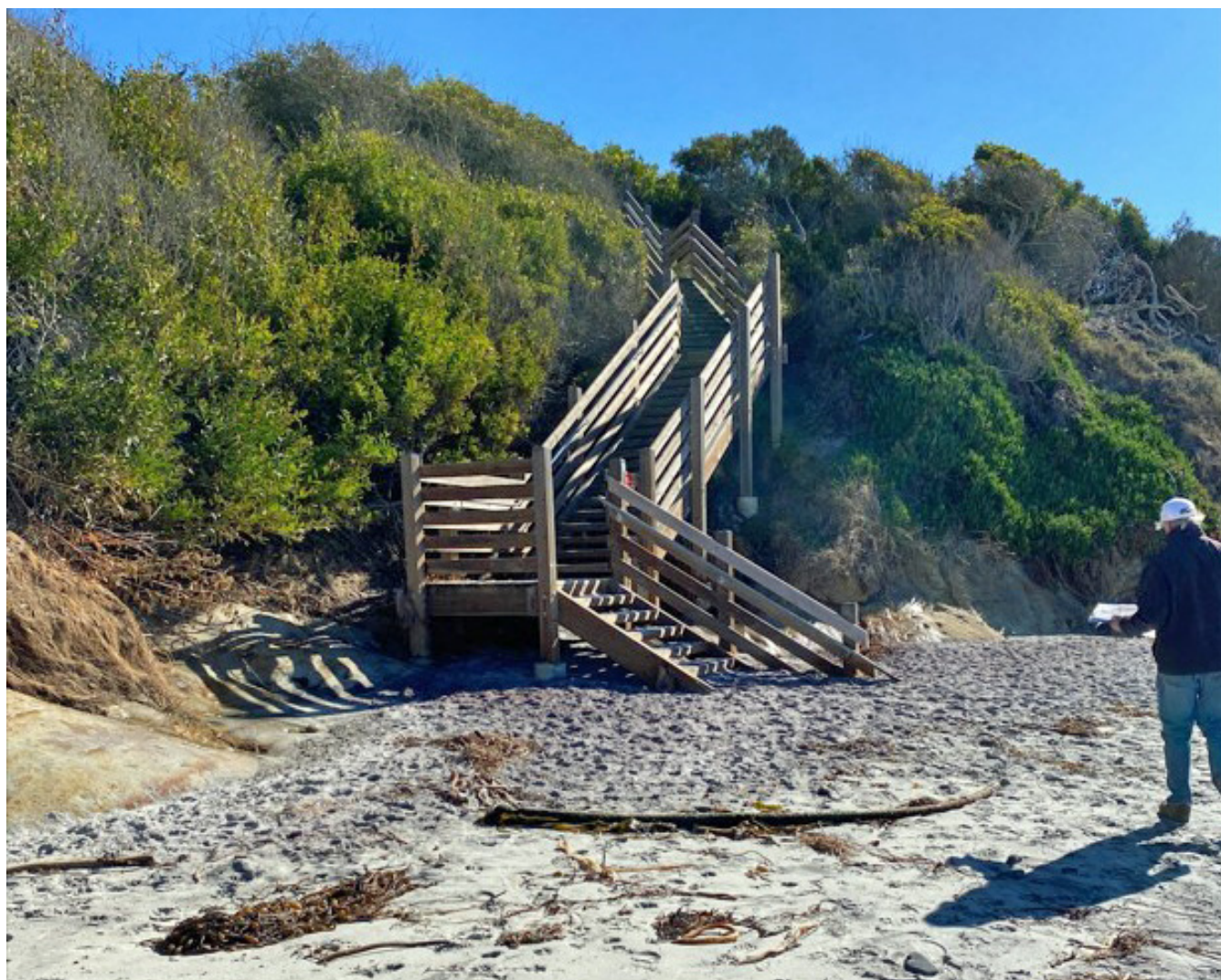
Photograph 96: Stairway ST11 on January 30, 2023
