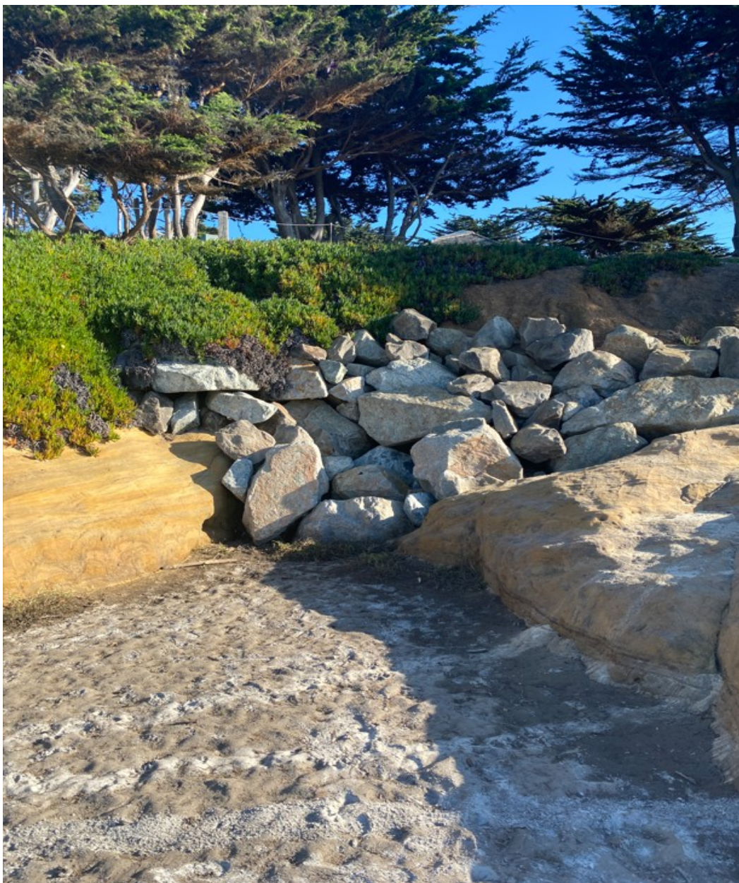
Photograph 19: Revetment R1 on December 22, 2022
