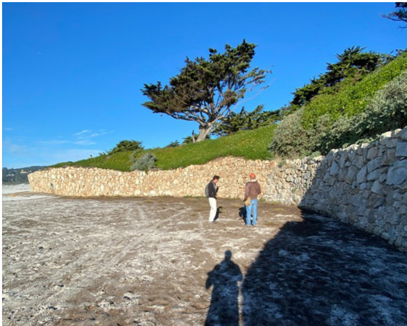
Photograph 25: Looking North at Seawall S3 on December 22, 2022
