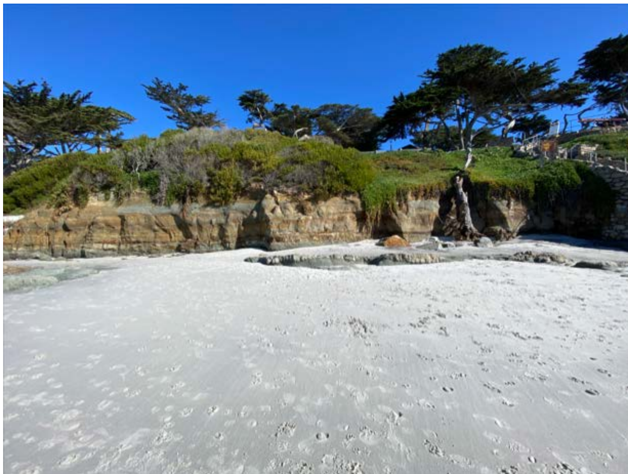
Photograph 59: Showing Bluff South of Revetment R4 on January 30, 2023
