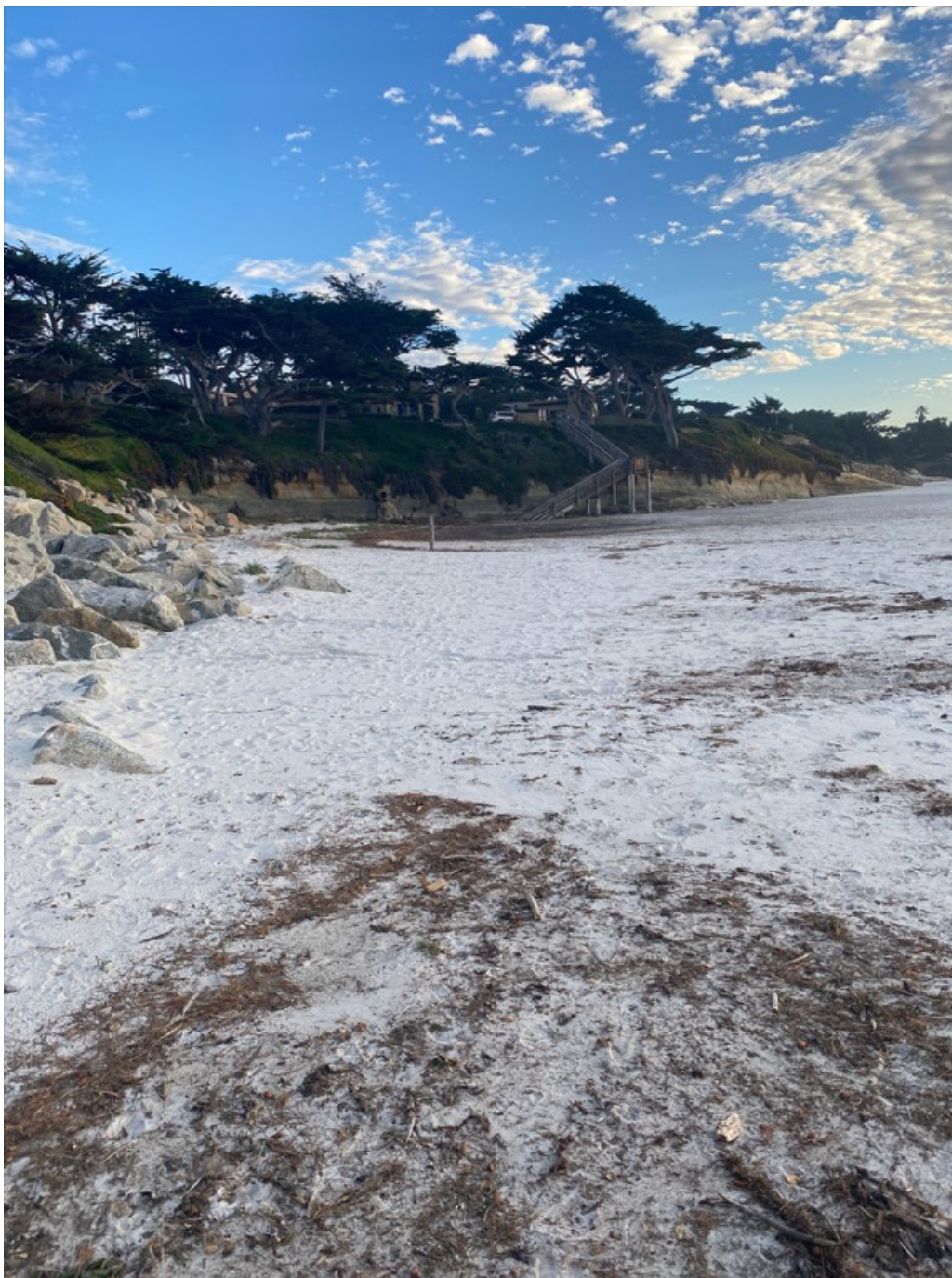
Photograph 46: Looking South along Revetment R3 towards ST4 on December 22, 2022
