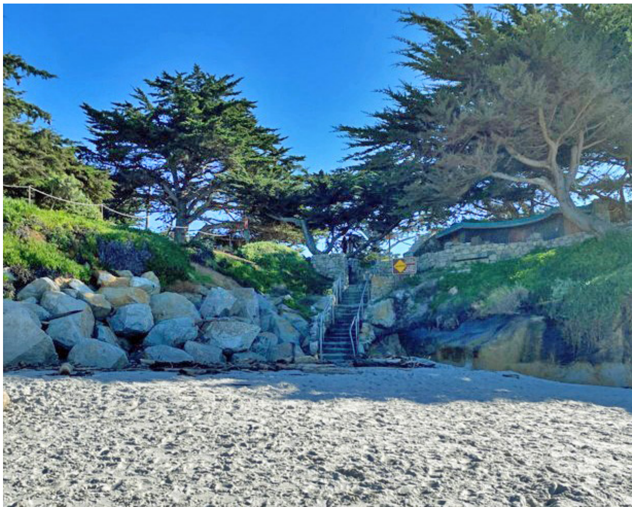
Photograph 15: Showing Revetment R1 and Stairway ST2 on January 30, 2023
