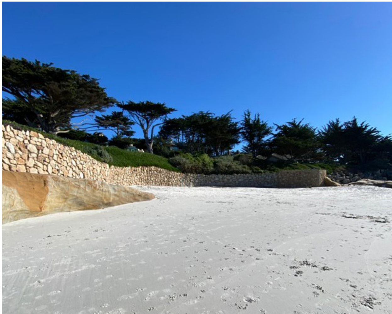
Photograph 35: Showing Seawall S4 on January 30, 2023
