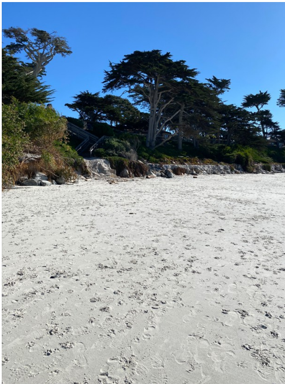
Photograph 84: Showing a Small Amount of Revetment R5 Riprap on January 30, 2023
