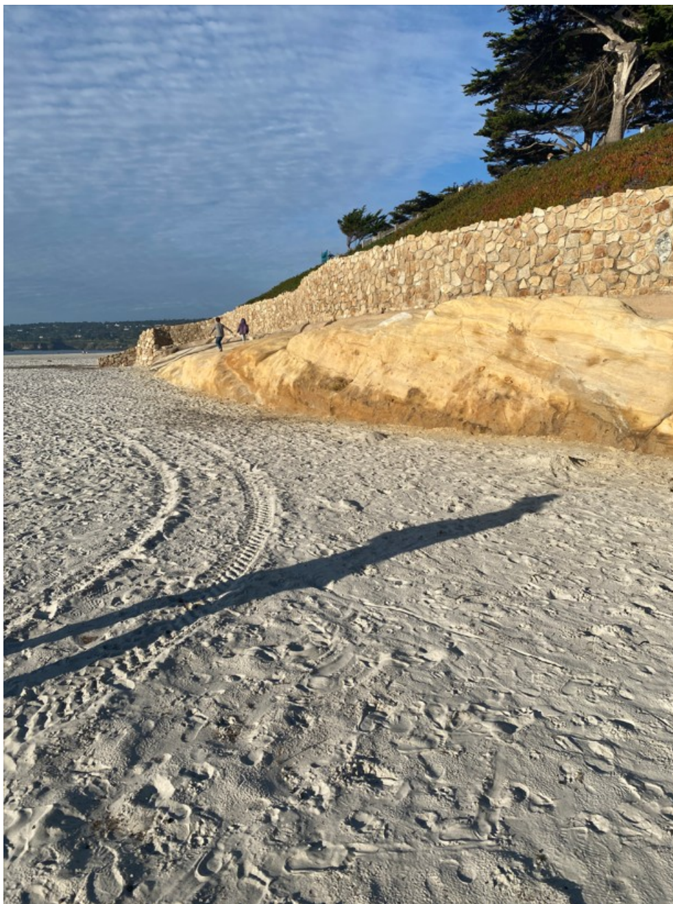
Photograph 36: Showing North Portion of Seawall S4 on December 22, 2022
