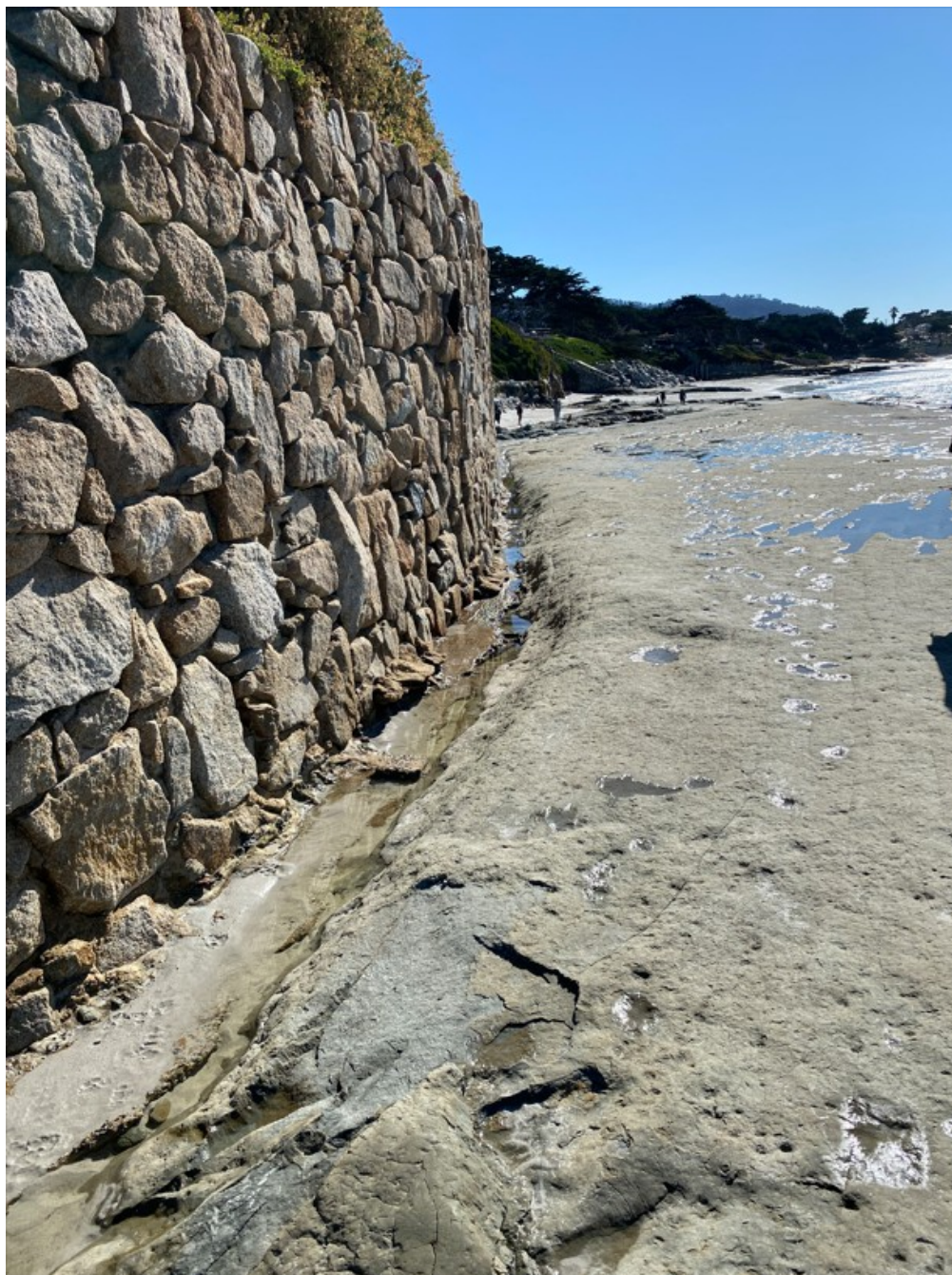
Photograph 71: Seawall S7 Foundation on January 30, 2023
