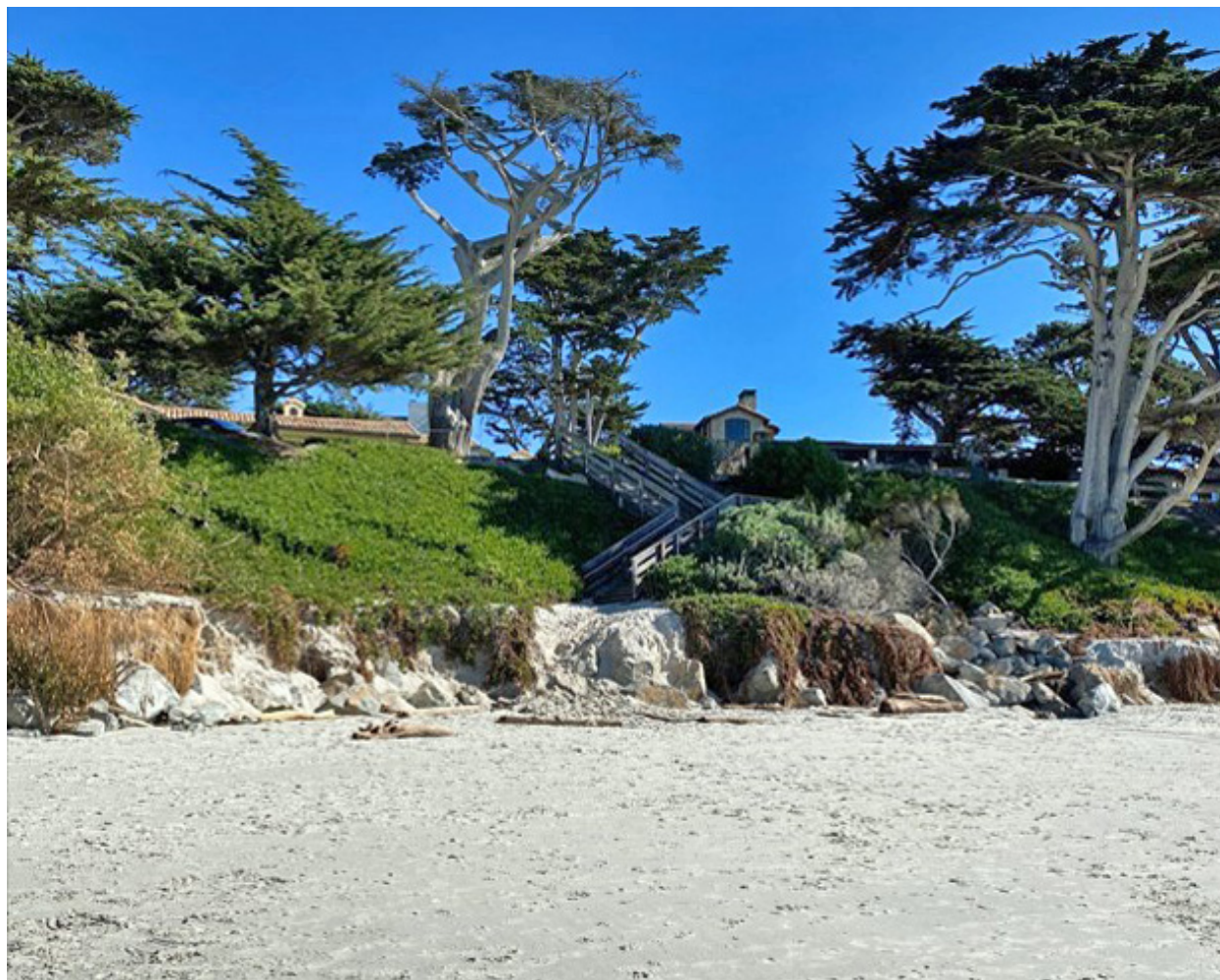
Photograph 79: Showing Beach Access Stairway ST8 on January 30, 2023
