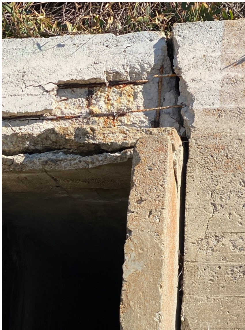
Photograph 95: Seawall S10 on January 30, 2023
