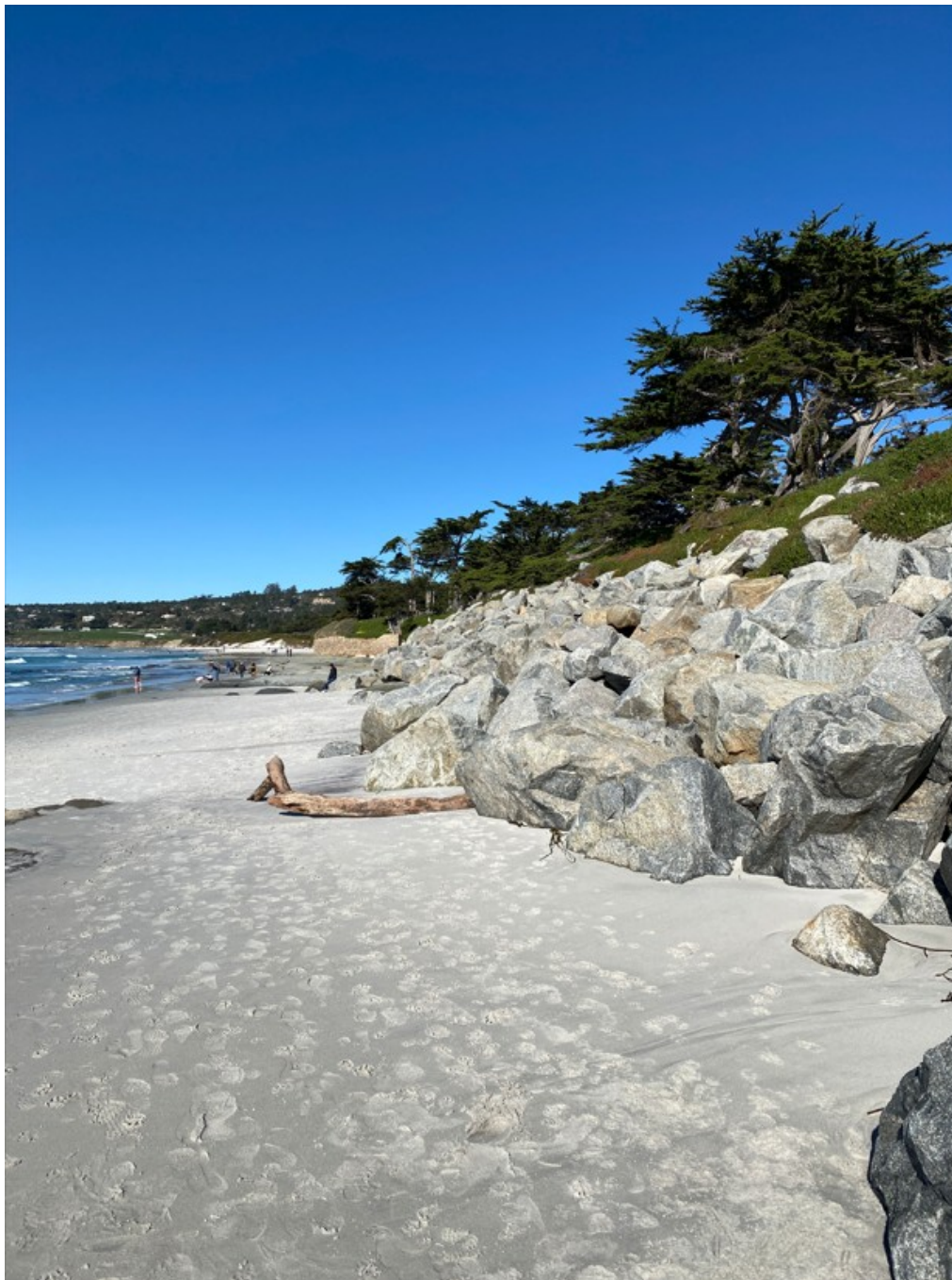
Photograph 52: Showing Revetment R3 Looking North on January 30, 2023
