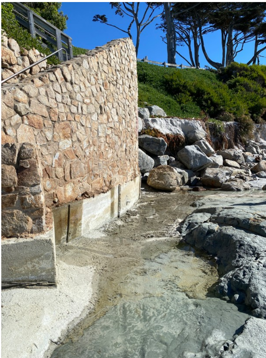
Photograph 68: South Foundation of Seawall S7 on January 30, 2023
