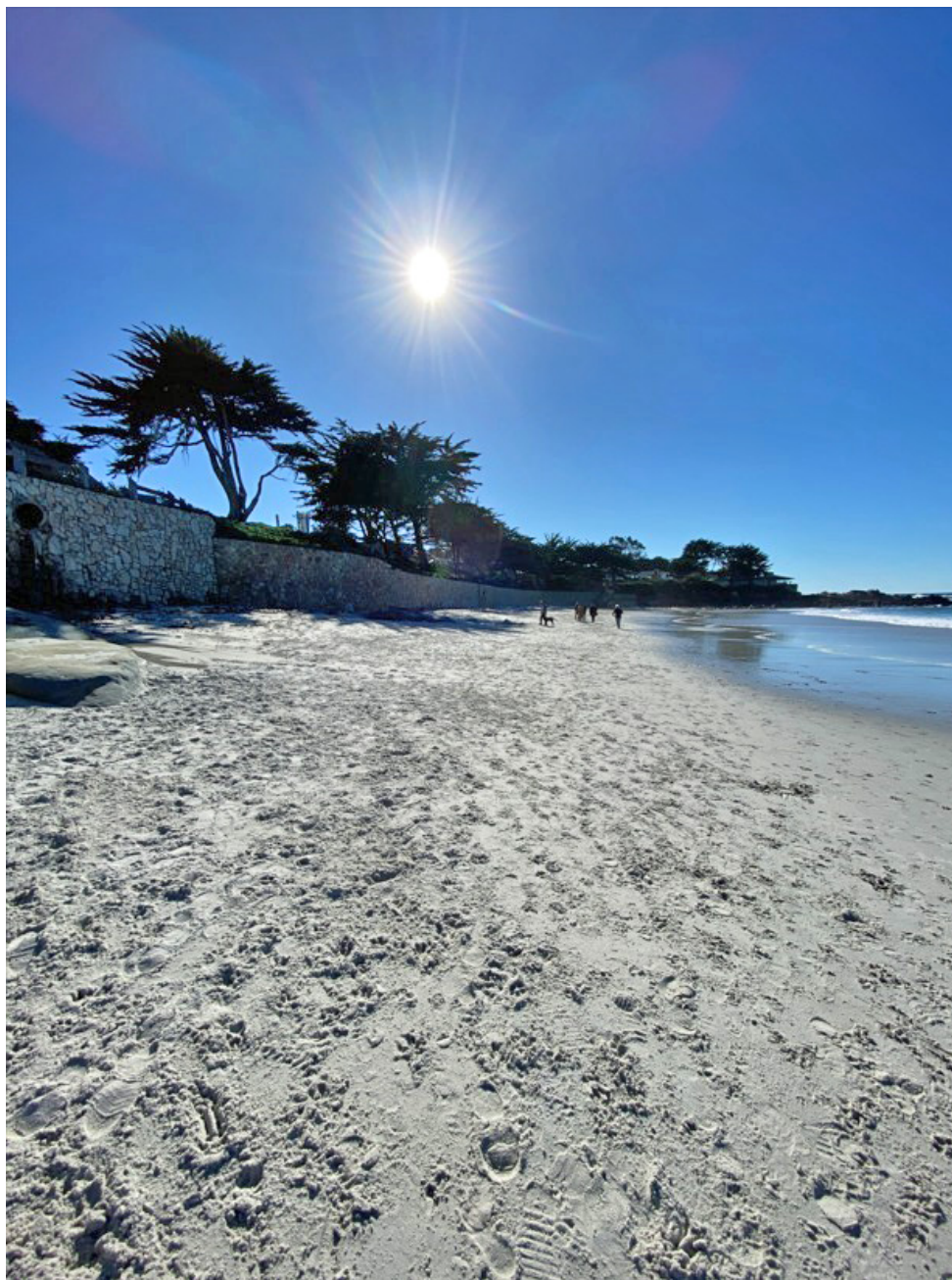
Photograph 8: Showing Seawall S2 on January 30, 2023
