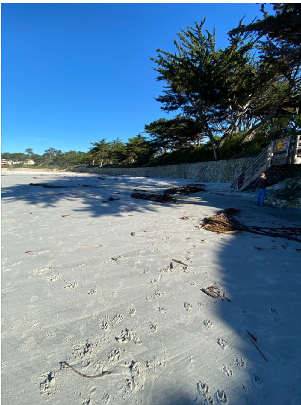
Photograph 3: Seawall S2 on December 22, 2022
