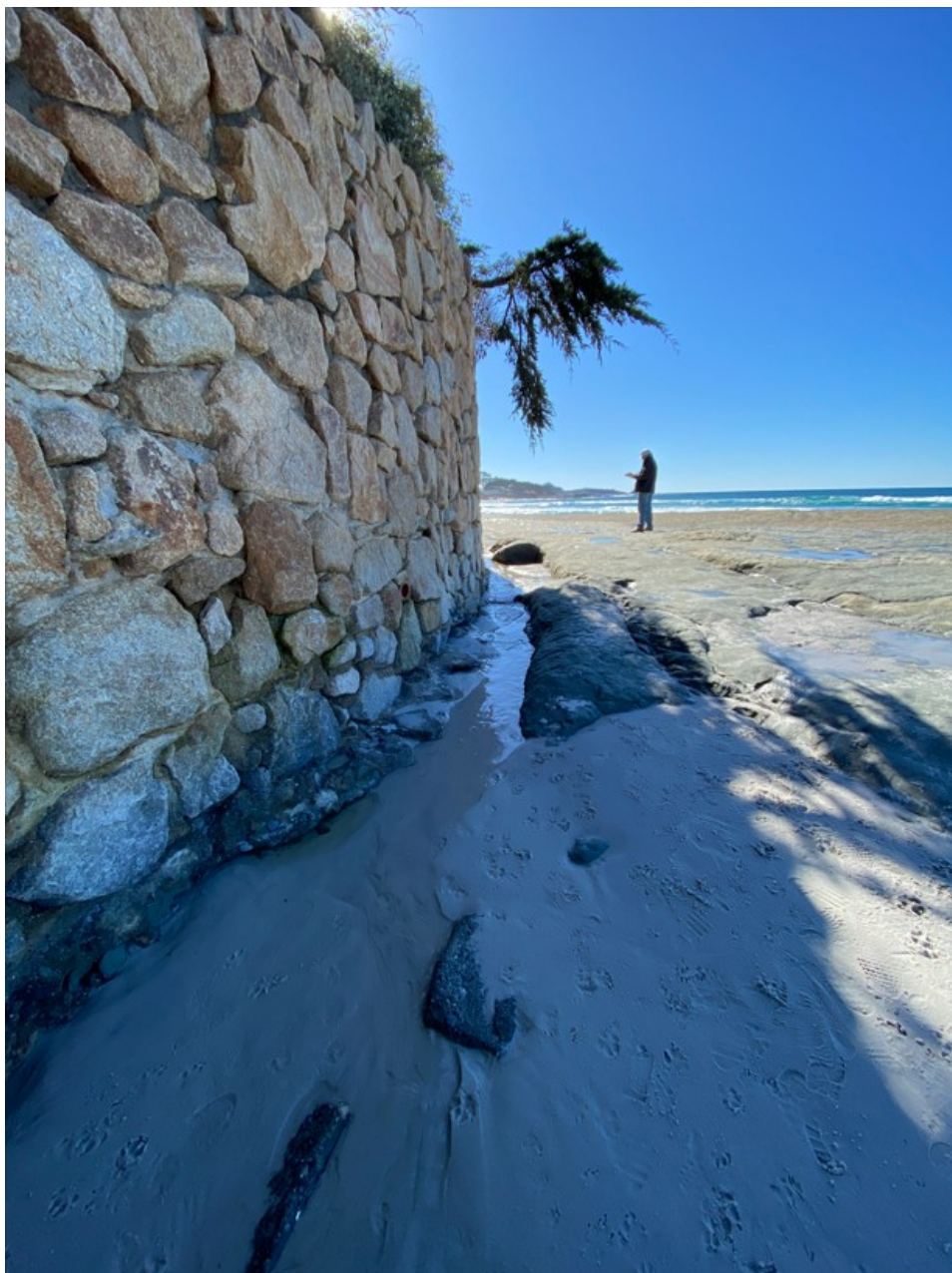
Photograph 70: Seawall S7 Foundation on January 30, 2023
