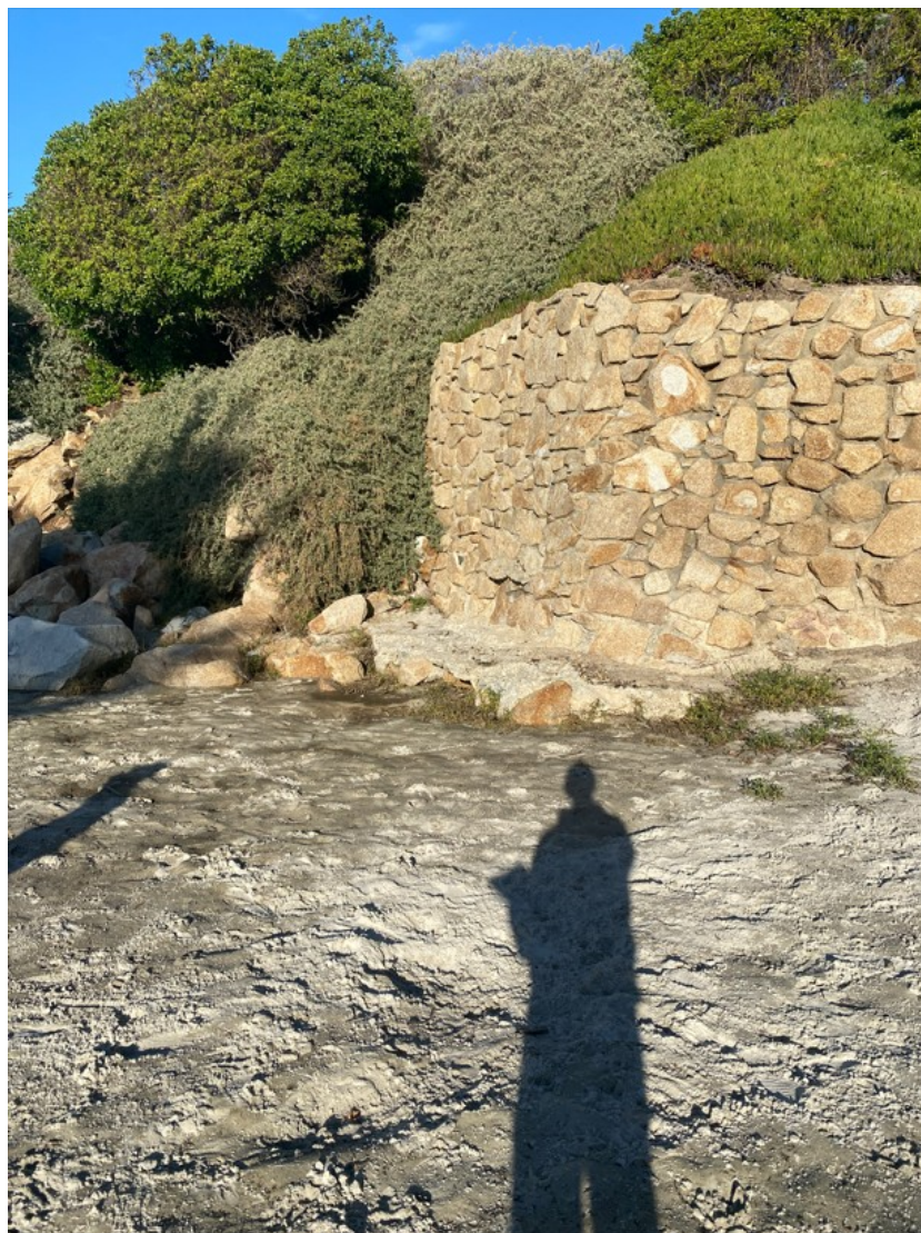
Photograph 32: North End of Seawall S3 on December 22, 2022
