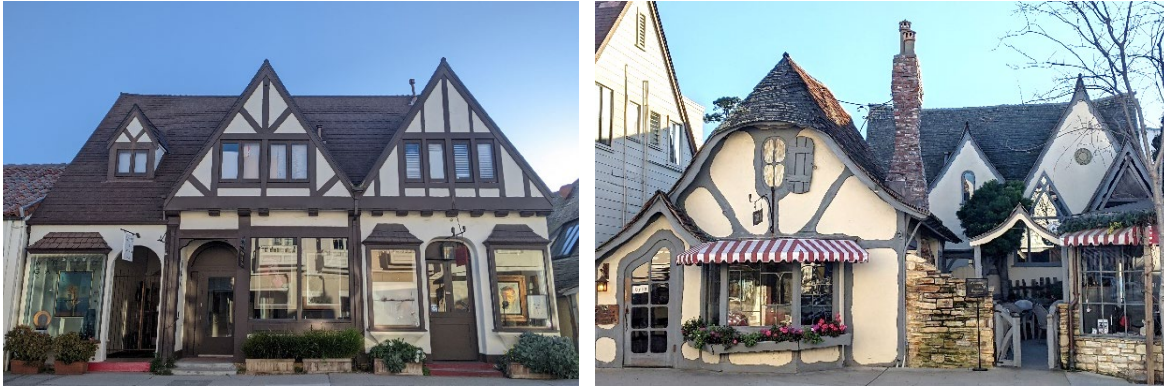
De Yoe Building (1922) on Dolores Street 3 NE of 7 th , with the Tuck Box (1926)(originally, Sallys) and the Lemos Building adjacent at Dolores 2 NE of 7 th . (Source: PAST Consultants, LLC, 2024).
