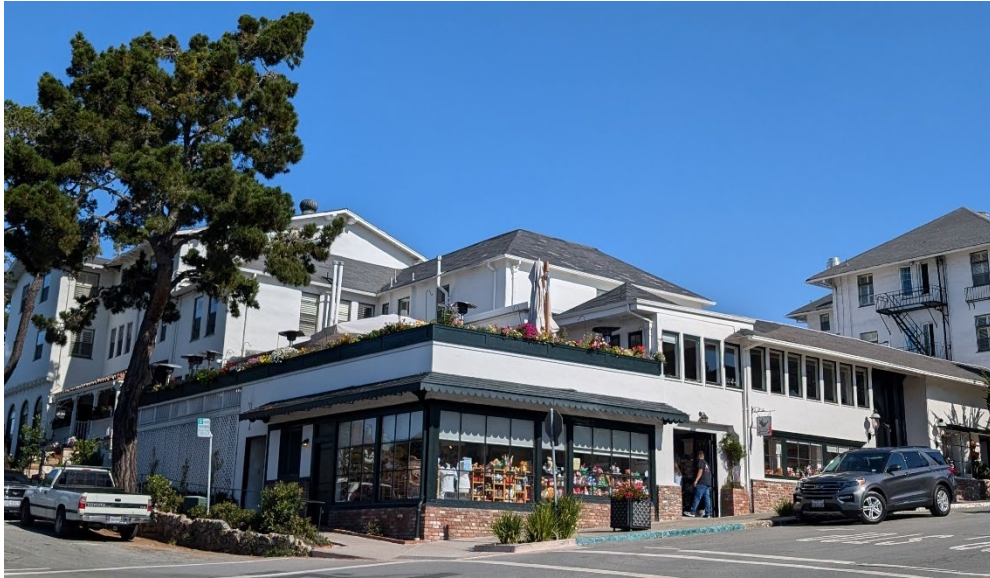
The Pine Inn (1889). (Source: PAST Consultants, LLC, 2024)
