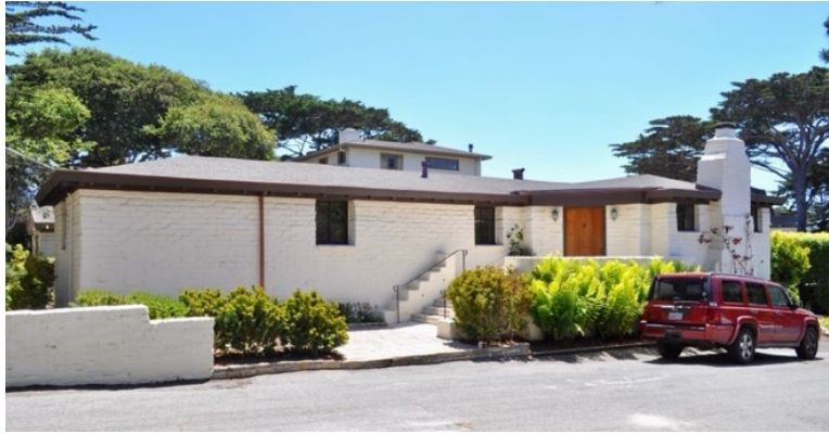
Mrs. B.C. Bowman House (1937), constructed out of “Bitudobe” masonry (Source: PAST Consultants, LLC, 2024 ). 162
