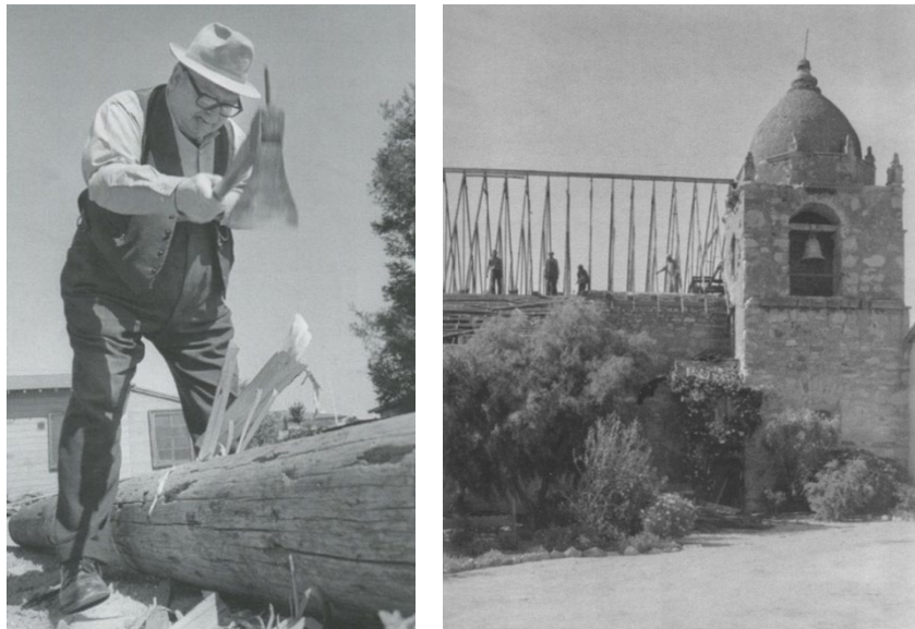
Left: Harry Downie with an adze. Right: 1936 image of the CCC crew installing the structural framing for the Mission’s roof (Sources: Missions of Monterey , 2012).
