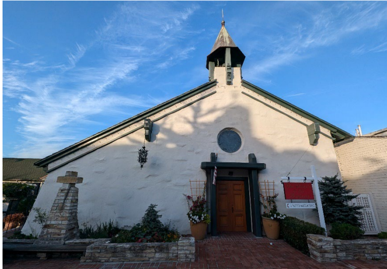
Robert Stanton's Church of the Wayfarer, on the southwest corner of Lincoln St. and 7 th Ave. (Source: PAST Consultants, LLC, 2024)
