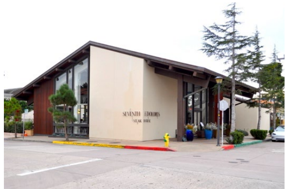
Northern California Savings and Loan (1972) by Burde and Shaw on the SE corner of Dolores St. and 7 th Ave.
