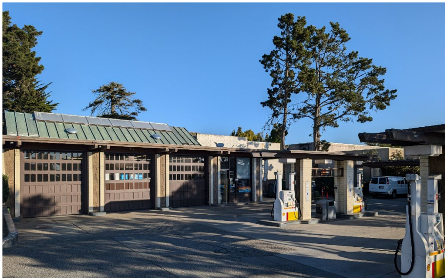
Shell Gas Station (1966) by Burde Shaw Associates on the SE corner of San Carlos St. and 5 th Ave. (Source: PAST Consultants, LLC, 2024).
