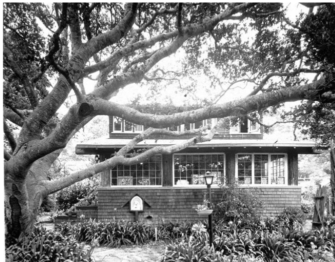
Arnold Genthe House (1906) on Camino Real 2 NE of 11 th . Note redwood trunks utilized as vertical structural supports (Source: Morley Baer photograph, Monterey Area Architectural Resources Archive)
