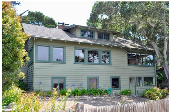
George F. Beardsley House (1909), southwest corner Casanova and 8 th
