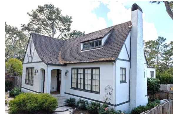
Ross E. Bonham House (1926), SW corner San Carlos and 12 th
