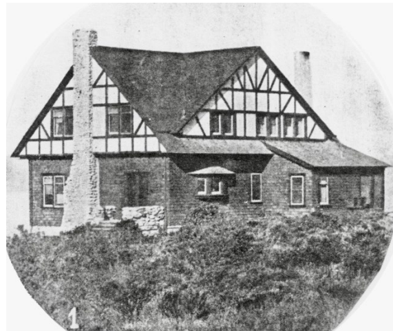
Early image of Grace McGowan Cook House (“Locksley Hall”)(1905) designed for the writer Grace McGowan Cooke and her sister Alice McGowan, extant on the north side of 13 th Ave between San Antonio Street and Carmelo (Source: Carmel: A History in Architecture ).
