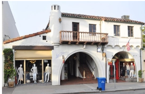
Las Tiendas Building (1930), south side of Ocean between San Carlos and Dolores
