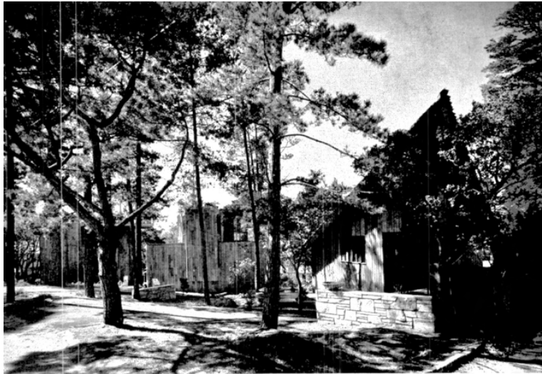
Albert Henry Hill's three Weekend Houses on Lopez Street (Source: Progressive Architecture , August 1962). 161
