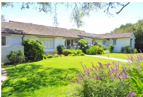
California Ranch house (1947), 2960 Santa Lucia Ave.
