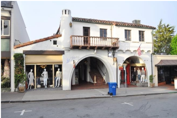
Las Tiendas Building, south side of Ocean between San Carlos and Dolores
