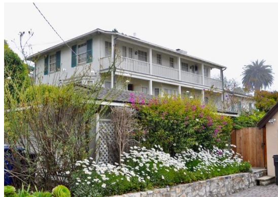
Holmes House, rear elevation, southwest corner of Carmelo and 8 th
