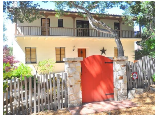
Louis Ralston House, west side of Lincoln between 12 th & 13 th
