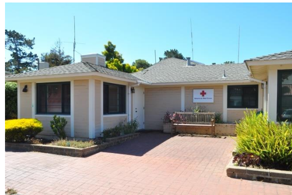
Carmel Red Cross Headquarters (1954) at SE Dolores Street and Eighth Avenue
