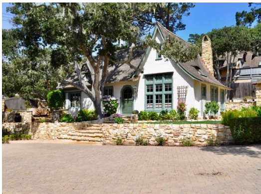
Hugh Comstock House, Northeast corner Torres and 6 th
