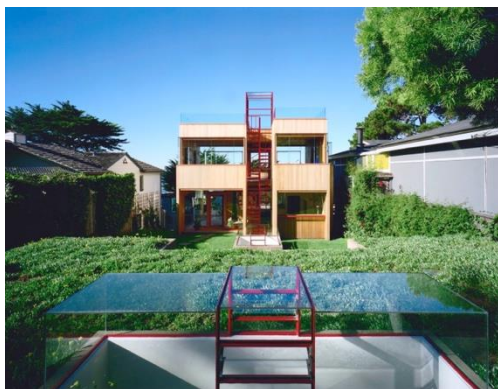
Light House (1982/1997) on Scenic Road between Ocean Ave. and 8 th Ave.
