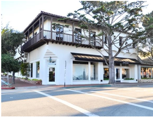
Goold Building, Northeast corner of Ocean and San Carlos
