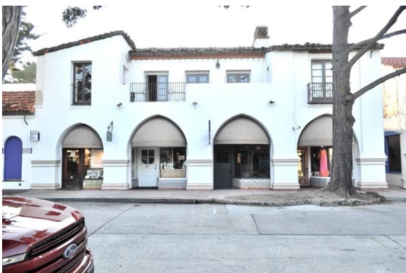
Draper Leidig Building, Dolores St., 2 SE from Ocean
