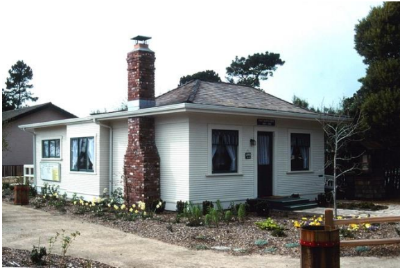
First Murphy House, west side of Lincoln between 5 th and 6 th
