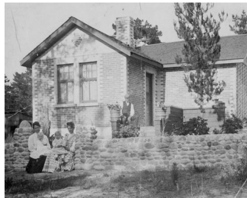
Benjamin Turner House, Monte Verde St. 2 SE of 5 th Ave. 67
