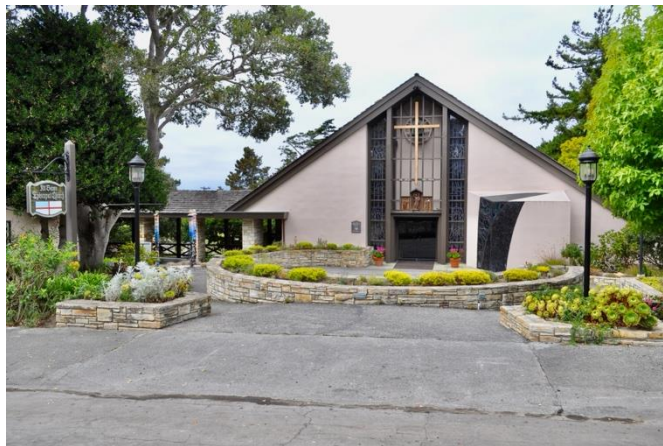
All Saint’s Episcopal Church on the southeast corner of Dolores St. and 9 th Ave. (Source: PAST Consultants, LLC, 2024).
