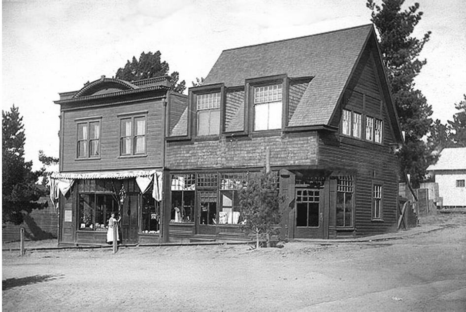
Historic image of the extant 1905 Shingle-style Philip Wilson real estate office at the northwest corner of Ocean Avenue and Dolores Street (Source: Carmel: A History in Architecture: Images of America ).
