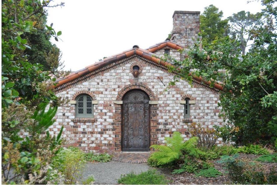
Charles Greene studio on Lincoln Street, 4 southwest of 13 th Avenue (Source: PAST Consultants, 2024)
