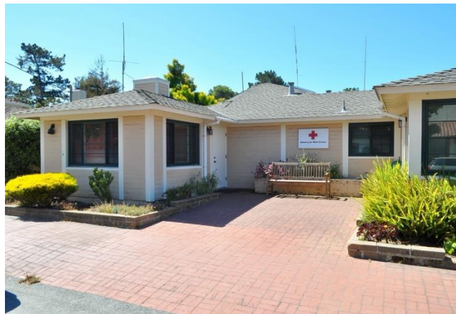
American Red Cross Building, on SE corner of Dolores St. and 8 th Ave. ( Source: PAST Consultants, LLC, 2024 ).
