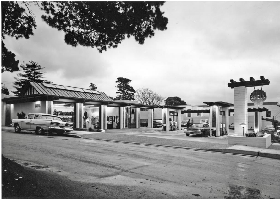
Shell Gas Station (1964) by the firm of Walter Burde and Will Shaw on San Carlos and 5 th (Source: Carmel: A History in Architecture ).
