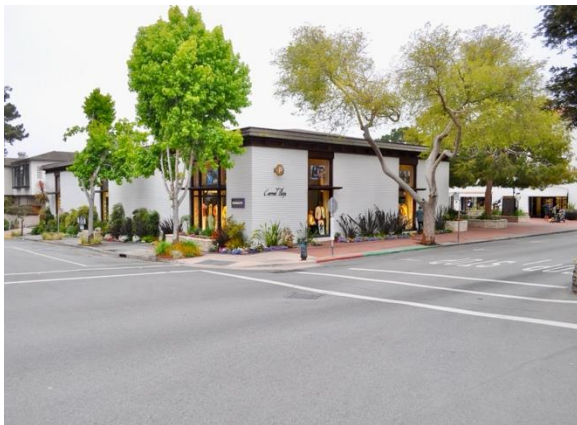
Modifications to Carmel Plaza (1974), on the southwest corner of Ocean Avenue and Junipero Street ( PAST Consultants, LLC 2024 )
