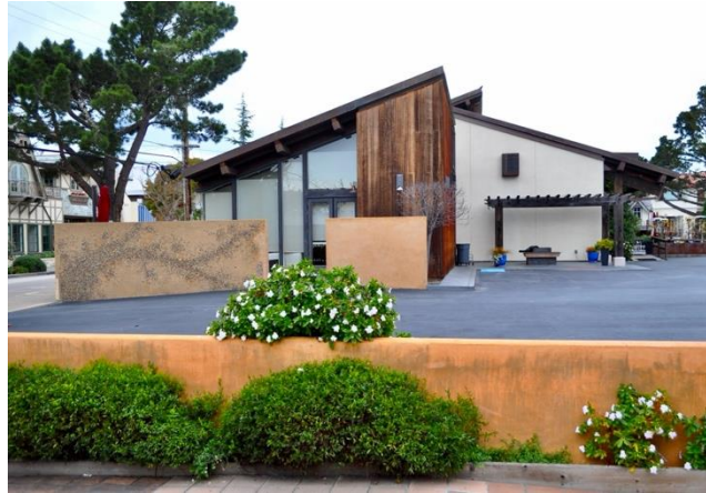
South Elevation showing the nested shed roofs of the Northern California Savings and Loan Complex (1972) by Burde and Shaw, on the southeast corner of Dolores Street and 7 th Avenue ( Source: PAST Consultants, LLC 2023 ).
