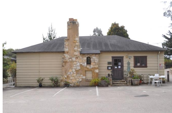
Sunset School Primary Classroom #18, SE corner of Sunset Center campus.
