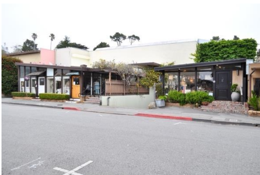
Postwar Modern commercial buildings on the east side of Dolores Street between 5 th and 6 th Avenues
