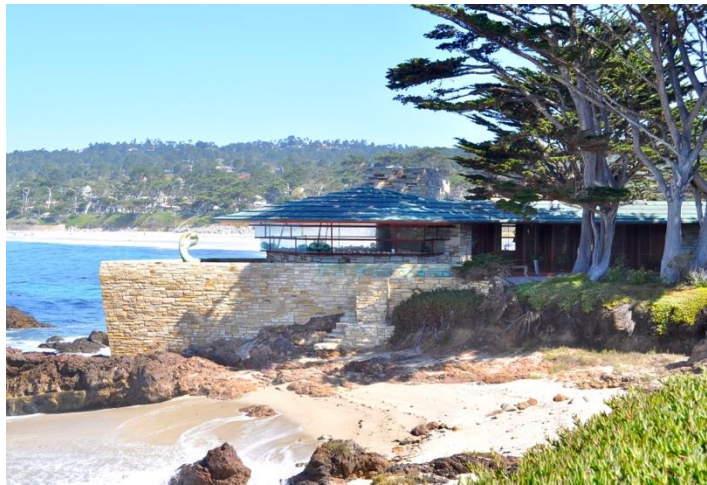
Recent view of Mrs. Clinton Walker House (Source: PAST Consultants, LLC , 2024).
