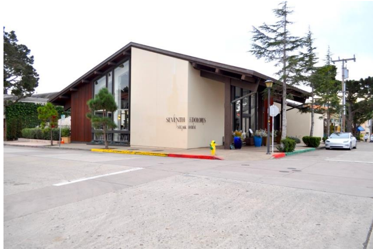
Northern California Savings and Loan (1972) by Burde and Shaw on the southeast corner of Dolores Street and 7 th Avenue (Source: PAST Consultants, LLC 2023).
