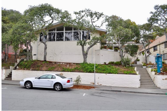
Carmel Ballet Academy on Mission Street between 7 th and 8 th Avenues ( Source: PAST Consultants, LLC, 2024 ).
