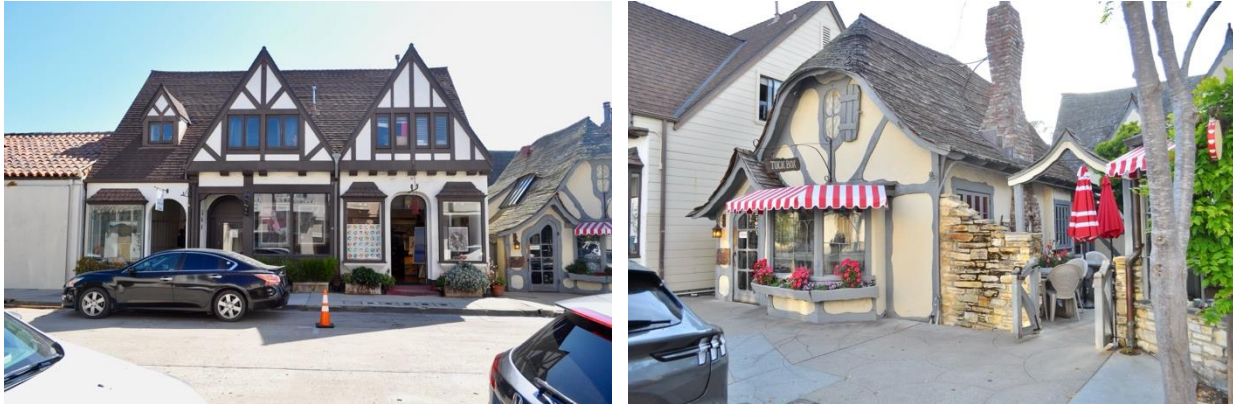
M.J. Murphy’s De Yoe Building (1922) on Dolores Street, with the Tuck House adjacent. Right: Hugh Comstock’s famous Tuck House (1926) adjacent and to the south ( Source: PAST Consultants, LLC, 2024 ).
