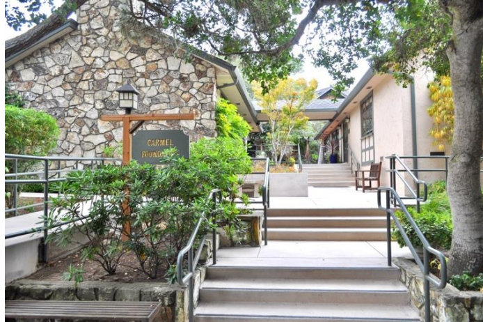
Additions to the Carmel Foundation Complex (1973), by James M. Pruitt, on the east side of Lincoln Street between 8 th and 9 th Avenues. (Source: PAST Consultants, LLC 2024).
