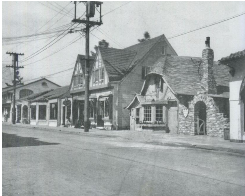
East side of Dolores Street, between Ocean and 7 th , circa-1931. From left to right: Isabel Leidig Building (1925); W.C. Farley Building (1927); Vining's Meat Market (Percy Parkes Building - 1926); De Yoe Building (1924); Tuck Box (1926); and a portion of the El Paseo Building (1928). Source: Pat Hathaway Collection, Monterey County Historical Society.
