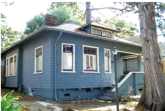
C.H. Gordiner House, east side of Dolores between 9 th and 10 th
