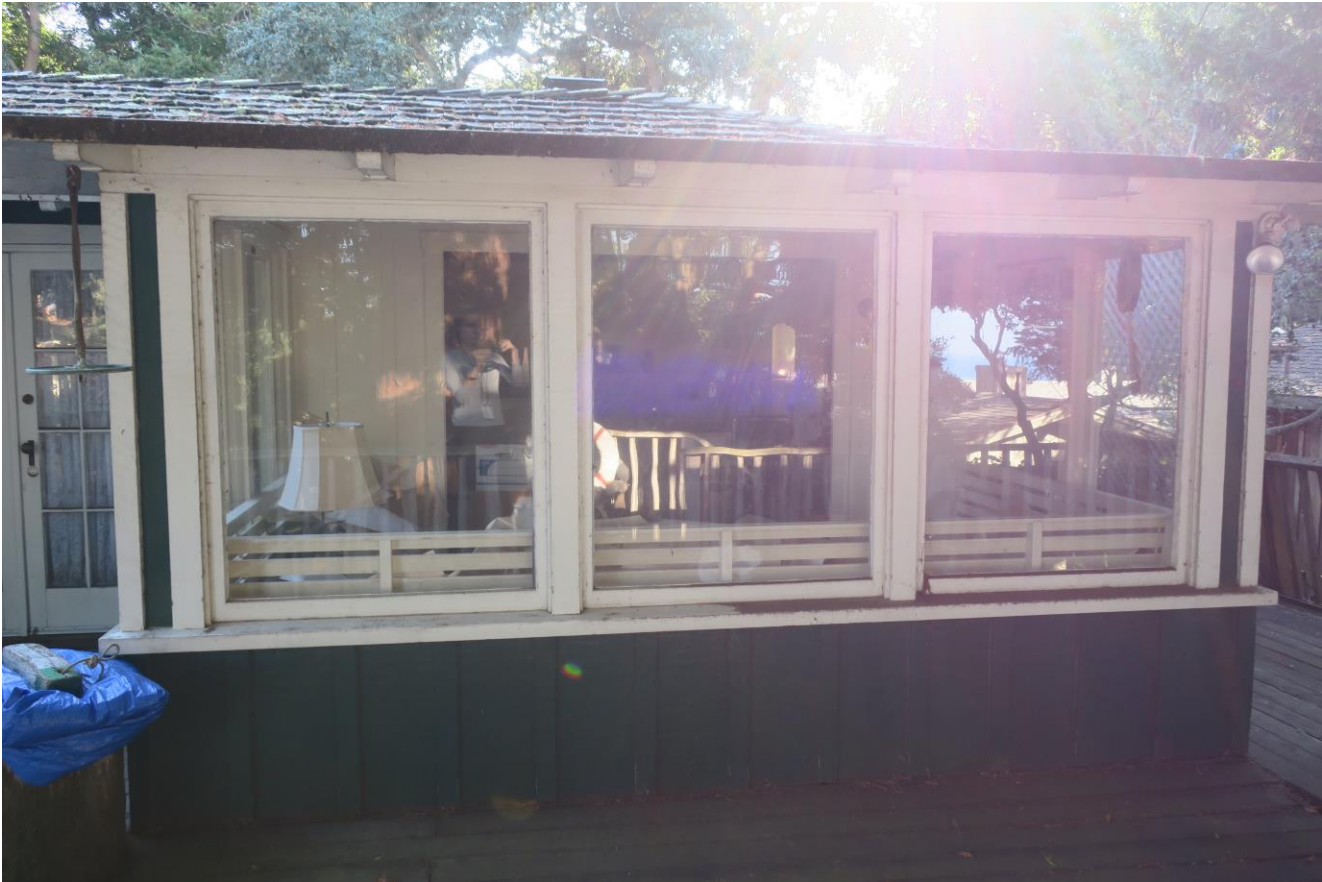
Rear (west) elevation, looking east at sunroom.
