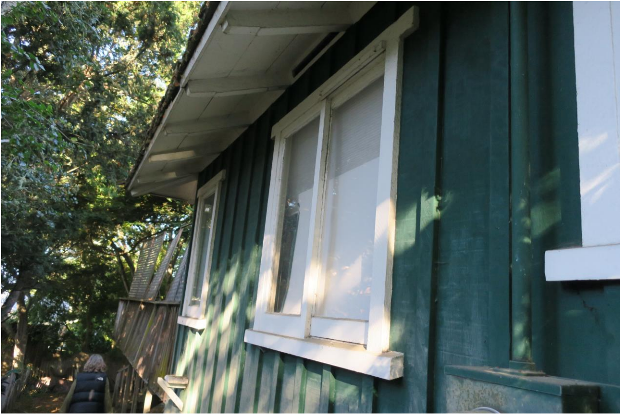
South side elevation, looking west
