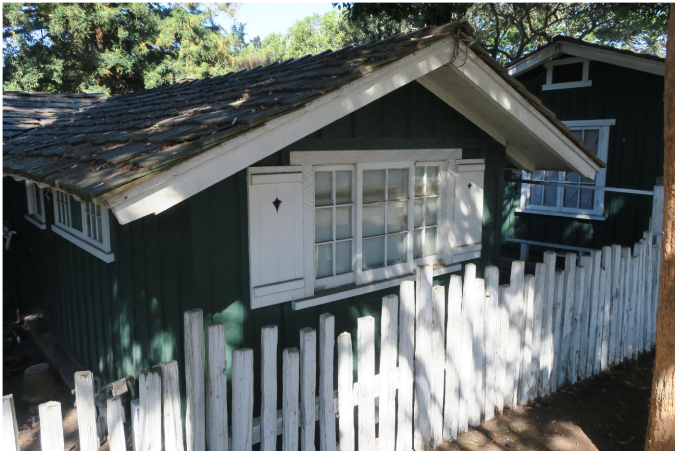
Front wing, looking northwest. Detached garage in background, image right.
