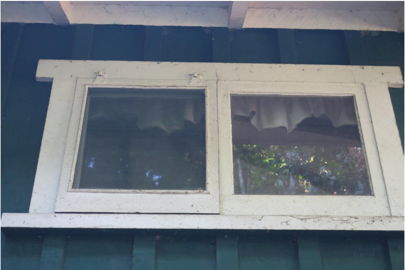
Detail of the "awning light" (left) with screen behind.
