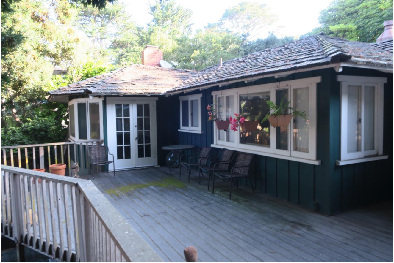
Rear (west) elevation, looking north/northeast.
