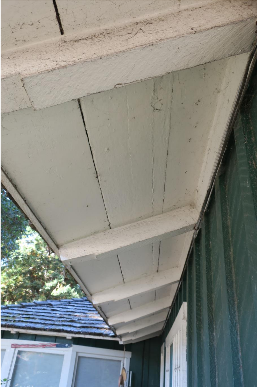
Detail view of exposed notched rafters in the eaves, typical throughout.
