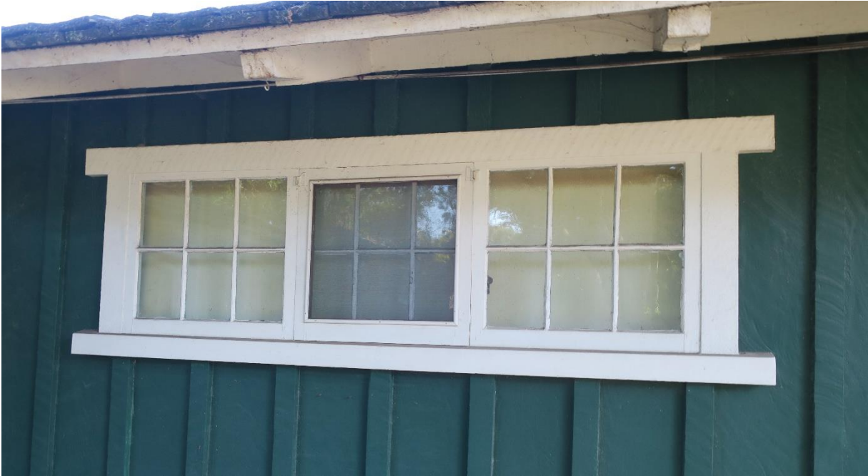
Detail view of extended sill and lintel, typical throughout.
