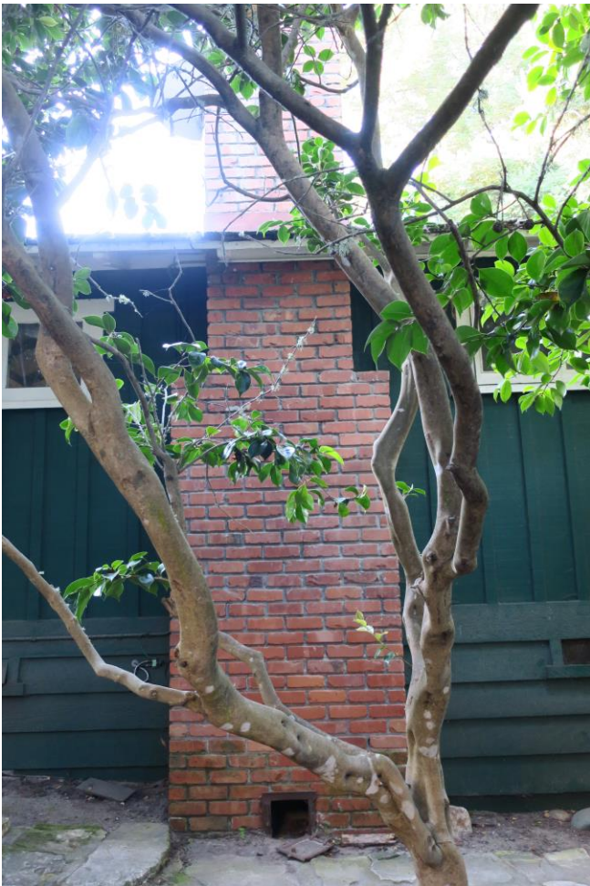
Exterior brick chimney at north side elevation. View looking south.
