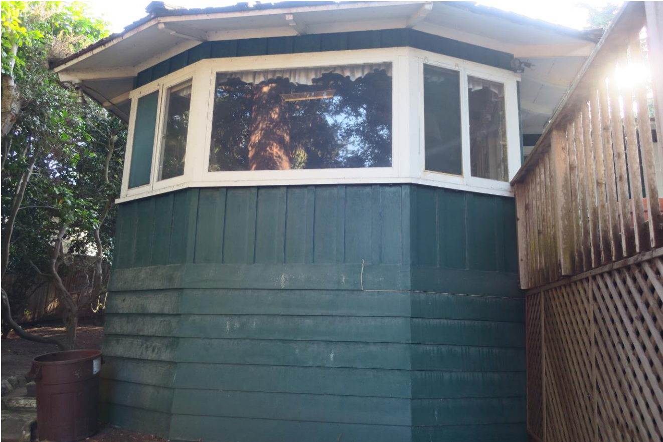
Rear (west) elevation, looking east at bay.
