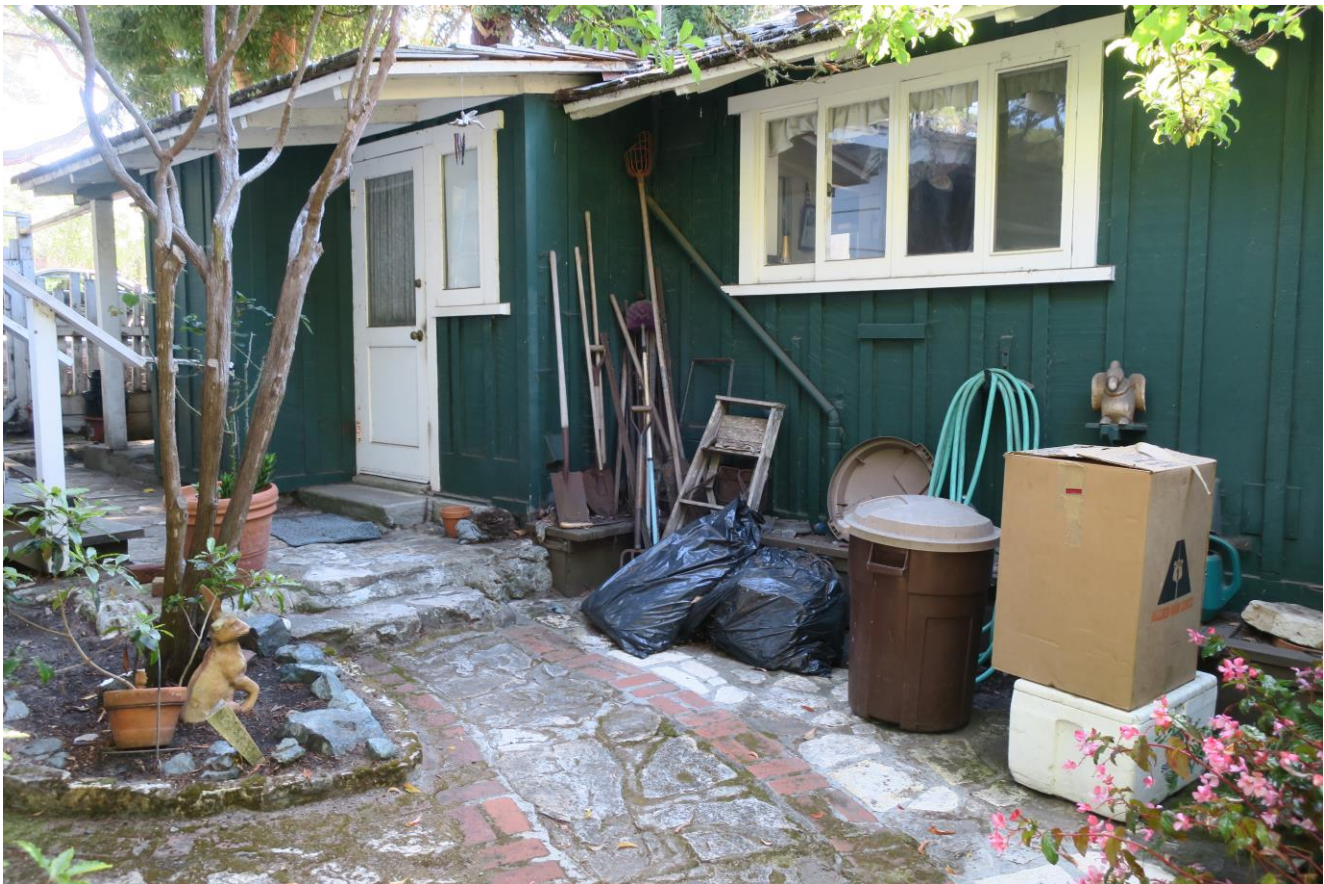
North side elevation, looking southeast.
