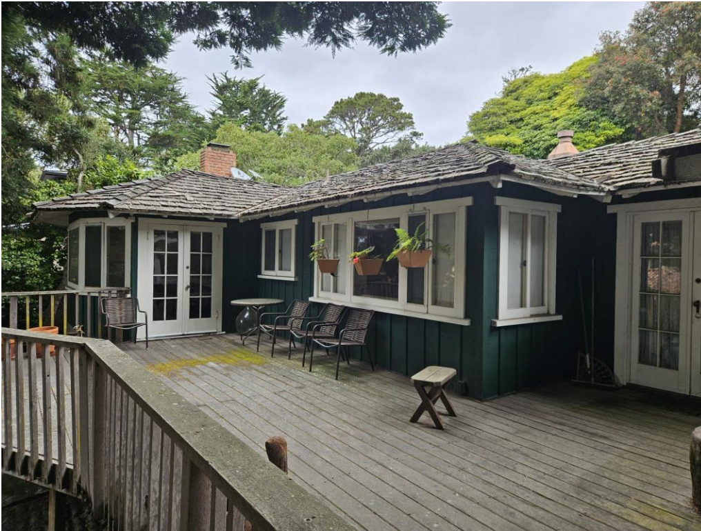
Figure 8: View of rear elevation and deck looking northeast.
