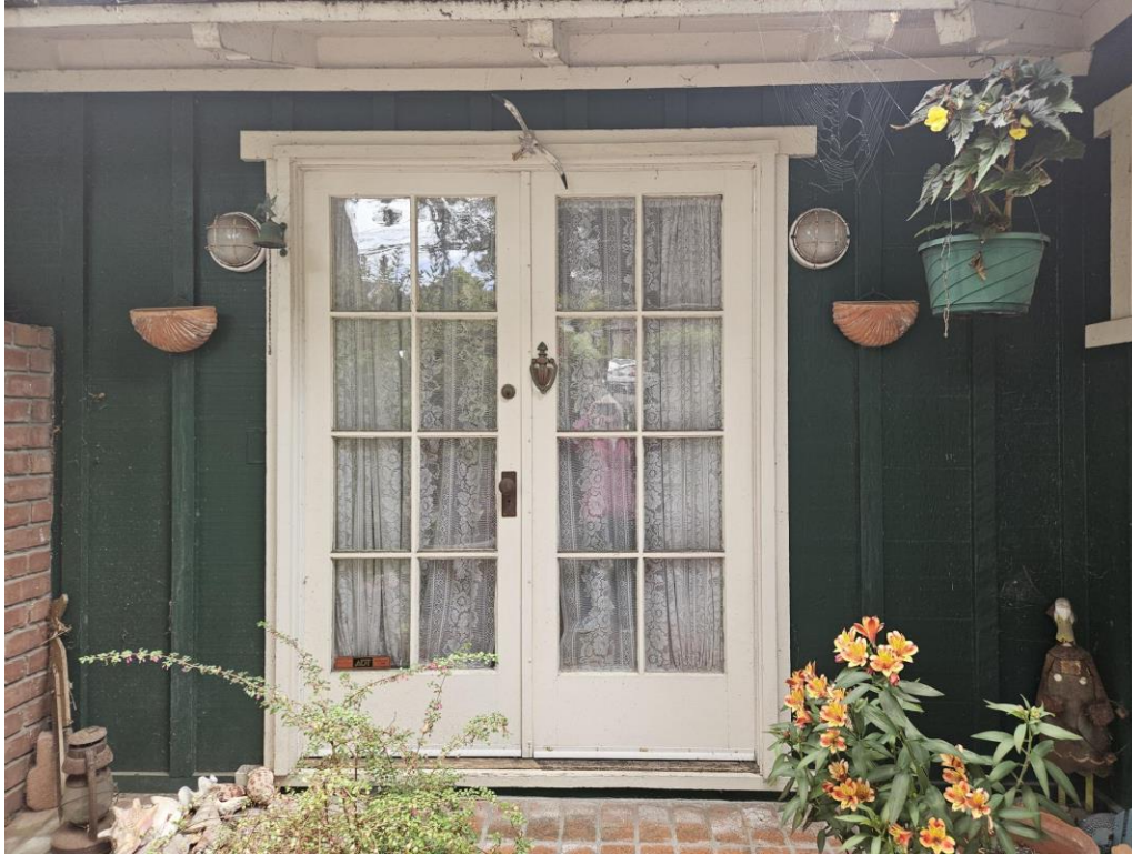
Figure 3: View of front French door with extended lintel and notched rafters.
