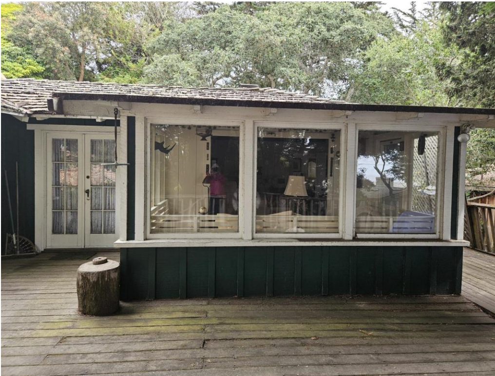
Figure 7: View of sunroom, rear (west) elevation.
