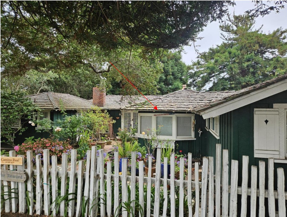
Figure 4: View of north wing bay, looking southwest.
