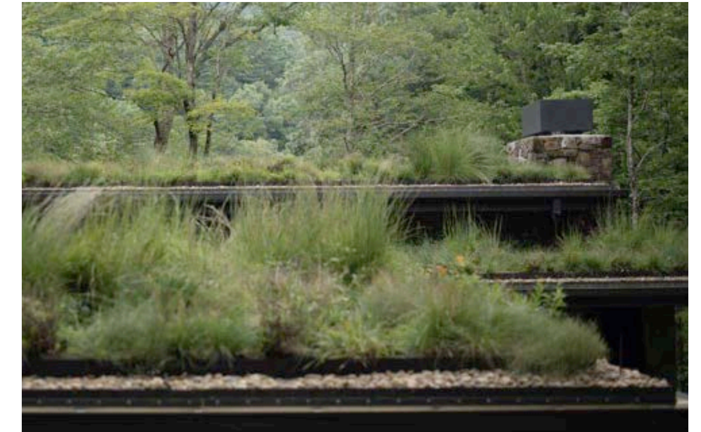
Green Roof Native, Drought-Resistant Living Roof
