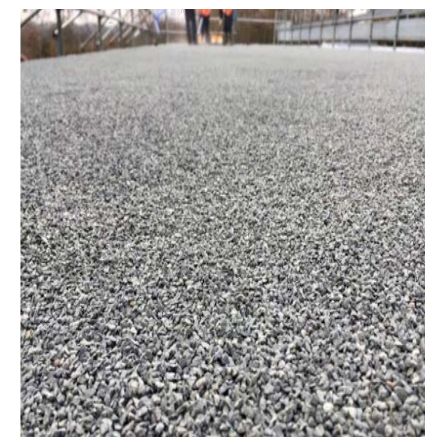
Flat Roof TPO w/ Gravel Ballast
