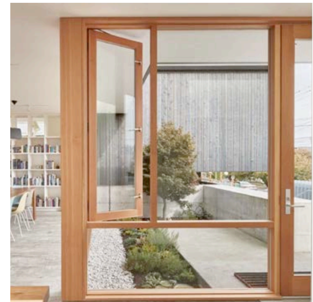
Exterior Doors + Windows Clear Finish, Douglas Fir Wood
