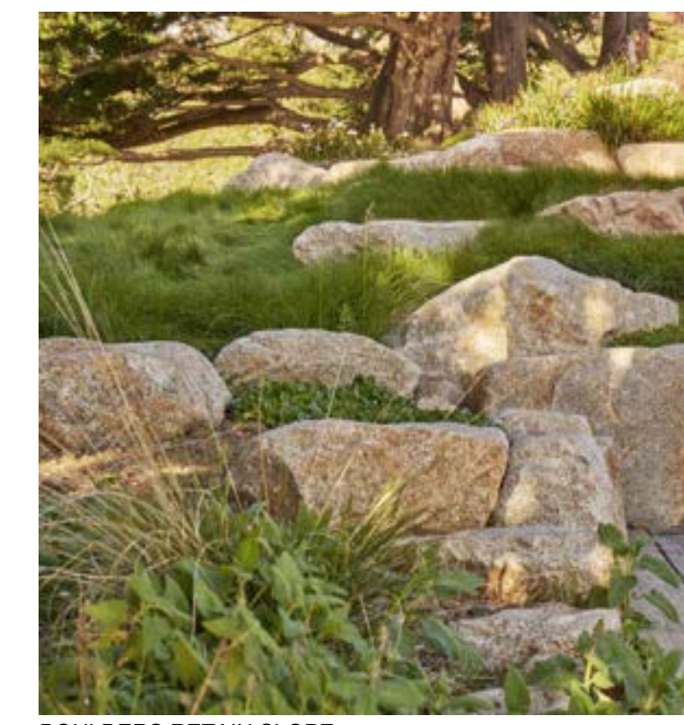
BOULDERS RETAIN SLOPE
