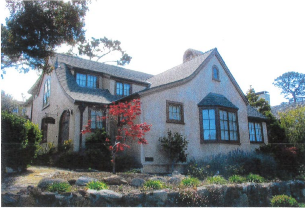
M.J. Murphy Tudor style office built 1926.
