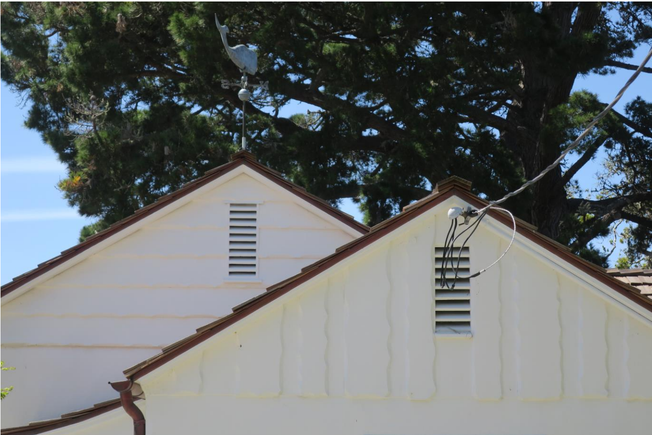
Figure 2: Wood and stucco detailing.
