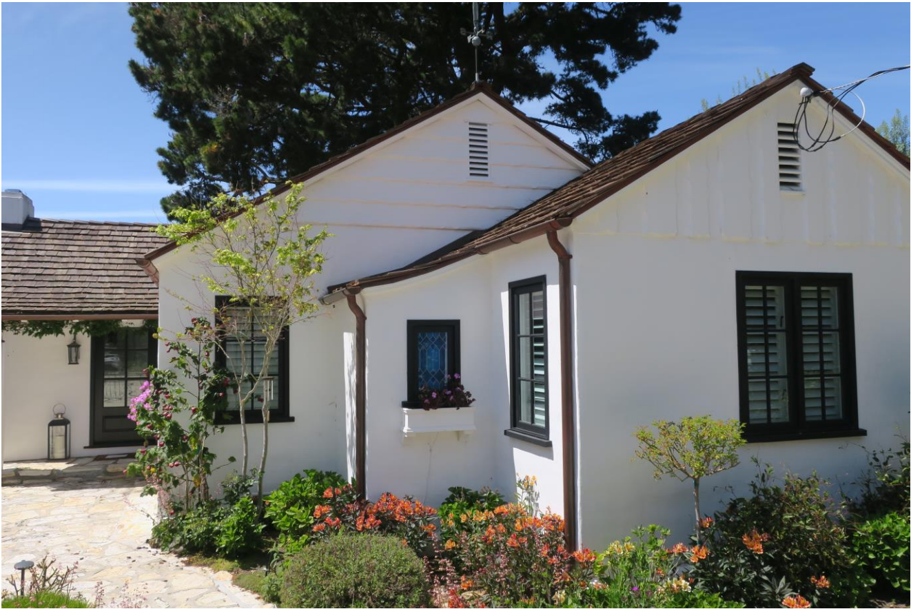
Façade, looking northwest.
