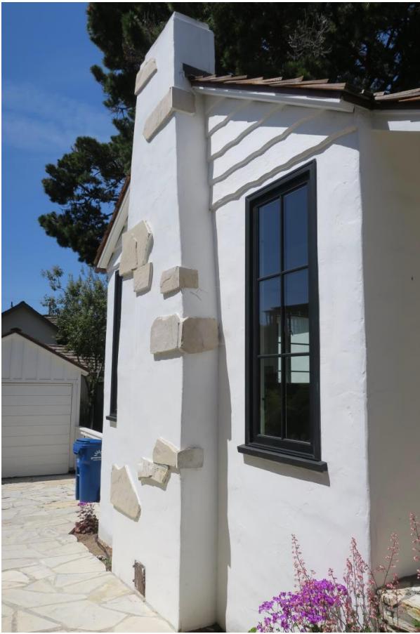
Original brick chimney on the south elevation covered over with stucco and stone, and replacement leaded glass window on the east elevation.
