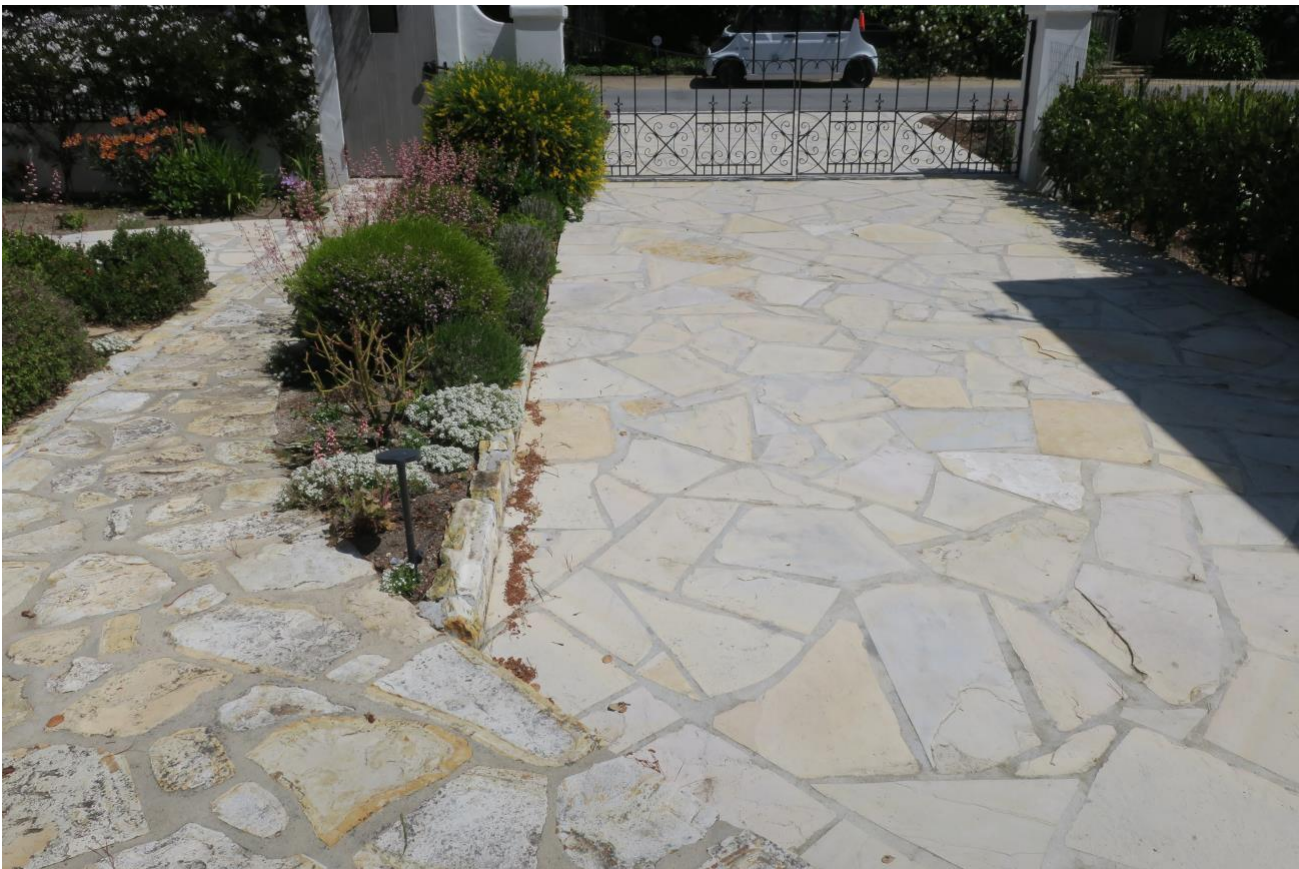
Original Carmel stone walkway (left) and recent stonework and driveway gate (right).
