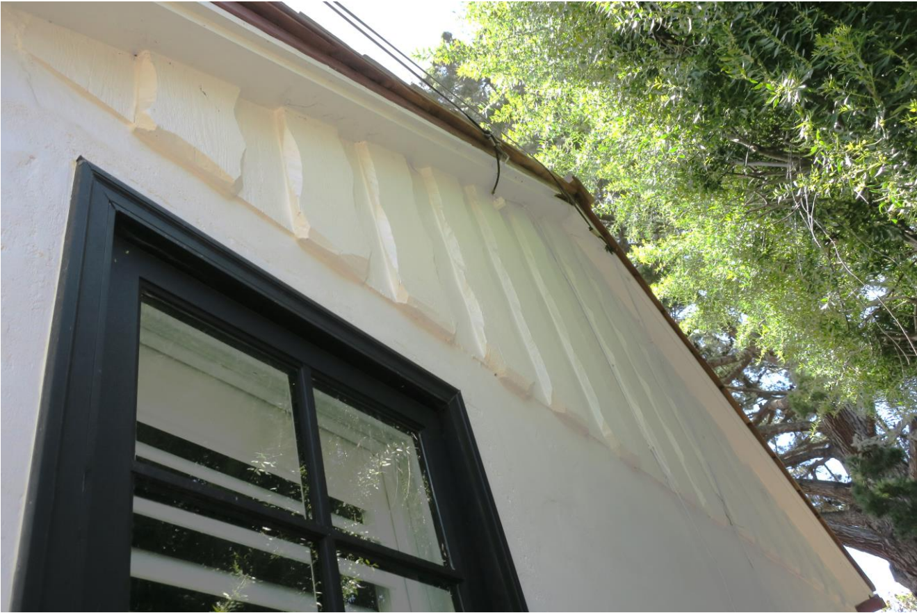
North elevation stucco and wood detailing in gable peak.
