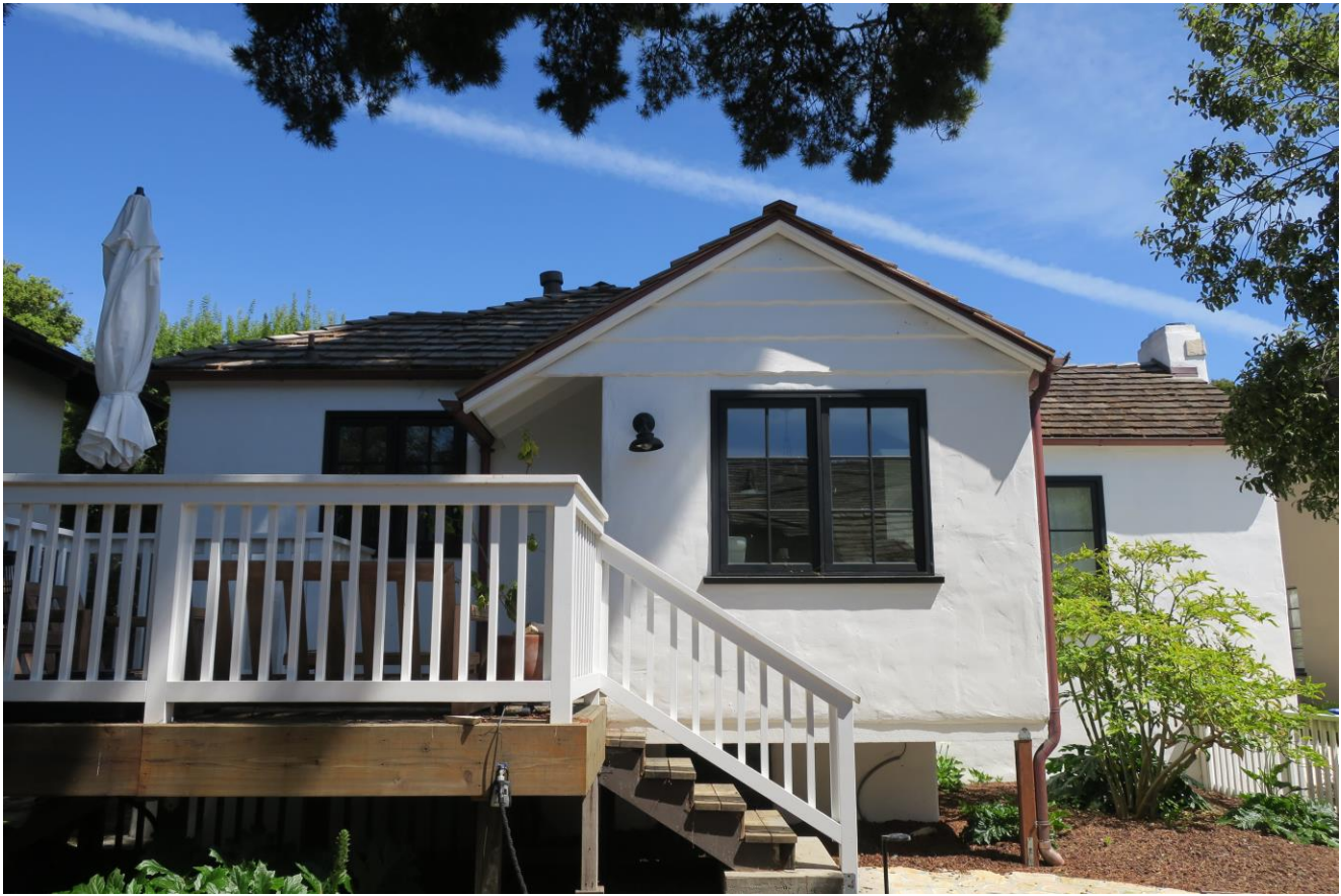
Rear (west) elevation, looking east.
