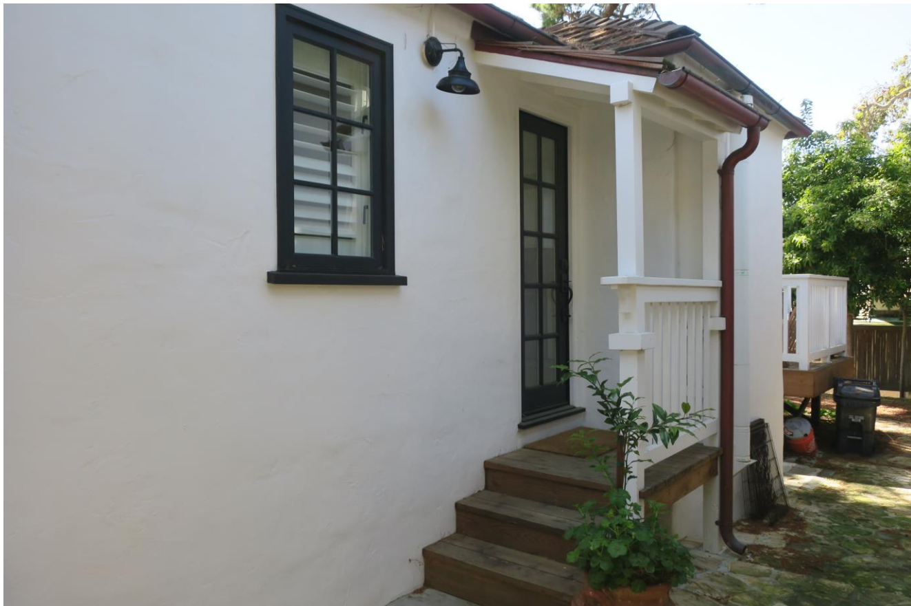
North elevation, looking southwest.
