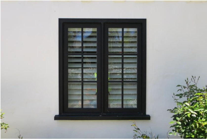
Aluminum-clad wood 6-lite replacement windows.
