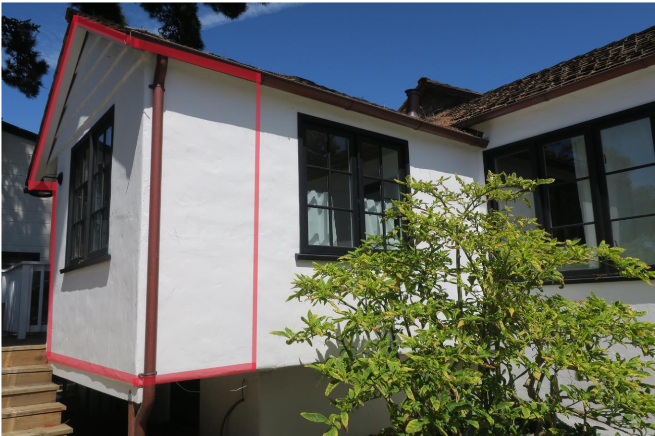
Rear (west) and south elevation, with the 1941 rear addition by Miles Bain outlined in red.
