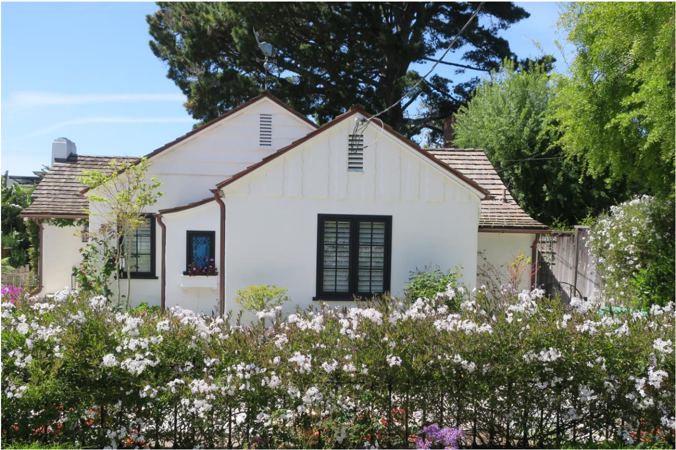
Figure 1: Façade, looking west.
