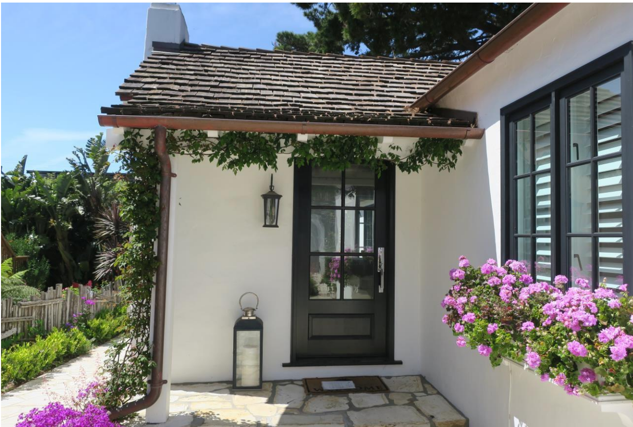
Replacement front door.
