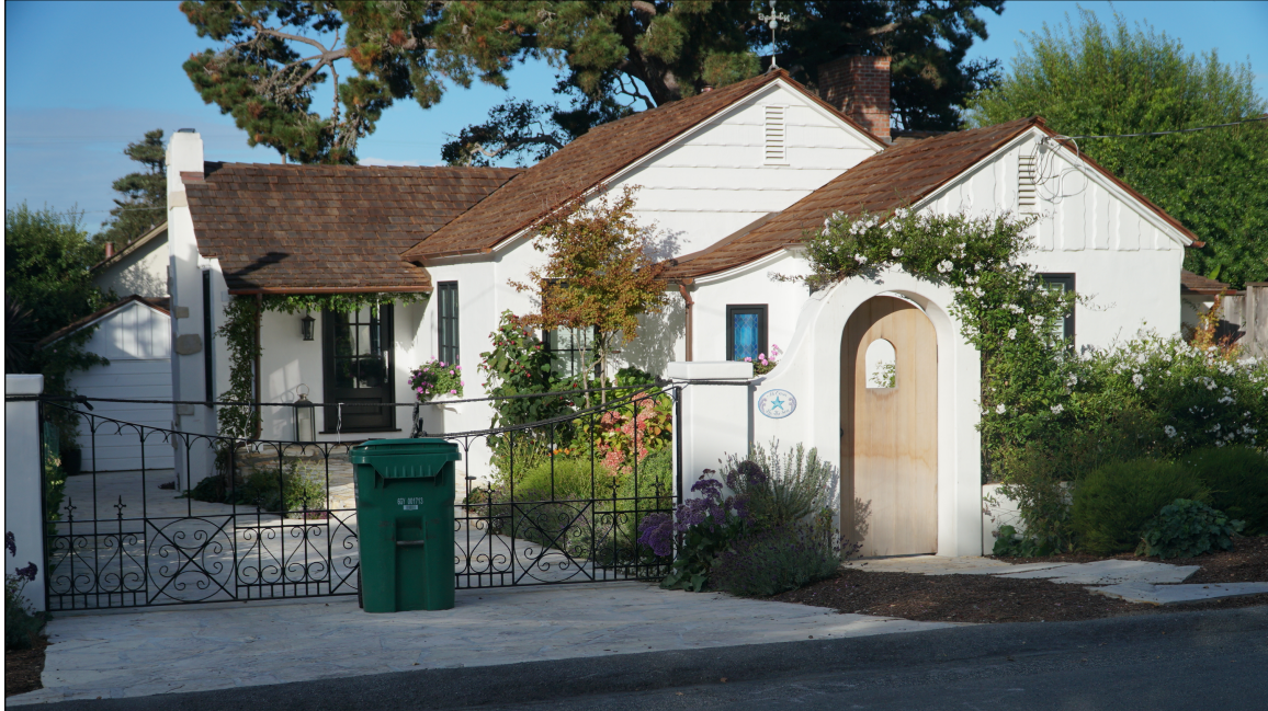
Figure 1. Looking northwest at south and east elevations of the house, 10 November 2023.
