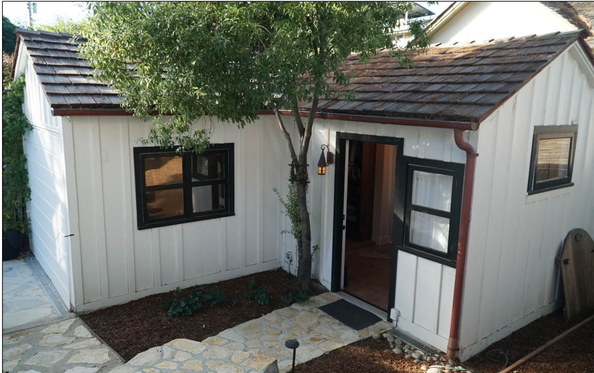
Figure 3. Looking southwest at east and north sides of former garage, now an office and a library, 10 November 2023.
