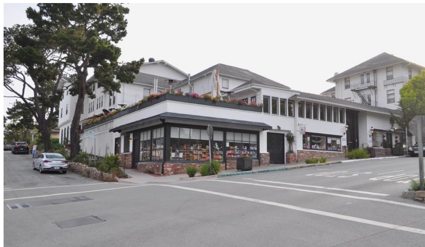
The Pine Inn. (Source: PAST Consultants, 2024)
