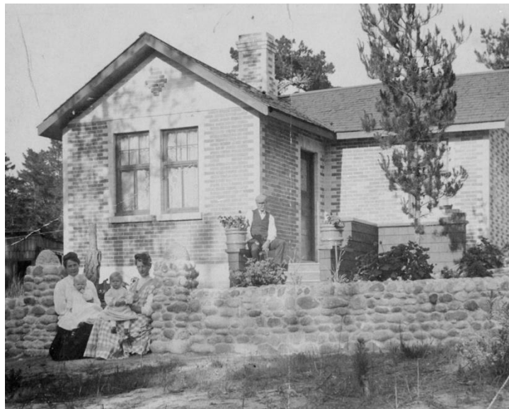
Circa-1900 image of the Benjamin Turner House, showing its vernacular-styled gable-on-wing massing, albeit with brick, rather than wood, wall cladding (Source: Harrison Memorial Library).
