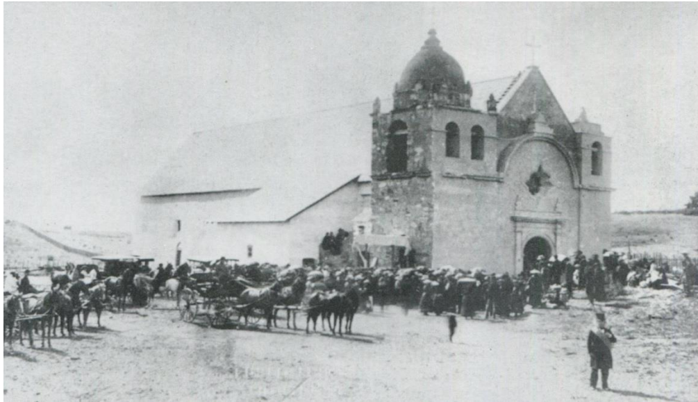
C.W.J. Johnson photograph of the August 28, 1884 rededication ceremony for the Carmel Mission, showing the replaced roof of improper pitch, compared to the original design (Source: Carmel: A History in Architecture ). 54
