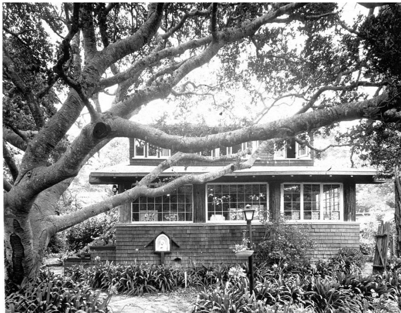
Arnold Genthe House on Camino Real. Note redwood trunks utilized as vertical structural supports (Source: Morley Baer archives, Monterey Area Architectural Resources Archive)
