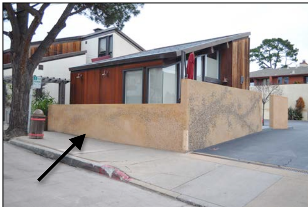
Figure 3. View of Community Room taken from Dolores Street, showing the wall cut down (arrow). The southern section retains its original height.
