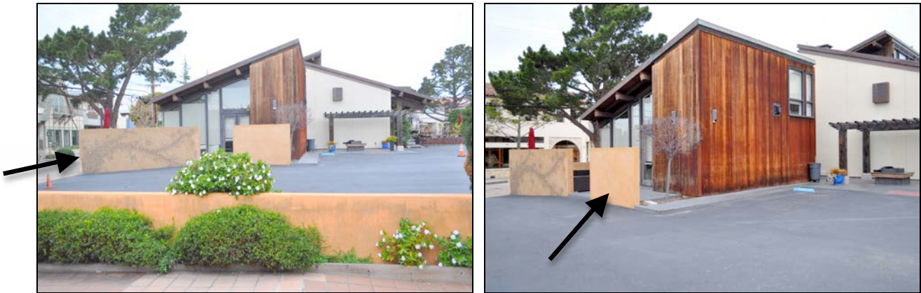
Figures 1 and 2. Left image looks north at the site. Constructed in 2014, the wall in the foreground is not a historic addition to the site. The original ornamented concrete wall is shown with an arrow. Right image details the Community Room looking northwest, with the 2014 stucco wall shown.
