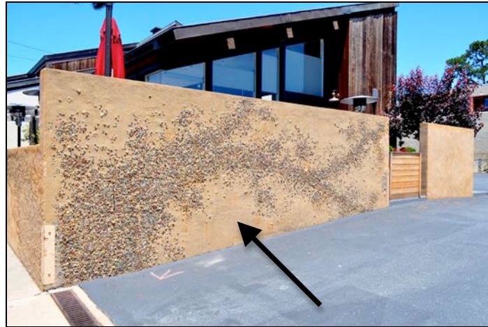
Figure 7. Remaining intact section of the ornamented concrete wall.
