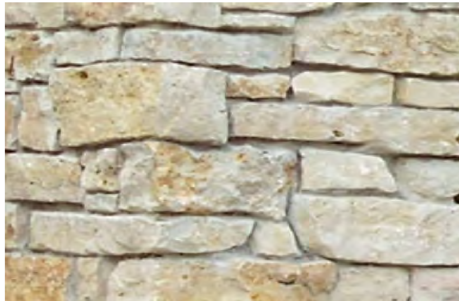
THIN VENEER STONE CLADDING
